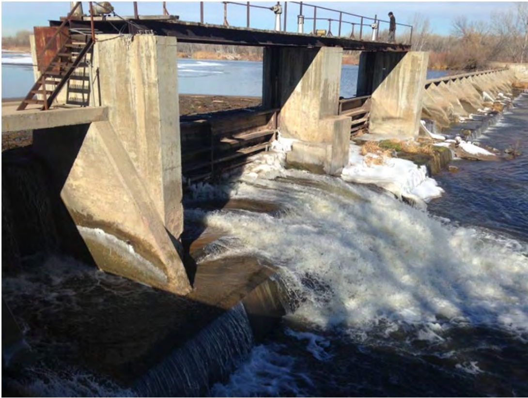
Fig. 9: Vertical gates, south section (looking upstream).
