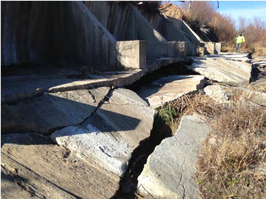
Fig. 4: Collapse of downstream floor slab, diagonal section.
