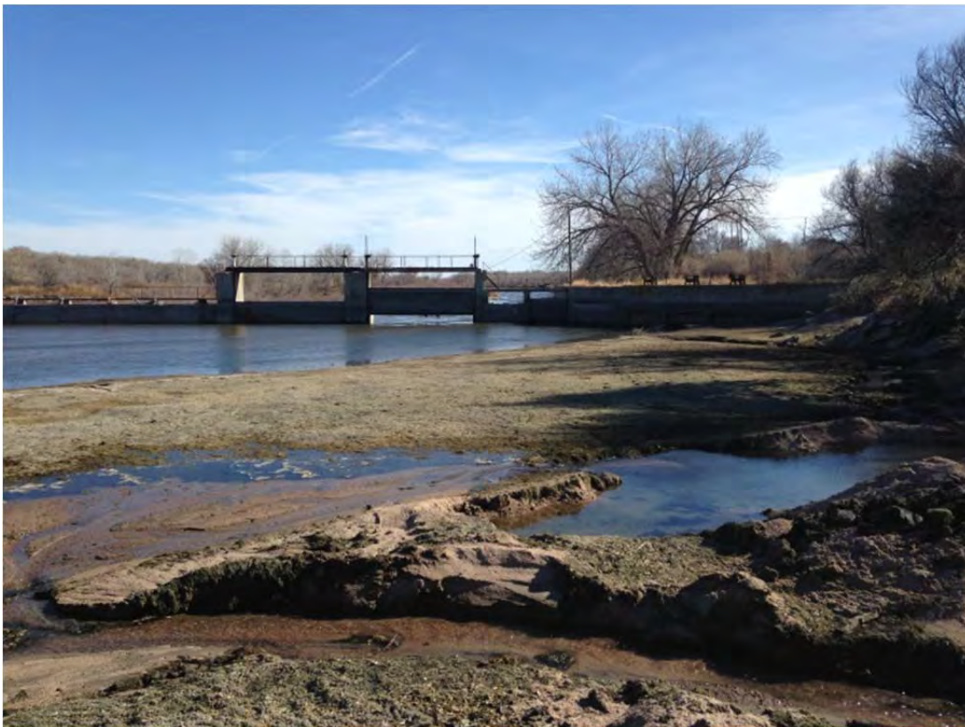
Fig. 8: Vertical gates and radial gate, south section (looking downstream).
