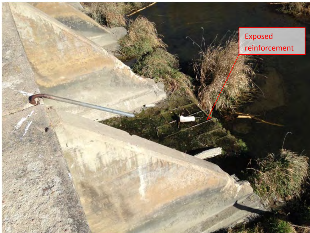
Fig. 6: Exposure of rebar on downstream floor slab, south section.
