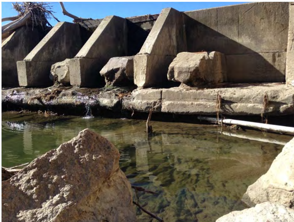
Fig. 2: Flash board bays, north section (looking upstream).
