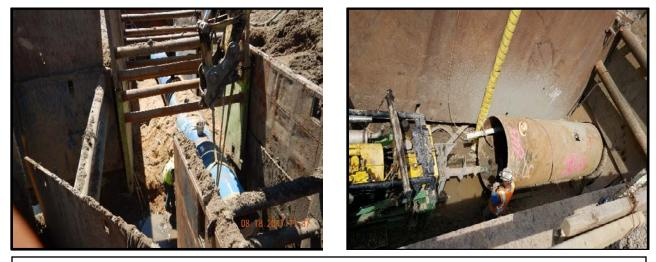
Photos show installation and welding of the new pipeline near Rueter-Hess Reservoir. The pipeline extends from Chambers Road and E-470 to the Parker Water Treatment Plant south of Rueter-Hess Reservoir.
