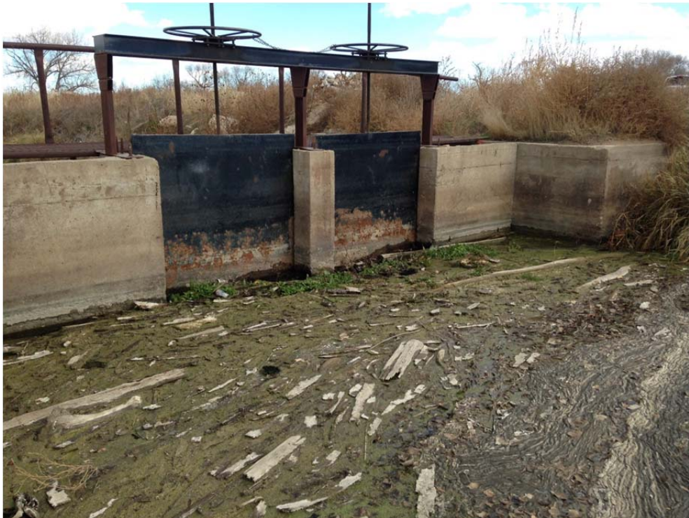
Photo 6: Ditch Intake Structure.
