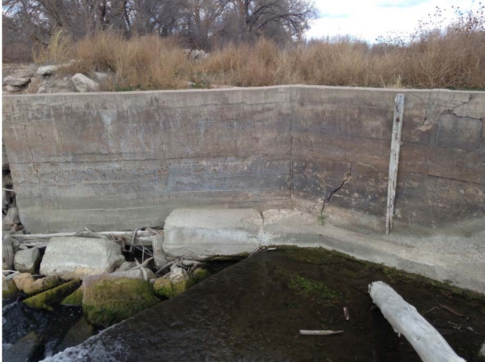
Photo 5: Fatigue Cracking on South Abutment Wall. Note exposed timber piling at lower left.
