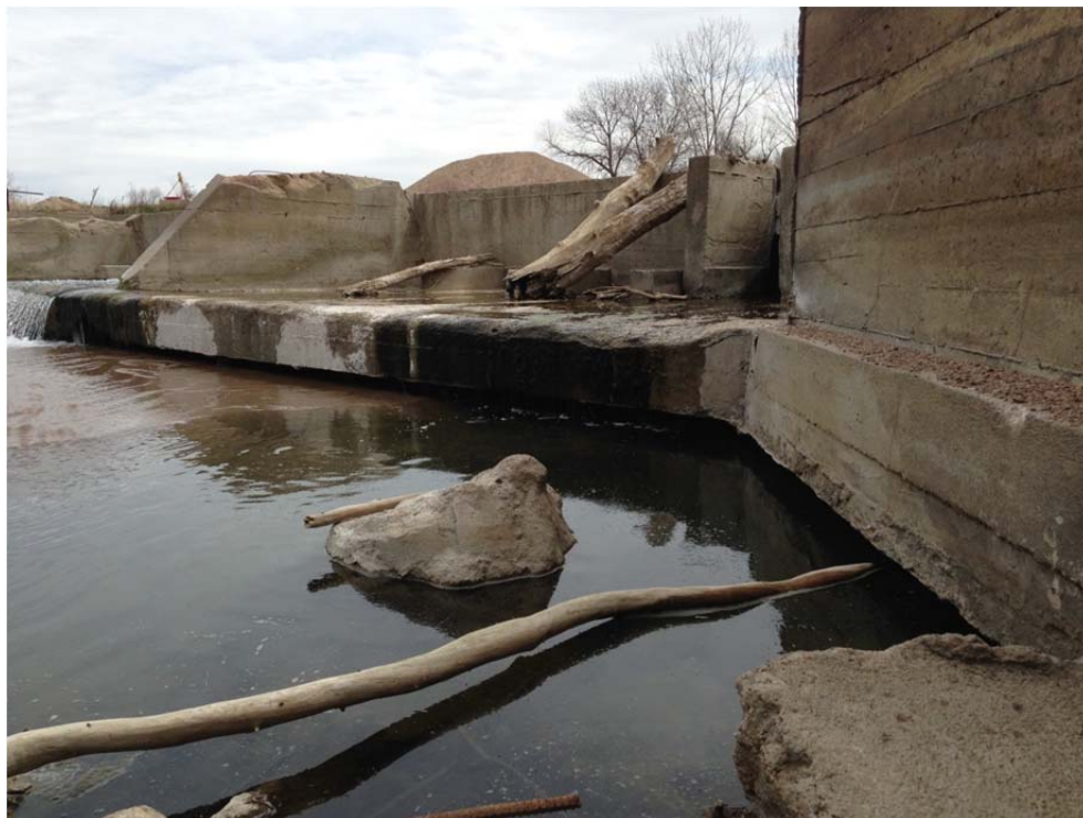
Photo 3: Void Under Structure Floor Caused by Scour (view looking upstream).
