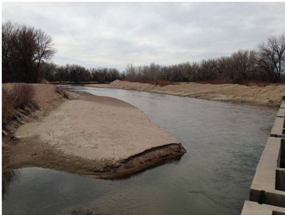
Photo 4: Sand Deposit and Dredging Windrow Upstream of Dam (sand chutes are fully open).
