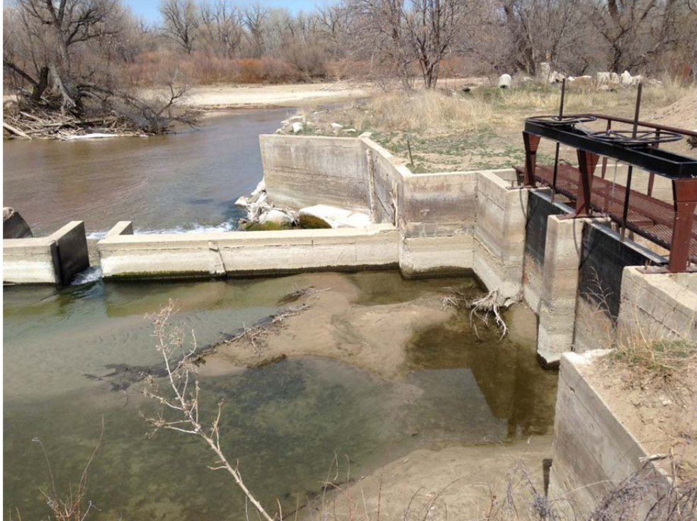
Photo 1: South Abutment and Ditch Intake (looking downstream). Note sediment deposition in front of headgate.
