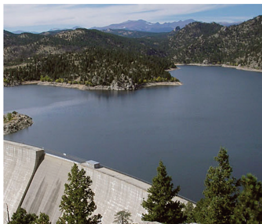
Gross Reservoir, located in the foothills southwest of Boulder, Colorado
