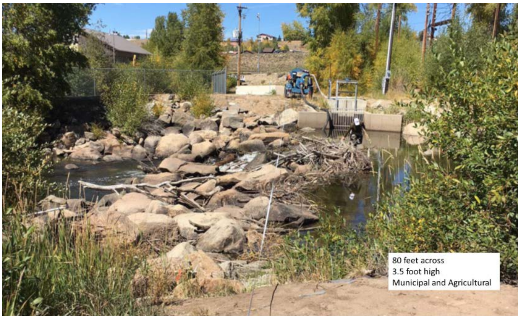
Figure 2. Granby Diversion Dam is a fish and boating barrier.
