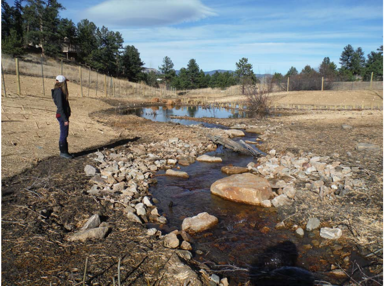
After Project Implementation. Bottom to top = Upstream to Downstream. Temporary Wood Grade Structure (TWGS) can be seen on the downstream end of the picture.
