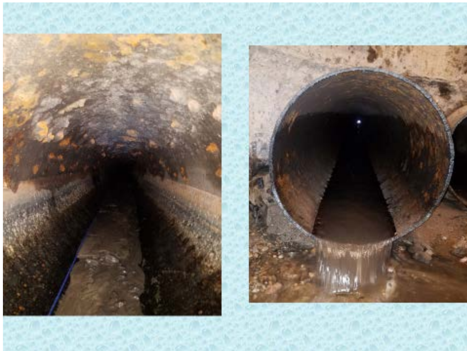
Jetting the Conduit pipes before Lining
