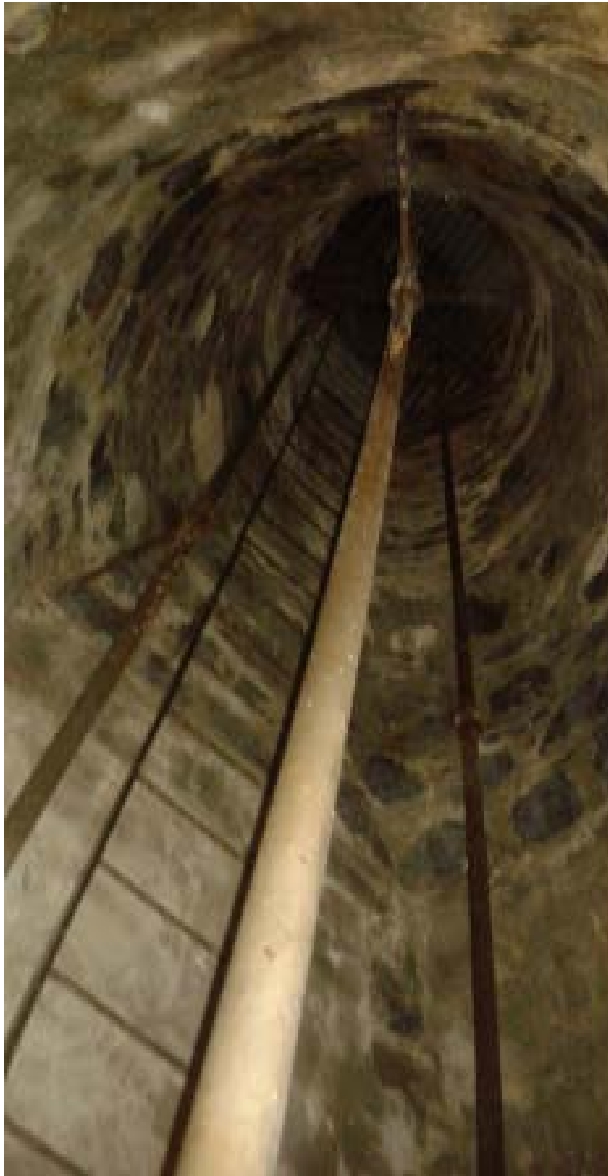
Shaft from Gate Valves to top of Dam, Valve Operators
