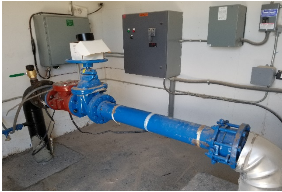
Well No. 12 control building new pump and SCADA system.
