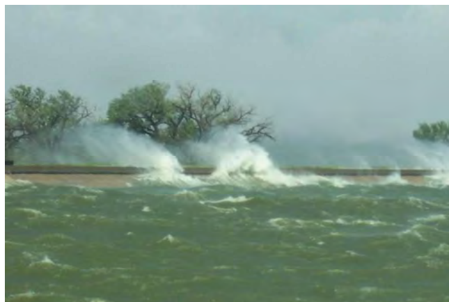
Figure 1-1: Embankment Overtopping During Wind Event
