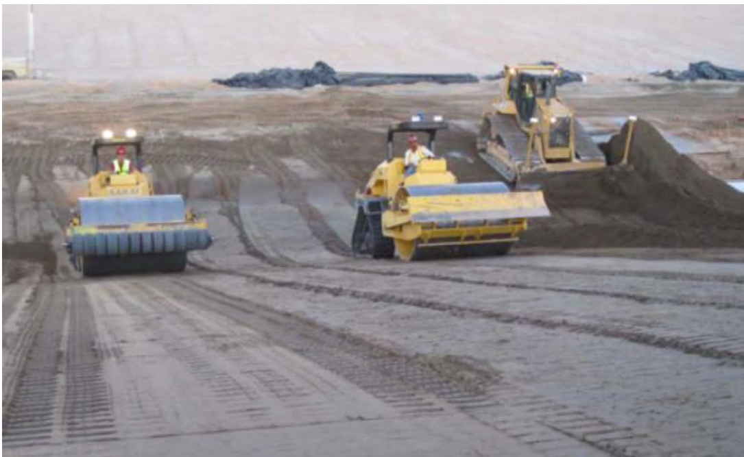
Figure 3-8: Plating Method of Soil-Cement
