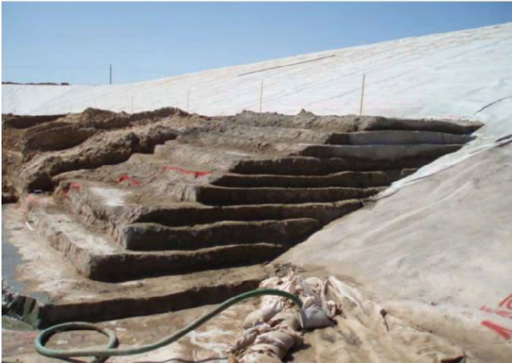
Figure 3-7: Stair-Stepped Soil Cement
