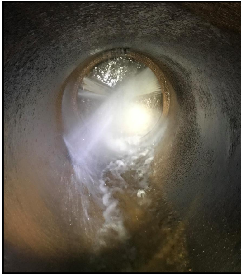
Photo 6. Downstream view of West Gate Valve Leakage
