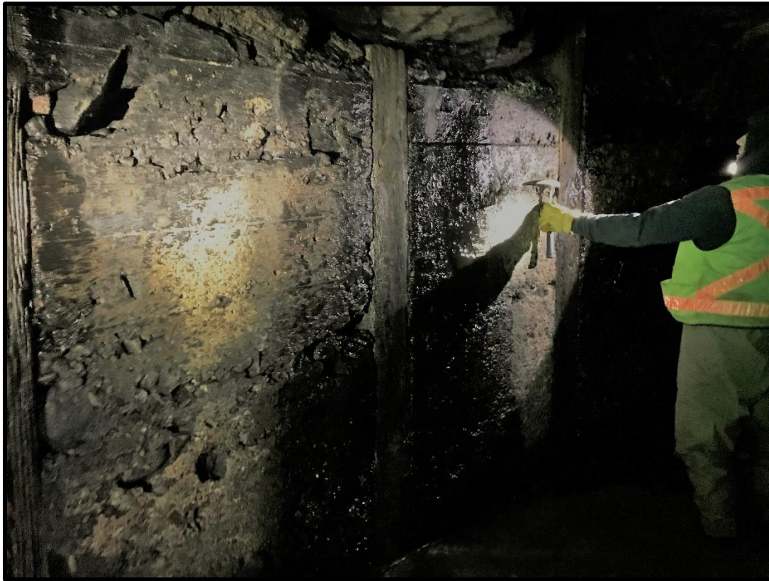
Photo 1. Concrete and timber bulkhead near abandoned access adit.
