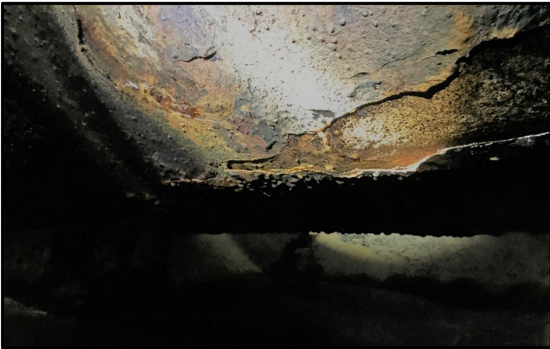
Photo 4. Underside of the 48-inch diameter welded steel pipe showing corrosion and iron oxide layers.
