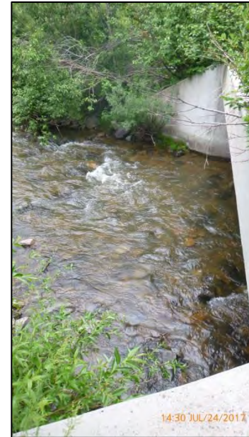
Photo 28. Road crossing at Pass Creek.
