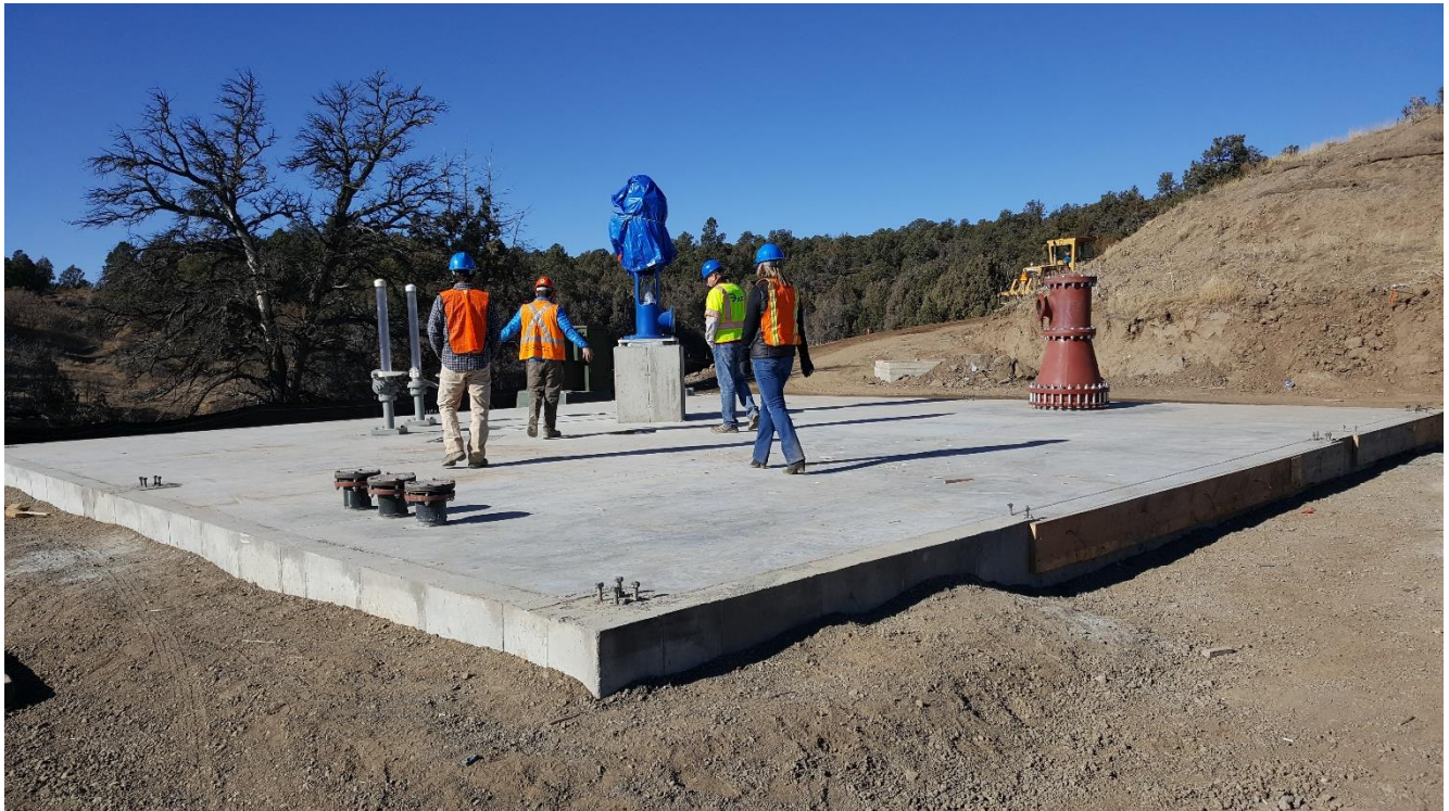
Figure 2: The intake Structure is below grade of concrete slab, which now has pumps mounted for Raw Water Pipeline Project
