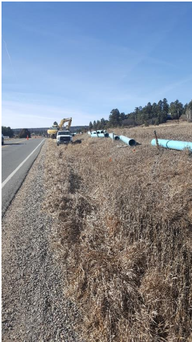
Figure 5: Installation of 16" LPWWA-CWCB funded pipeline segment
