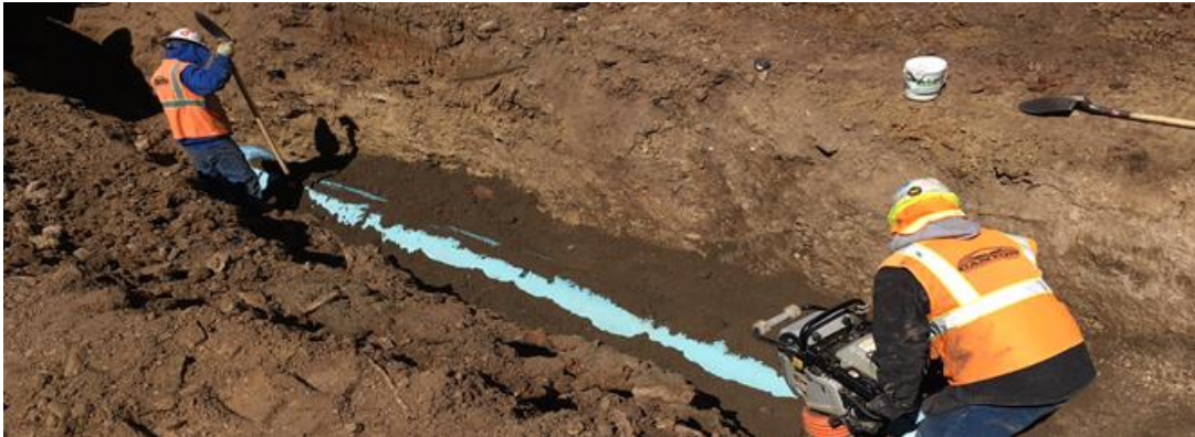
Figure 4: Installation of the 16" pipeline
