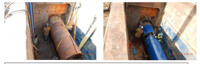
All photos show installation and welding of the new 42-inch Ridgegate pipeline near Rueter-Hess Reservoir. The pipline extends from Chambers Road and E-470 to the Parker Water Treatment Plant south of Rueter-Hess Reservoir.
