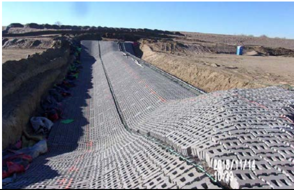
ACB mat installation at Station 17+00 completed. Mat joints still require concrete fill.
