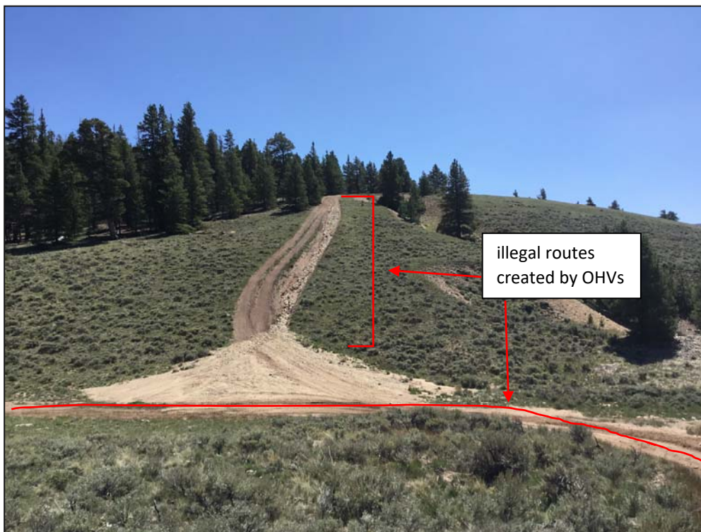
Image 1. Photo of an illegal route on hillside. The hillside has a long path of erosion and a large sediment plume at the bottom of the route. We would use heavy equipment to break up the compacted route, re-seed and install water bars. We would also close this route from the top and bottom with large boulders and close signs. Just downhill of this photo is a headwater stream that feeds into an important wetland called a Fen.
