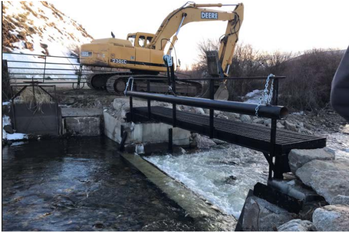
Metal strapping on blocks (below)
