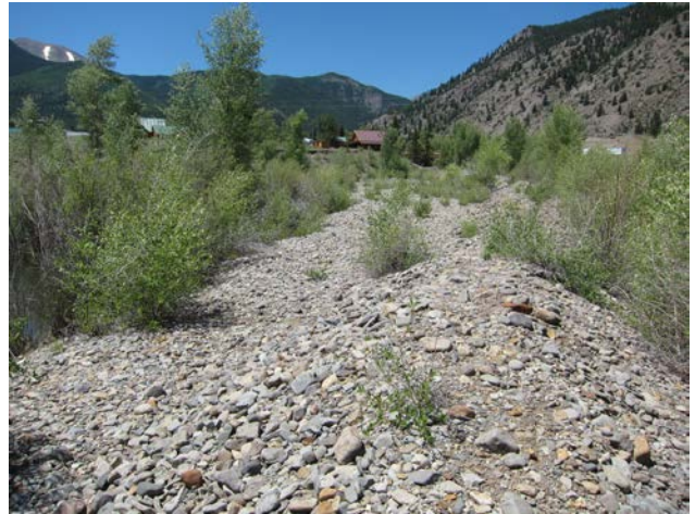
Figure 3. Pre-construction photos of area pre-flood (2009) and post-flood (2014 and 2016). In 2015-16, many of the trees on the left bank were lost. The first photo shows the gravel berm on the west side. This one was mostly washed out with the high flows in 2014-16 (third and fourth photos). The second photo shows the old gravel berm on the east side of the river, which was removed.
