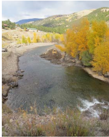
Figure 5. Reshaping of the flood plain and structure installation below the 8 ½ Street Bridge (fall 2016). The second to last photo is looking back toward the bridge and shows where a large area of berm was removed. Last photo is the area after one year of high flow (fall 2017).
