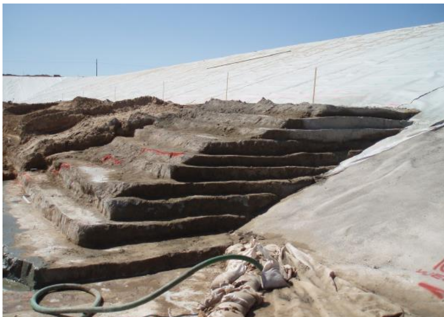
Figure 2: Stairstep Soil-Cement Placement
