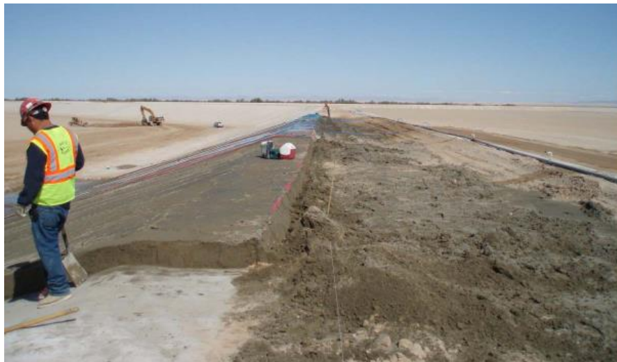
Figure 1: Plating Soil-Cement Placement
