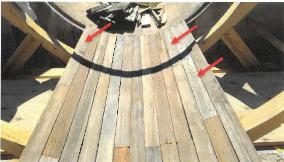
Figure 6. Short staves installed at the southeast end of the Flume. These staves will need to be removed and replaced by longer staves, spanning at least across two bends.
