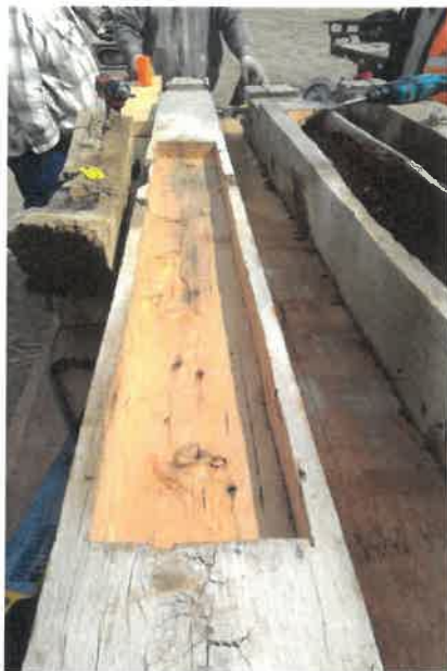
Figure 8. Dutchman repair at sill. Deteriorated wood removed to sound material. Pocket to be filled with new lumber.
