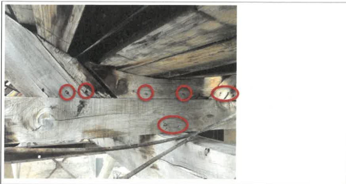
Figure 9. Typical toe-nail connections at Flume bent.
