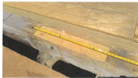
Figure 6. View of repair work at sills.
