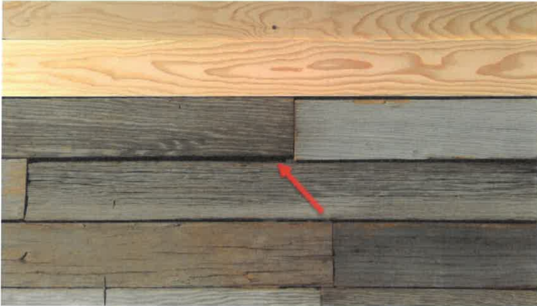
Figure 5. Misaligned staves, leaving large gaps in the half-pipe.
