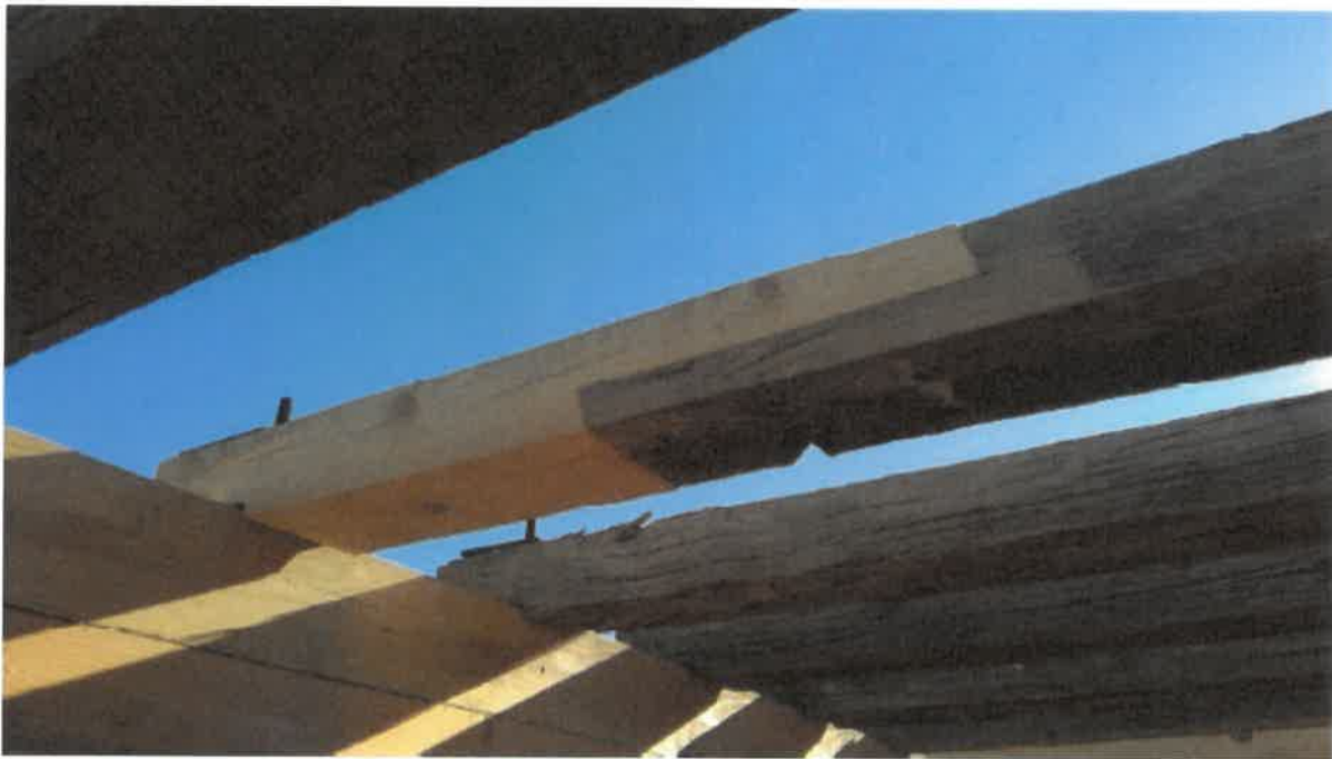
Figure 6. Closeup view of splice repair at spreader's end.
