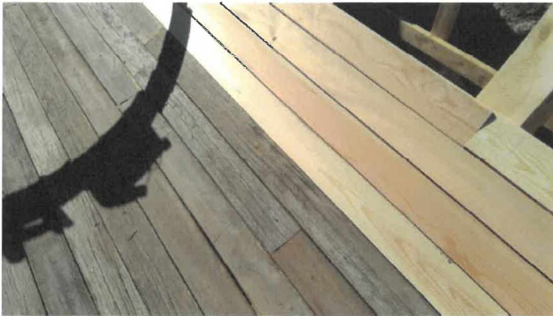
Figure 3. Grain structure and profile of new staves closely matches the original material.
