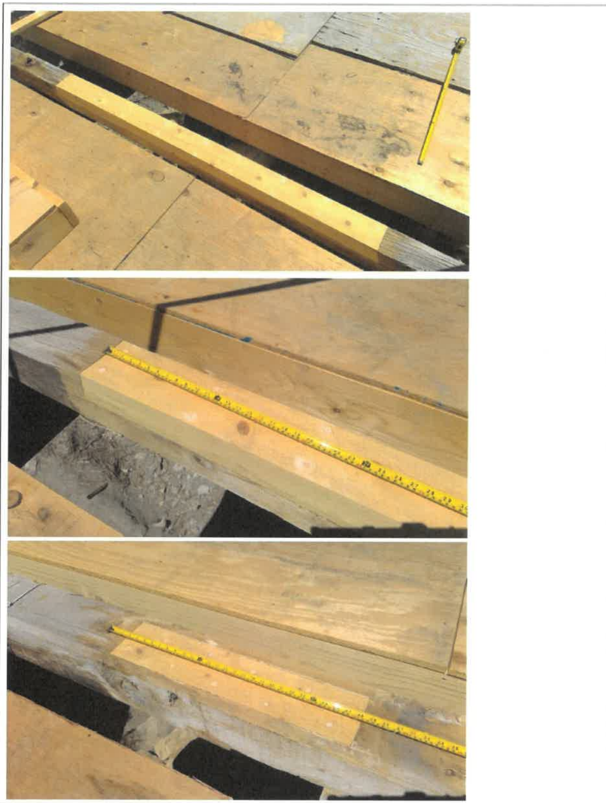
Figure 6. View of repair work at sills.
