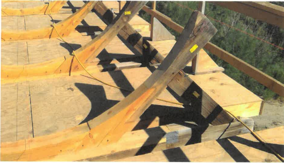
Figure 2. View of splice repair at segments.
