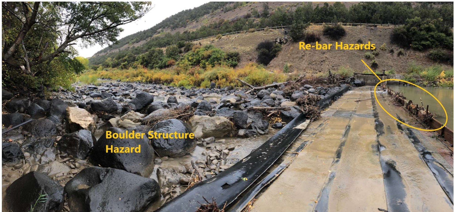
North Fork Farmers Ditch Diversion: Boulder Structure and Re-bar Hazards
