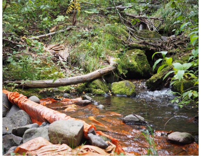
Tarp being used to divert flow to the Himes Ditch.
