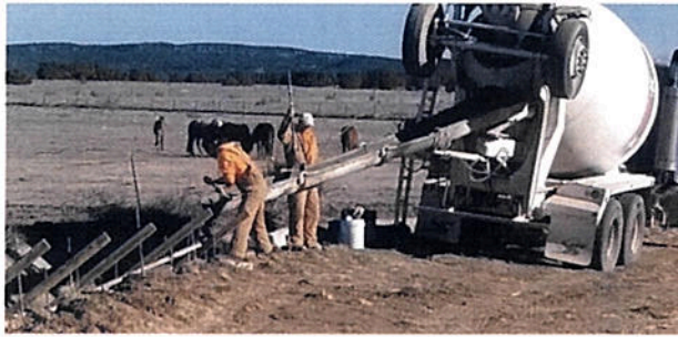
New concrete canal sections being formed and poured (January 8, 2019).
