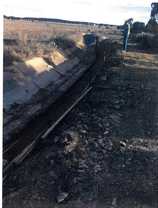
Damaged concrete canal lining sections removed. New sections being formed. Completed sections covered with freeze protection tarps in the background (January 8, 2019).
