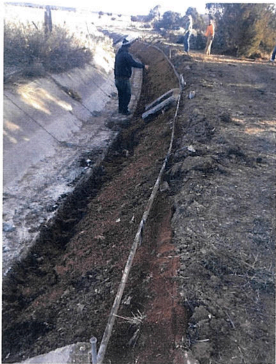
Damaged concrete canal lining sections removed. New sections being formed. Completed sections covered with freeze protection tarps in the background (January 8, 2019).
