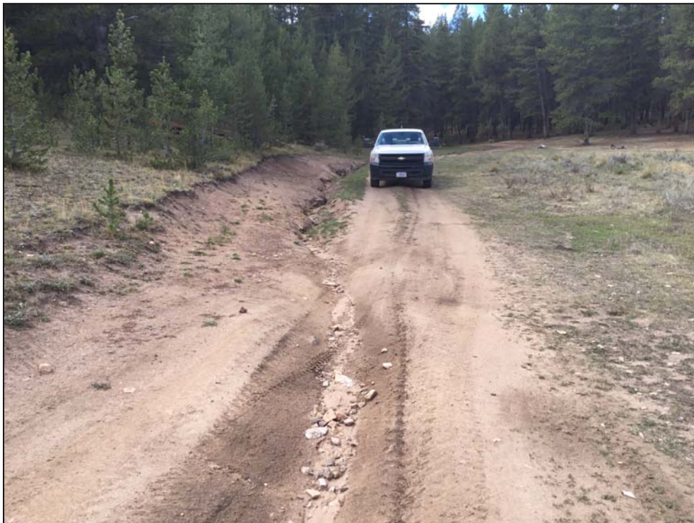
Image 8. Just another road in the project area that is to be closed. Note the erosion coming down the road. We use heavy equipment to close and build in water bars.
