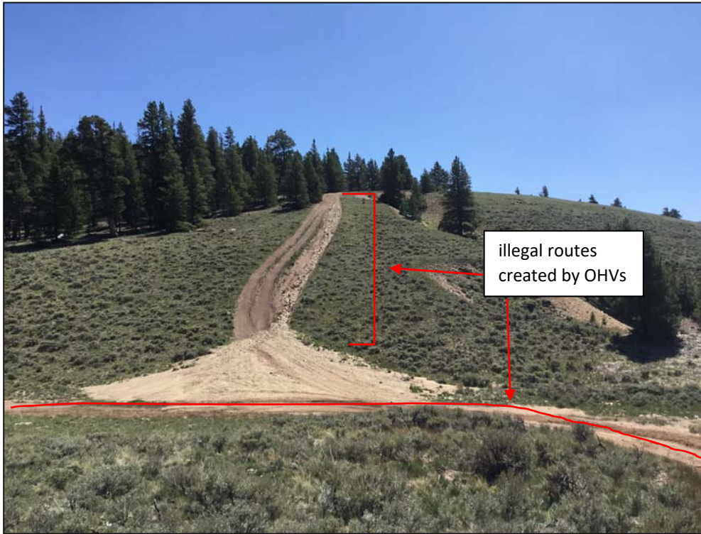
Image 1. Photo of an illegal route on hillside. The hillside has a long path of erosion and a large sediment plume at the bottom of the route. We would use heavy equipment to break up the compacted route, re-seed and install water bars. We would also close this route from the top and bottom with large boulders and close signs. Just downhill of this photo is a headwater stream that feeds into an important wetland called a Fen.
