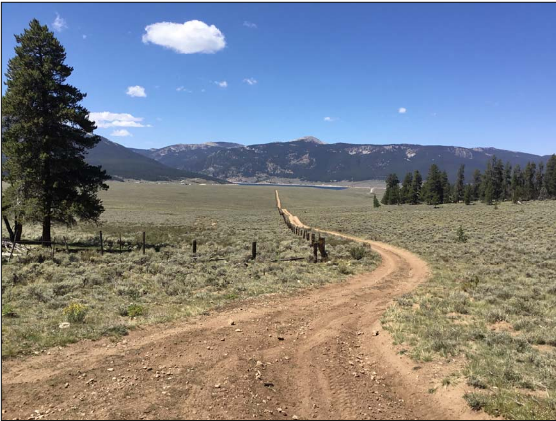
Image 7. While it might be hard to believe, this entire route in the photo is a user created, illegal route. We would use heavy equipment to rip the road and reseed. We would also use large boulder to close both ends of the routes and sign with closer signs.
