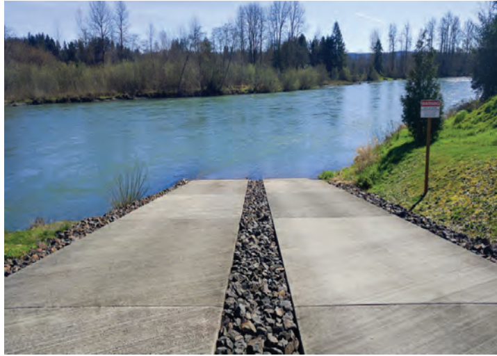
Concrete Boat Ramp - 30' Wide
