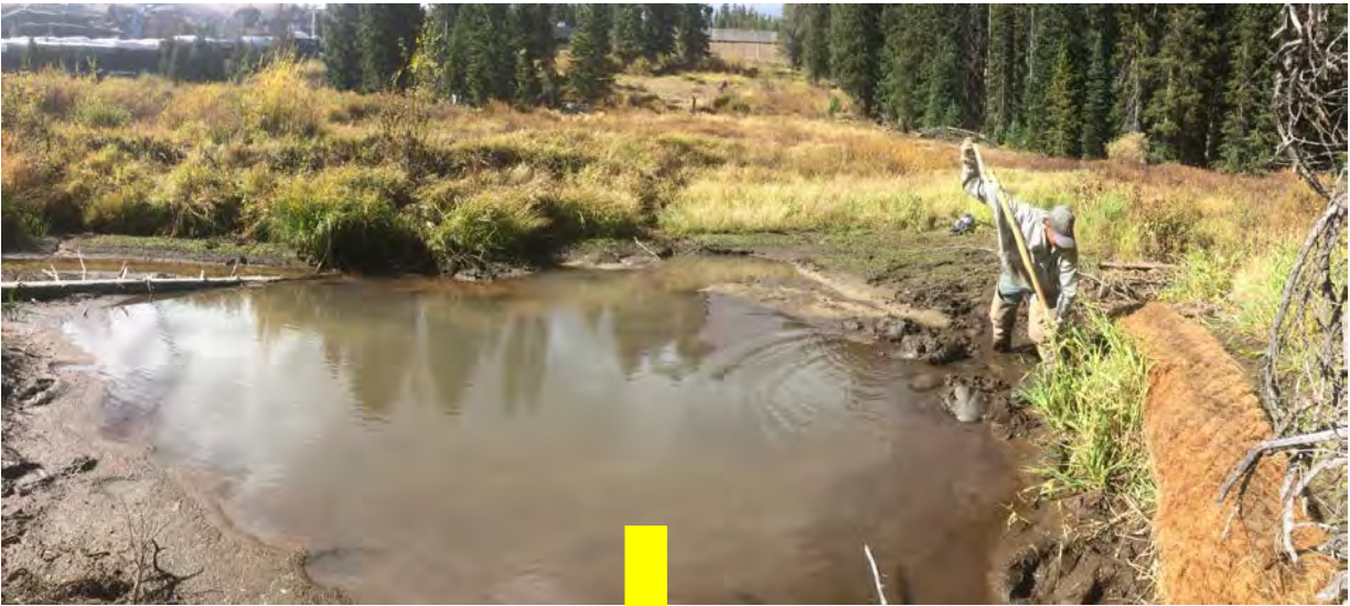
↑Repairing breached beaver dams with coir logs and sod.
