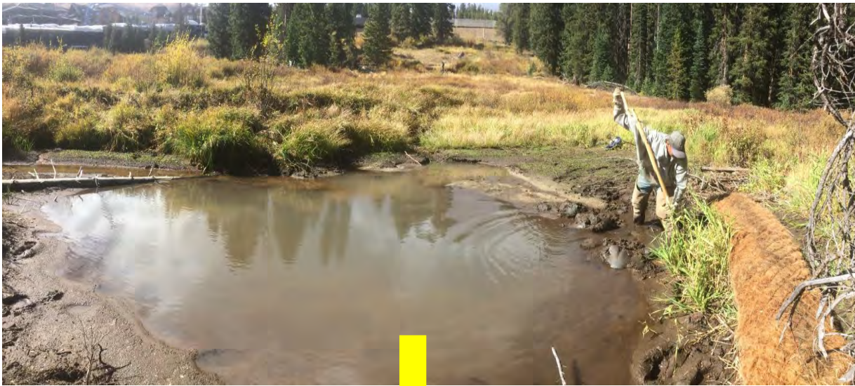
↑ Repairing breached beaver dams with coir logs and sod. ↓ Before and after.
