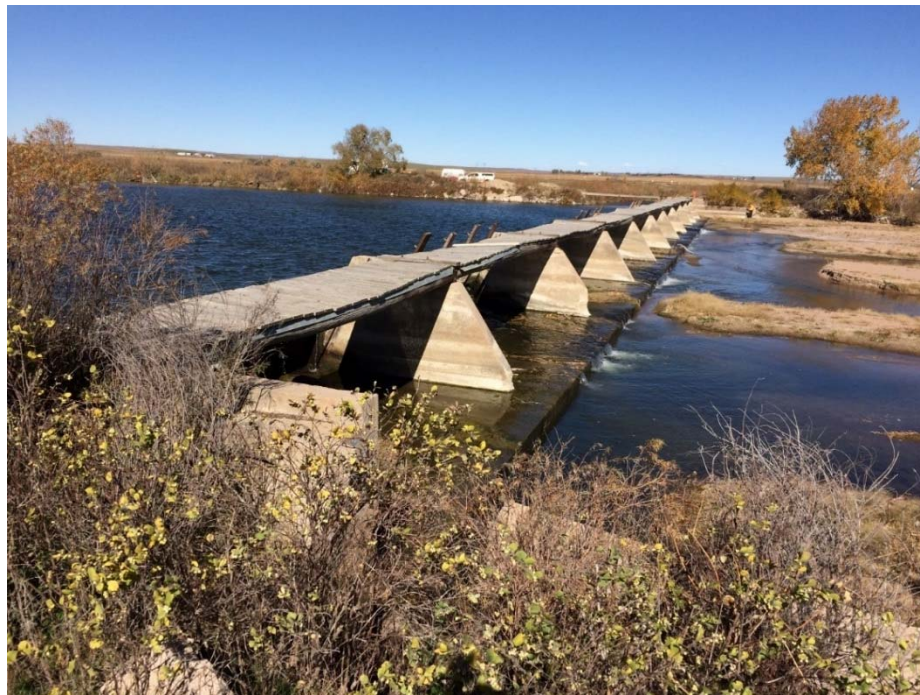
PHOTO 2 – DOWNSTREAM VIEW OF 320-FOOT DIVERSION DAM
