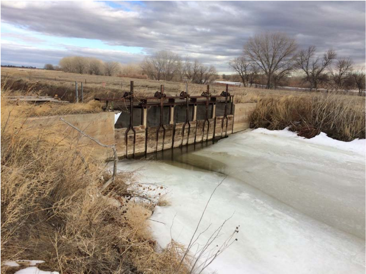
PHOTO 6 DITCH GATE STRUCTURE DURING WINTER OPERATIONS
