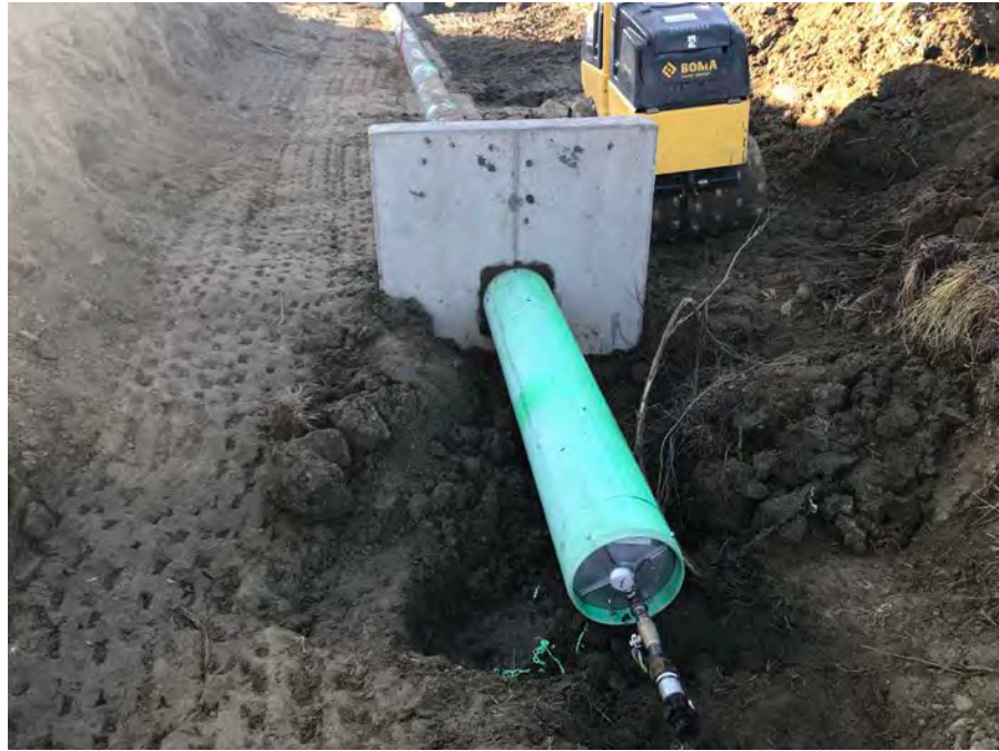
37. View of the pressure test of the outlet conduit completed on Oct. 25, 2018.
