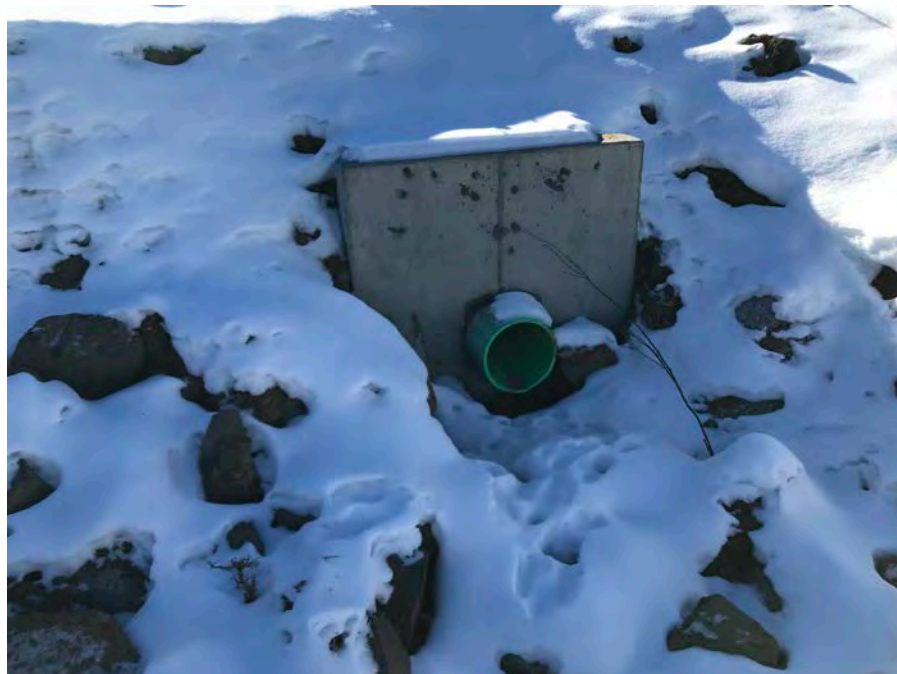
58. View of the new mid-level outlet headwall and discharge pipe.
