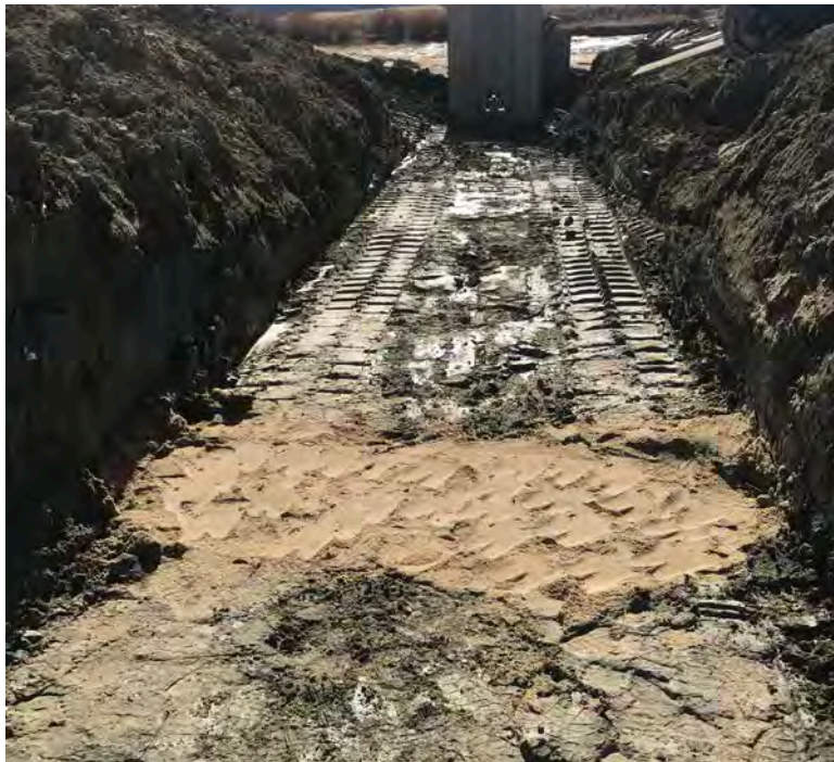
26. View of installed filter diaphragm below the outlet conduit pipe and cradle.
