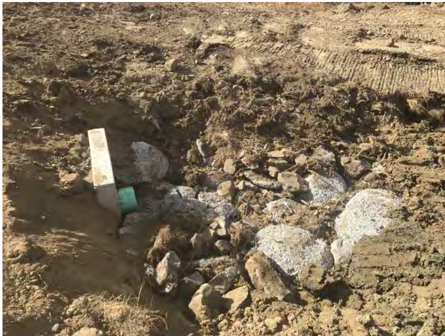
50. View of completed mid-level discharge outlet, Note riprap installed in the channel.
