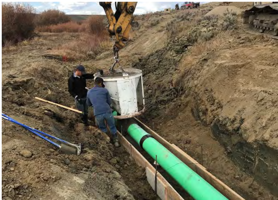
32. View of the concrete placement for the outlet conduit pipe cradle.
