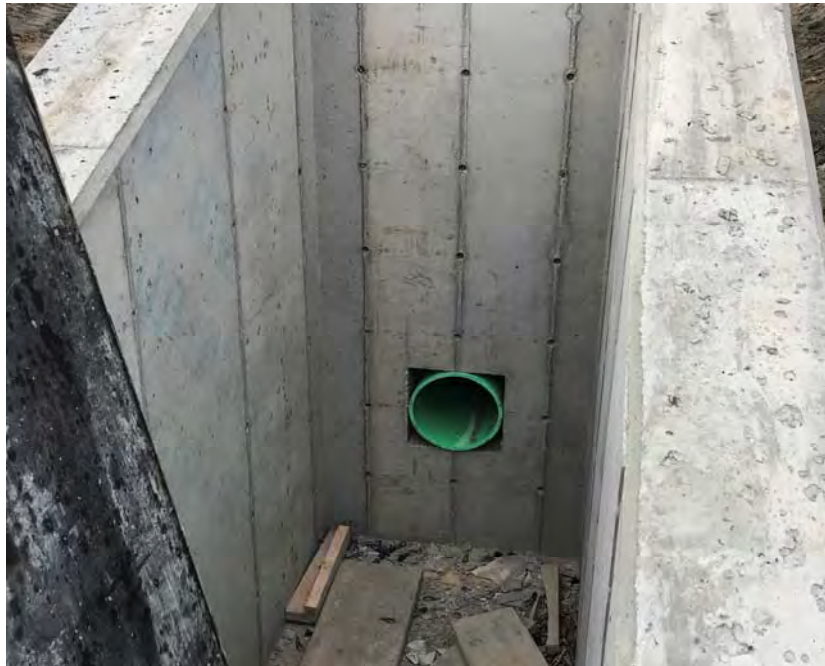
28. View of the new outlet pipe installed through the intake structure.
