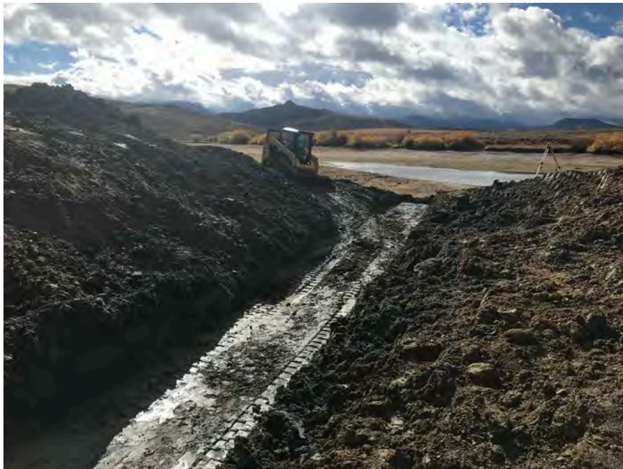
6. View looking upstream of the exposed foundation preparation for the mid-level intake structure.
