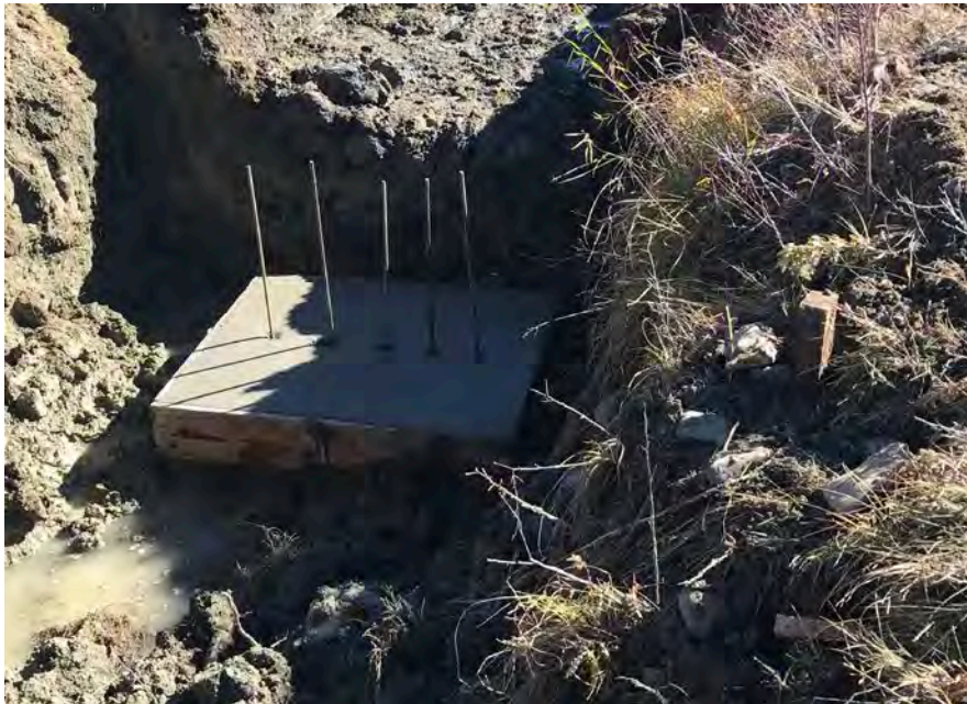
16. View of the finished concrete placement for the downstream discharge structure.
