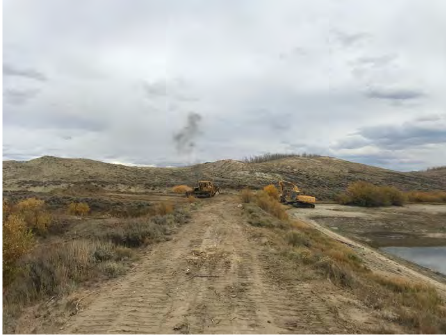
1. View of RLW beginning the excavation of the mid-level outlet
