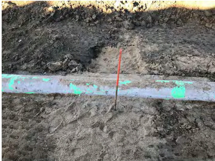
36. View of filter diaphragm installed to the spring line of the outlet conduit.
