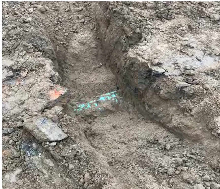
48. View of the filter diaphragm installation prior to ASTM C33 sand being installed.
