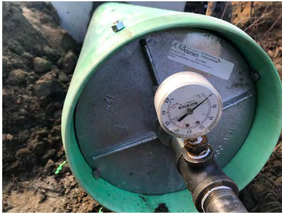
38. Close up view of the pressure test. Note pressure was held at 5 psi.
