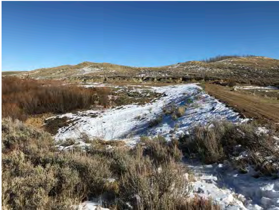
60. View looking right across the downstream slope.
