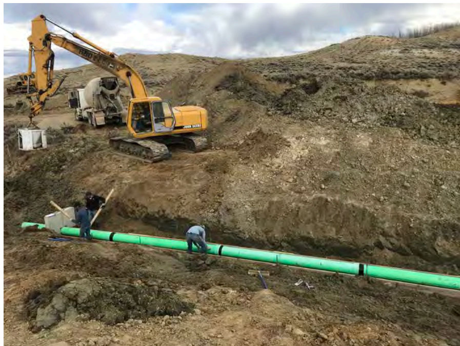
30. View of RLW forming the concrete cradle for the outlet pipe.
