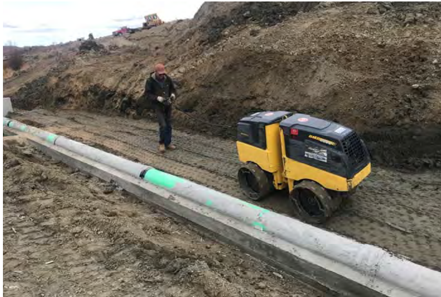
34. View of the backfilling and compaction of the embankment material around the pipe cradle.
