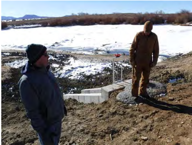
Photo 3 Waste concrete pad to facilitate gate access at high water levels
