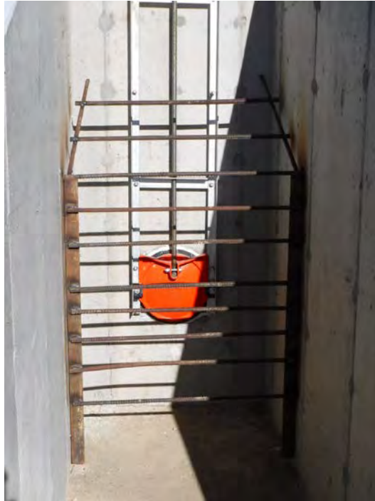
Photo 1 New gate and trash rack
