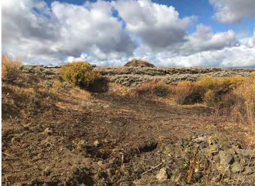
7. View looking left across the downstream slope at the clearing and grubbing work done to remove vegetation along the slope.
