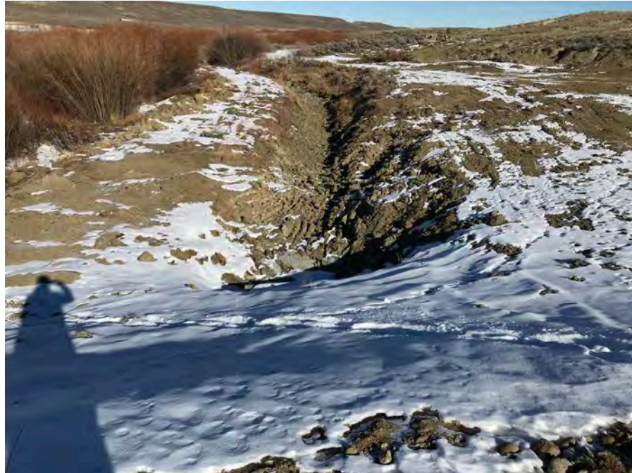
51. View looking downstream at the mid-level outlet discharge channel and downstream slope.
