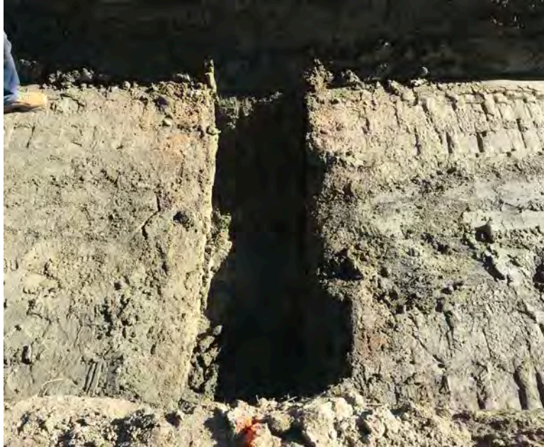
25. Close up view of the filter diaphragm trench below the pipe.
