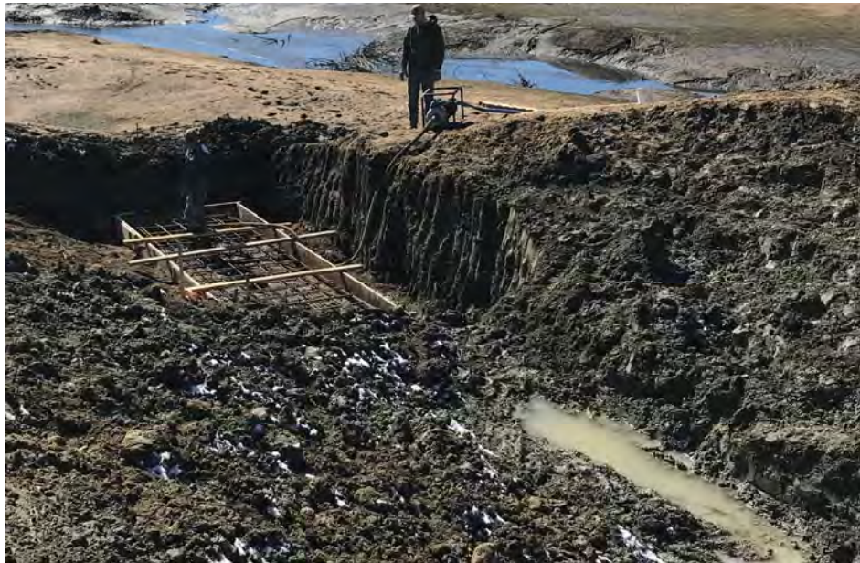
12. View looking upstream at the intake structure footing prior to concrete installation.
