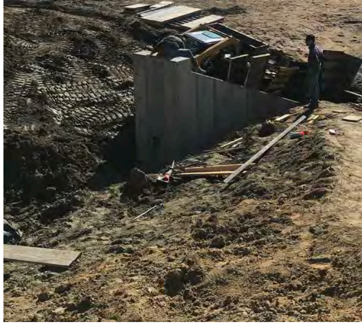
23. View of the completed intake structure following removal of the forms.
