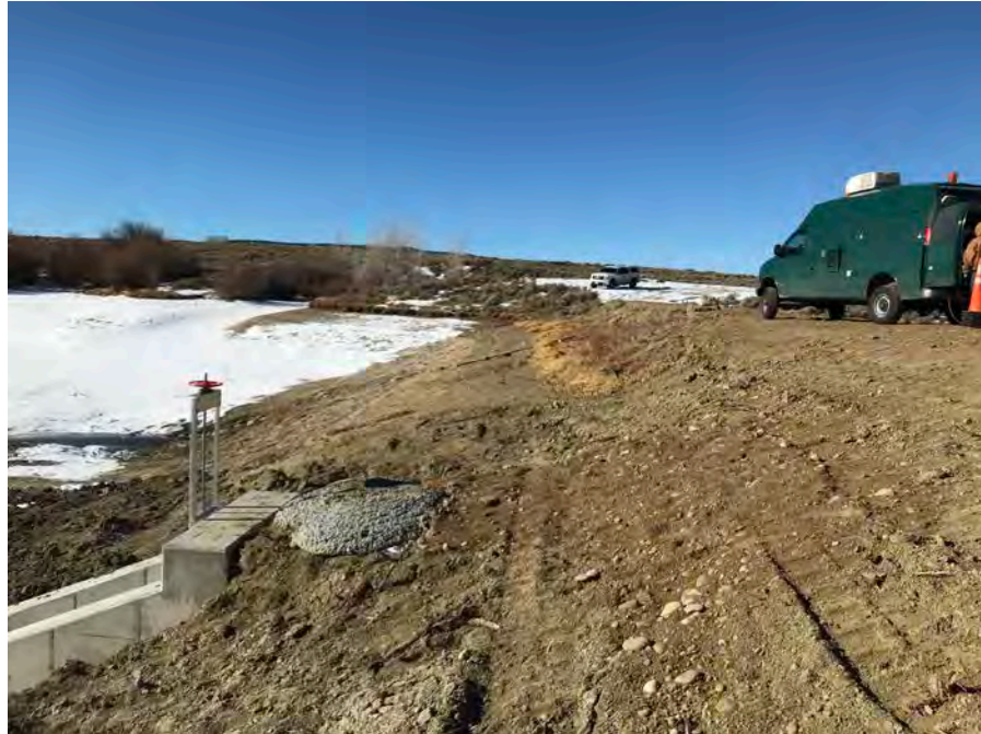
57. View looking left across the completed upstream slope.
