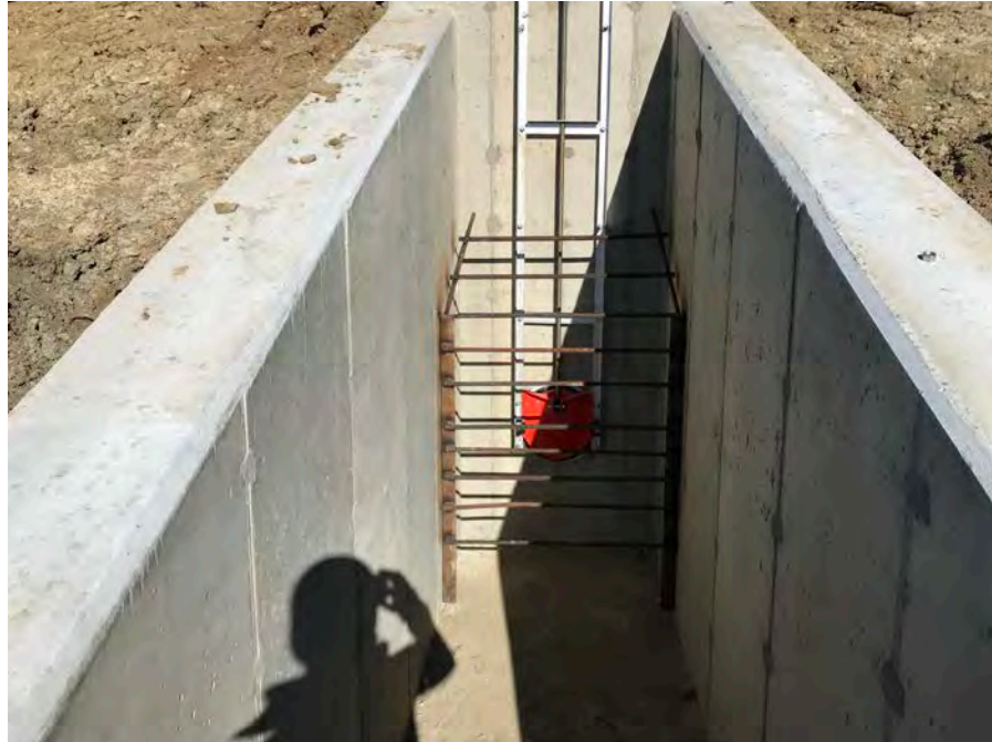
55. Close up view of the intake structure gate and trashrack.
