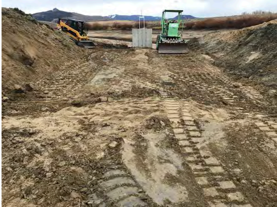
49. View of the completed filter diaphragm installed 2-feet above the outlet conduit.
