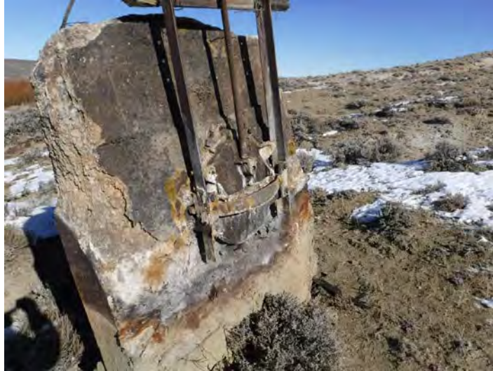
Photo 6 Removed downstream outlet gate
