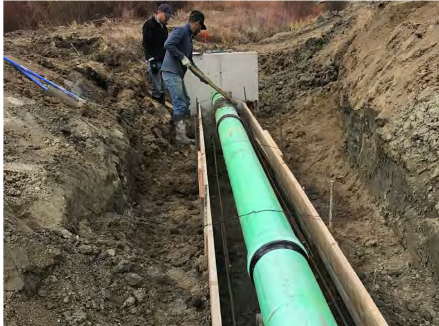
31. View of the concrete cradle reinforcement and formwork.
