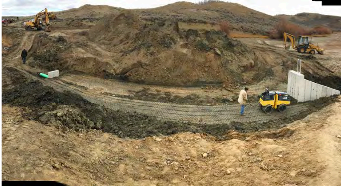
45. General panoramic view of the backfill and compaction for the mid-level outlet.
