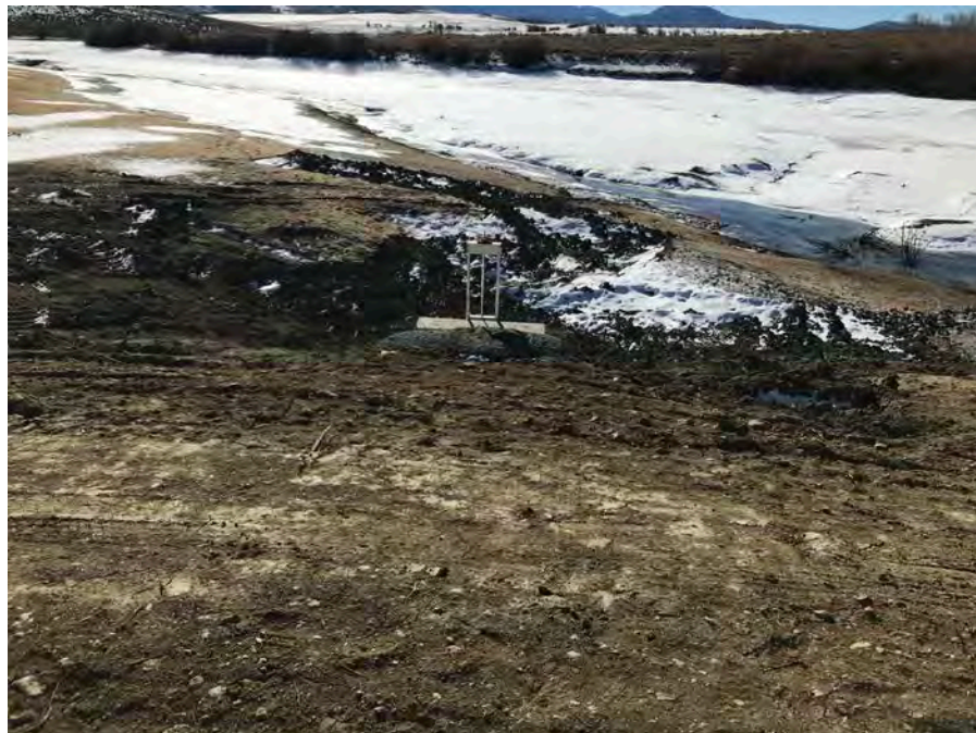
52. View looking upstream at the completed slope and intake structure.
