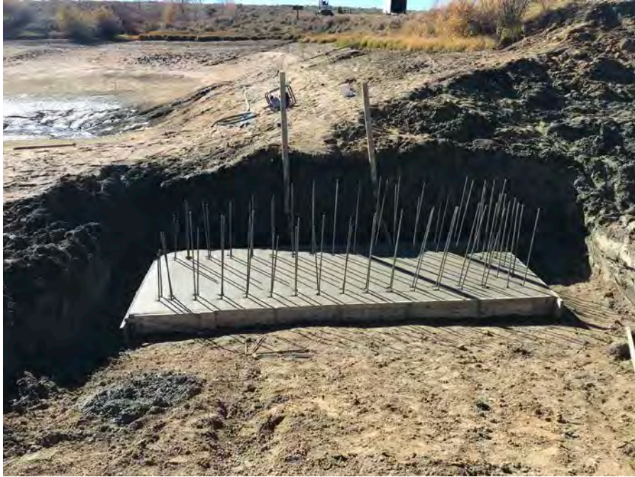
15. View of the finished concrete placement for the intake structure footing concrete.
