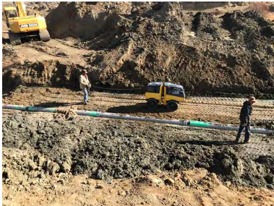
44. View of the embankment lift compaction process.
