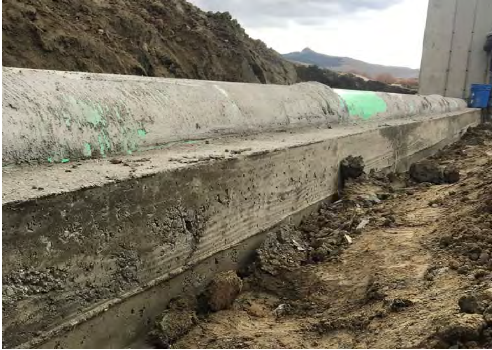
33. View of the completed concrete cradle for the mid-level outlet conduit.
