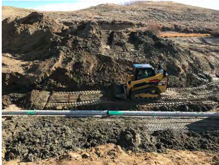
43. View of the embankment material spreading and compaction process.
