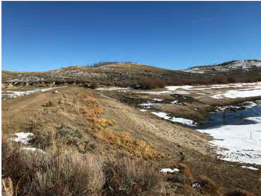
62. View looking right across the completed upstream slope.
