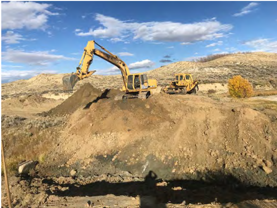
2. View of the mid-level outlet excavation.
