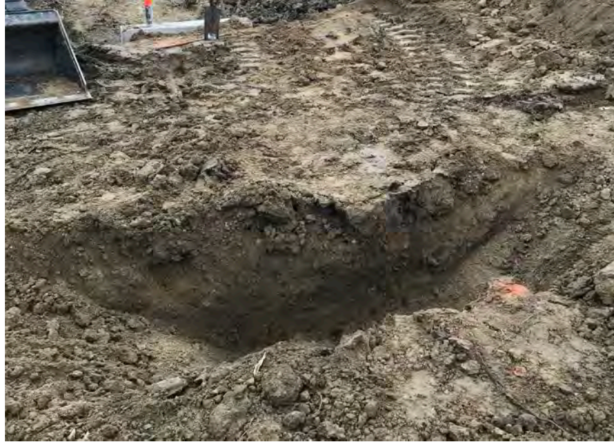
47. View of the filter diaphragm installation process after embankment lifts have been installed.
