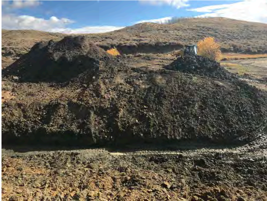
5. View of the exposed foundation preparation of the mid-level outlet.
