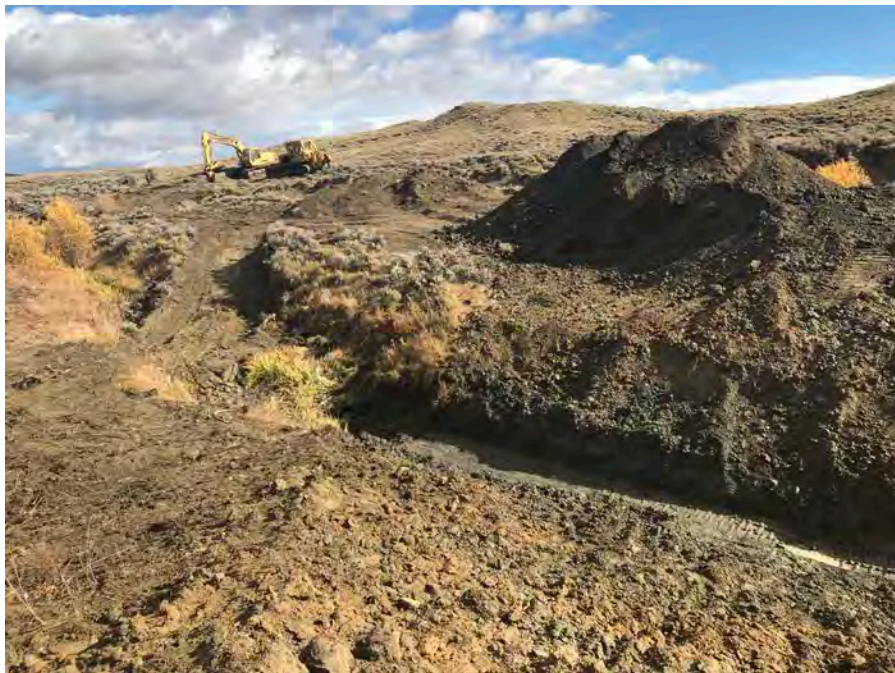
4. View of the of the exposed foundation looking downstream from the dam.
