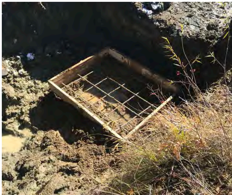
14. Close up view of the footing reinforcement for the downstream discharge structure.
