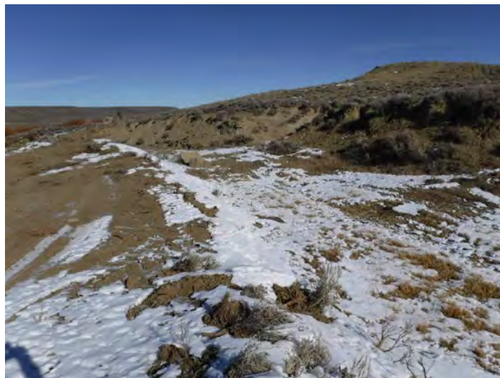
Photo 5 Small berm in the emergency spillway channel
