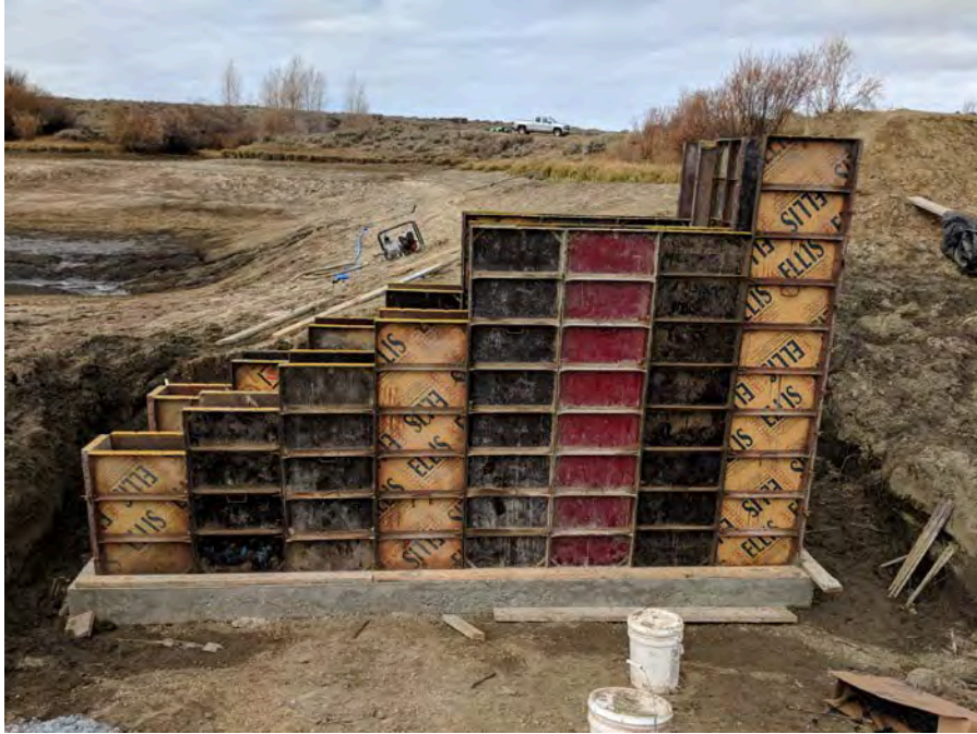
17. View looking left of the formwork for the right wingwall of the intake structure.
