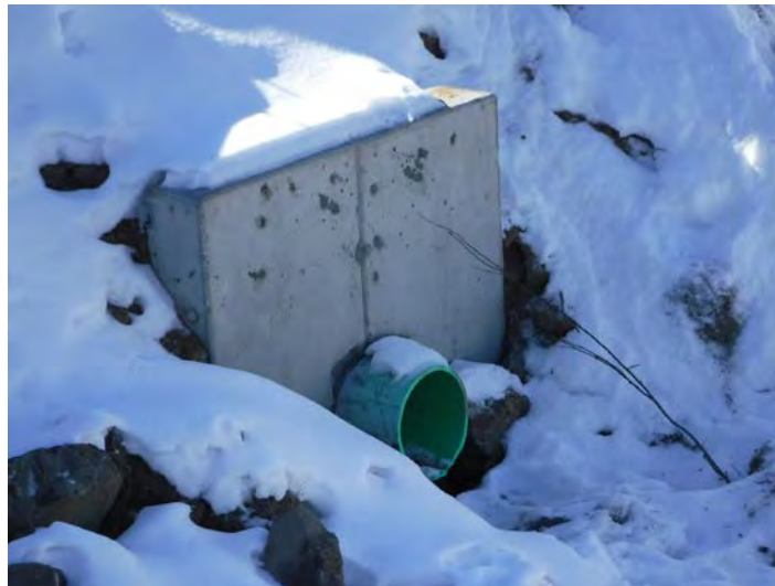
Photo 4 Downstream end of the new outlet
