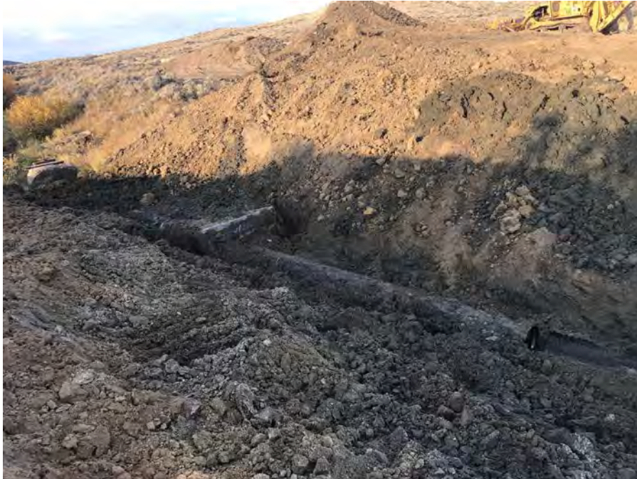
3. View of the exposed existing 18-inch diameter CMP mid-level outlet prior to removal.
