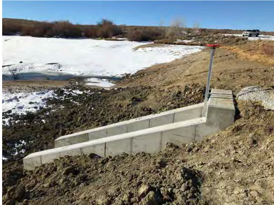
53. View looking left across the completed upstream slope and at the intake structure
