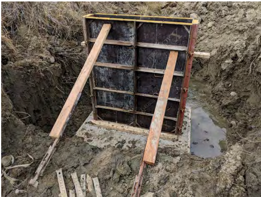
20. View of the formwork for the outlet discharge structure headwall.
