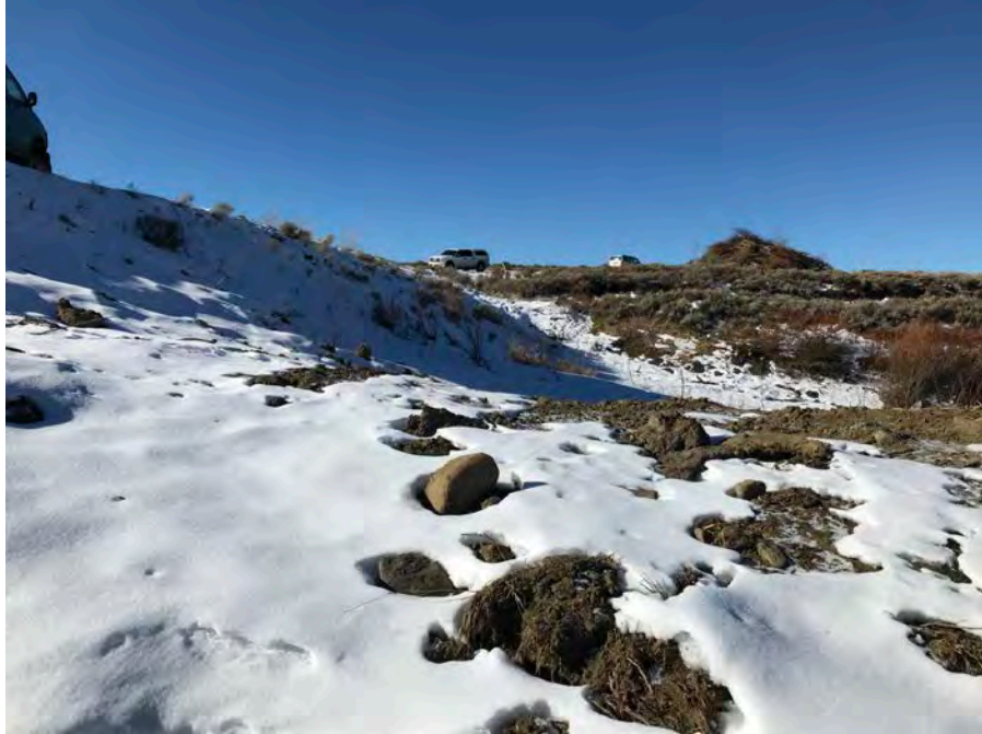
59. View looking left across the downstream slope. Note the vegetation has been removed.
