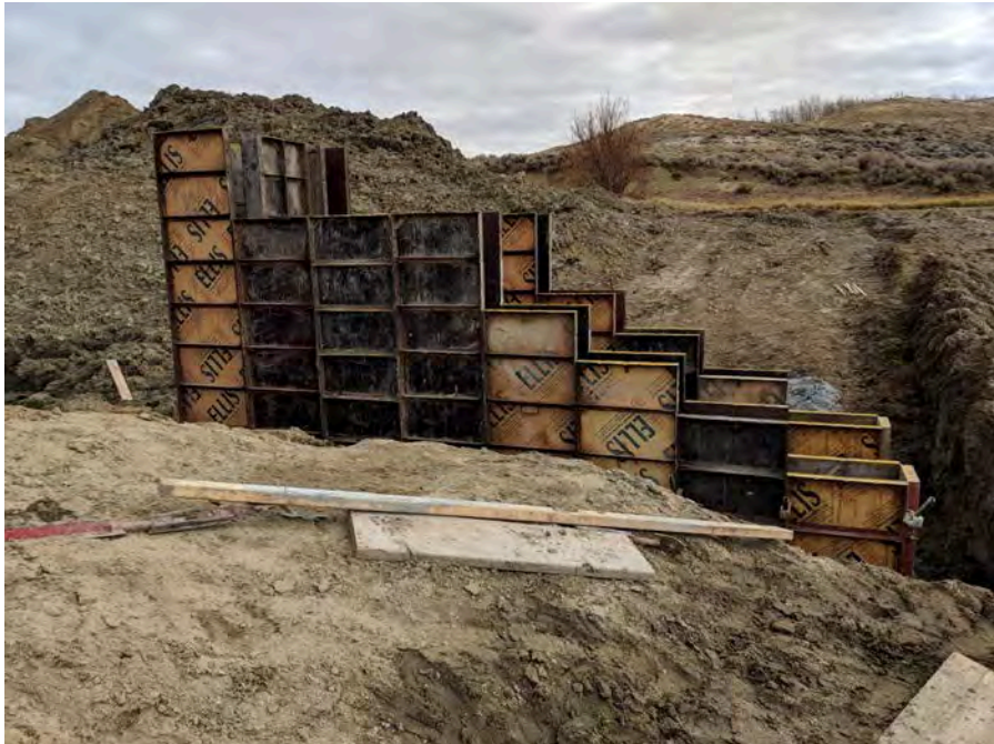
18. View looking right of the formwork for the left wingwall of the intake structure.
