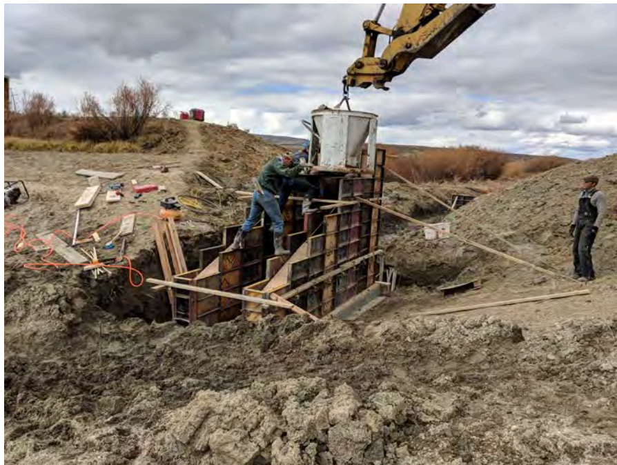
22. View of the concrete placement of the intake structure headwall and wingwalls.
