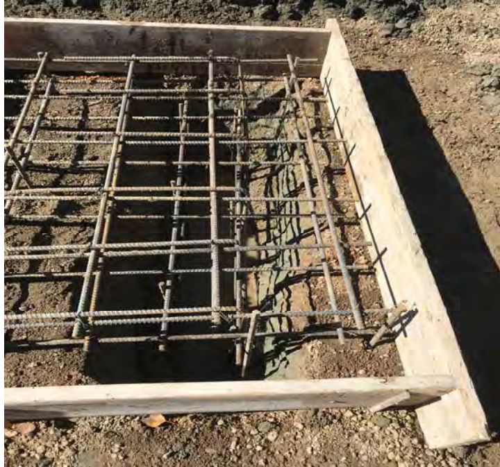
11. Close up view of the intake structure cutoff wall steel prior to concrete installation.
