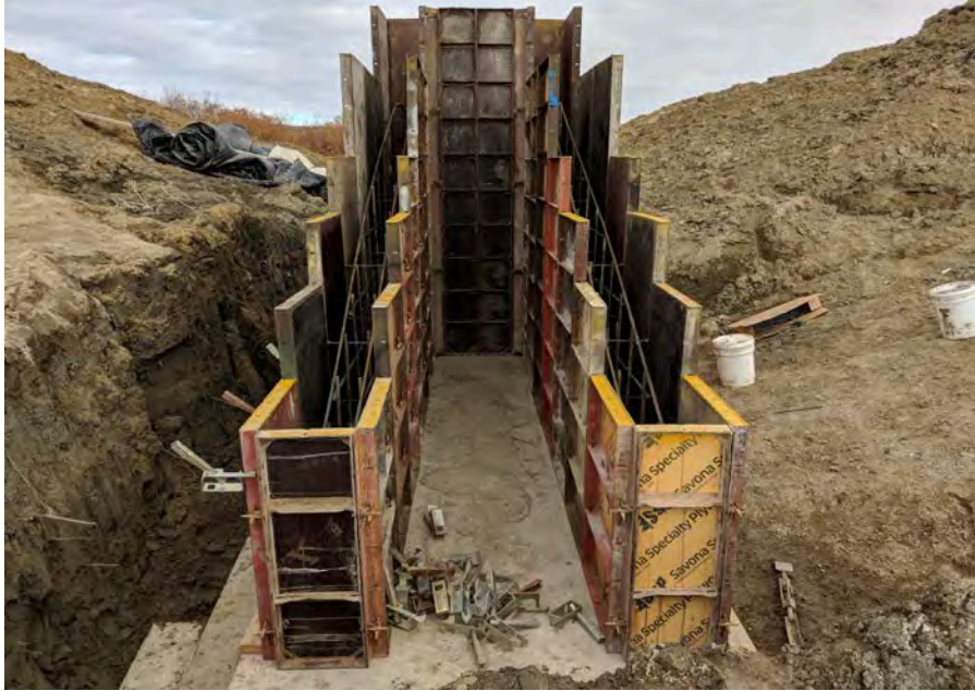
19. View of formwork and reinforcing steel for the intake structure.
