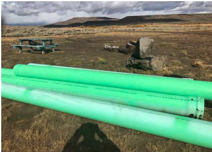
8. View looking at the 12-inch diameter SDR 35 PVC pipe that will be installed as the mid-level outlet conduit.
