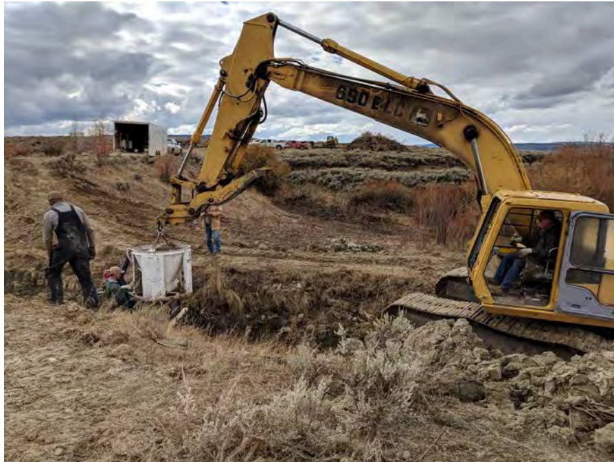
21. View of concrete placement of the outlet discharge headwall.
