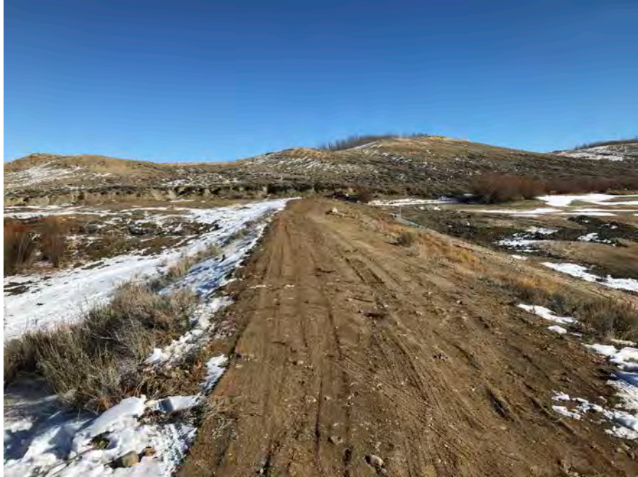
61. View looking right across the dam crest. Note the new road base added.
