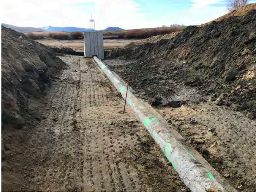
41. View of the filter diaphragm and embankment backfill looking upstream from the outlet.
