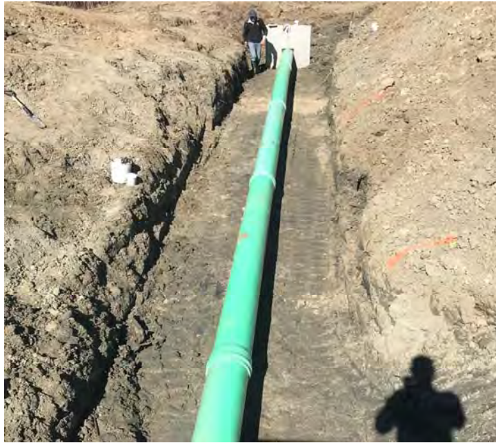
27. View of the 12-inch diameter SDR 35 PVC outlet pipe being installed.
