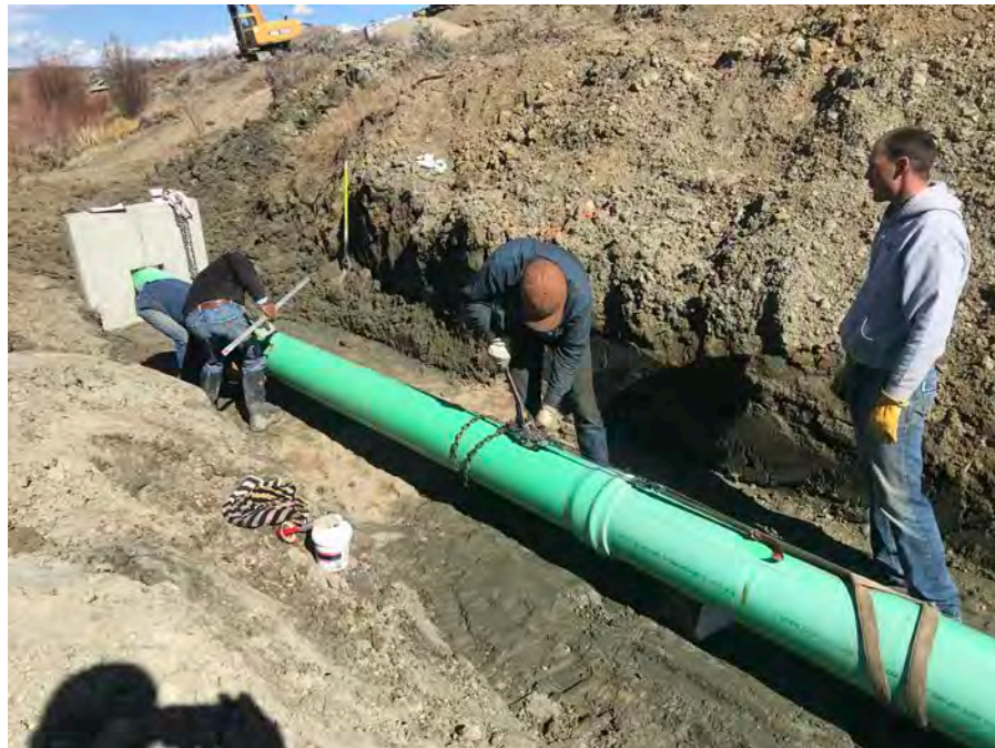
29. View of the mid-level outlet conduit installation.
