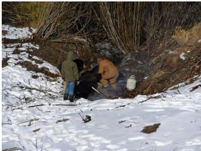
Photo 8 Heating the pipe to remove ice jam for inspection of the low level outlet
