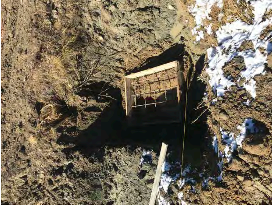
13. General view of the footing reinforcement for the mid-level outlet downstream discharge structure.
