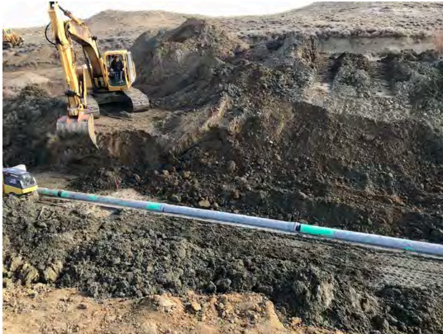
42. General view of the embankment backfill process around the mid-level outlet.
