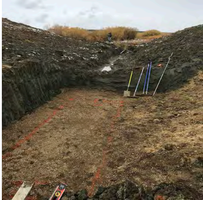
9. View of the final subgrade preparation for the new mid-level intake structure.
