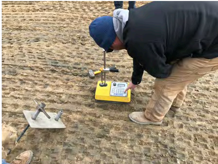
46. View of a typical compaction test being completed on an embankment lift.
