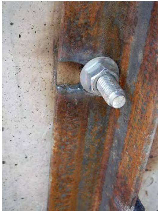
Photo 2 Notch for easy trash rack removal
