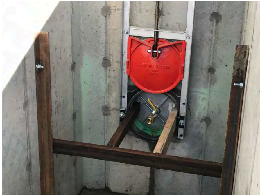
39. View of the pressure test setup at the intake structure.
