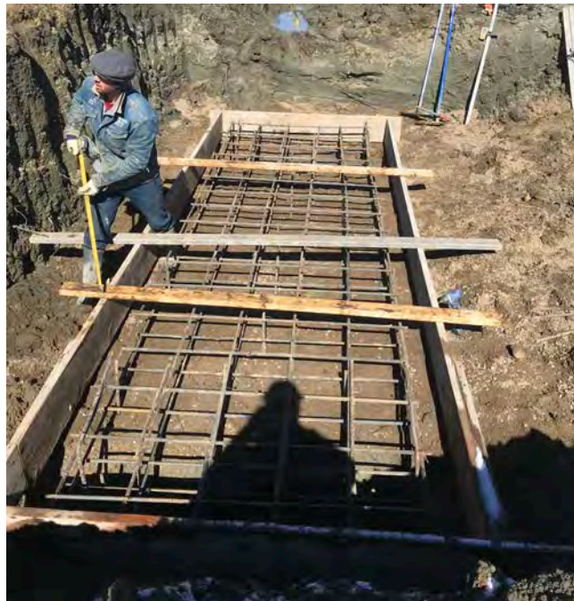
10. View of the intake structure footing steel and formwork
