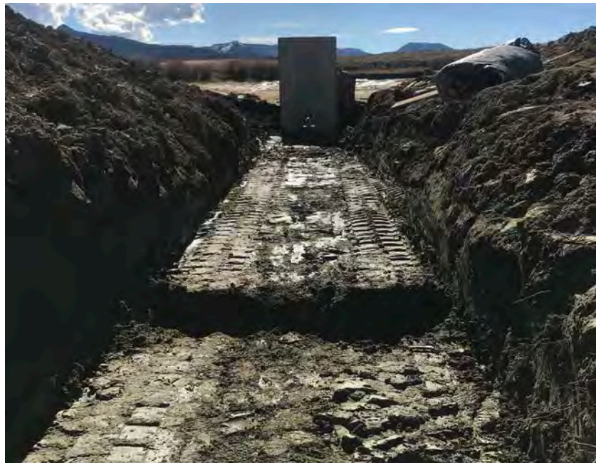
24. View looking upstream at the final grade and filter diaphragm trench prior to installation of the outlet pipe.
