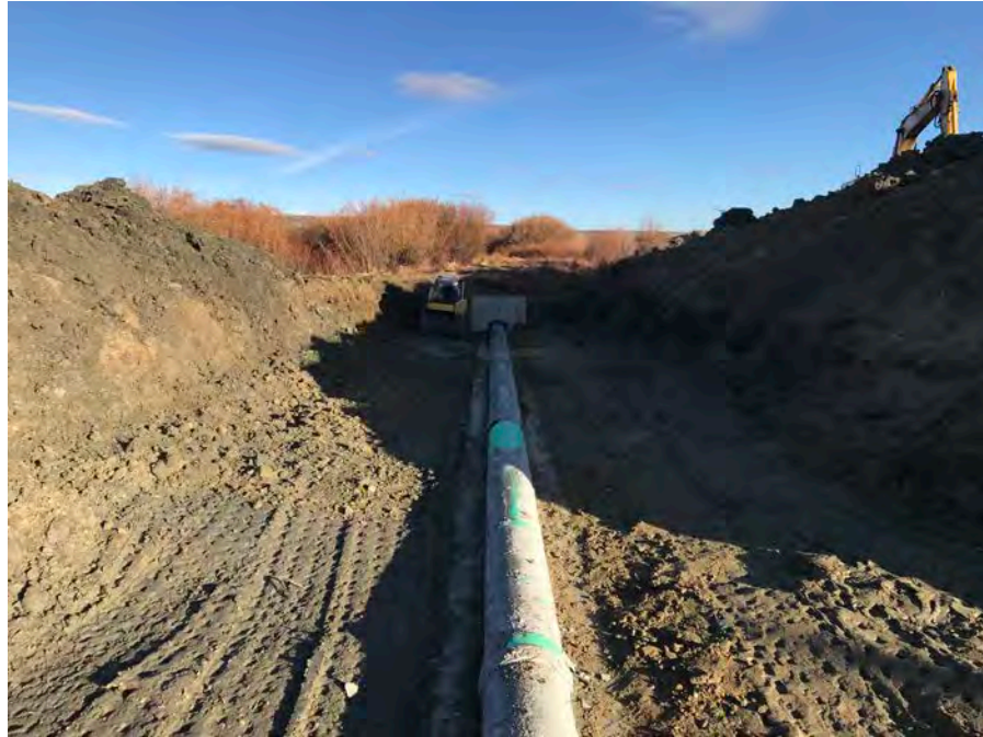
35. View of the embankment compaction up to the spring line of the outlet conduit.
