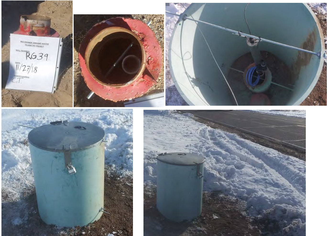
Picture 55, 56, 57, 58, 59: RG 39 telemetry well site installation. Pictures 55 and 56 show the well before installation. Pictures 57, 58, 59: Shows the construction of the vault over RG 39 to place the tube for the well. RG 39 is on County Line Road 8.6 miles north of Highway 160 in Alamosa County.
