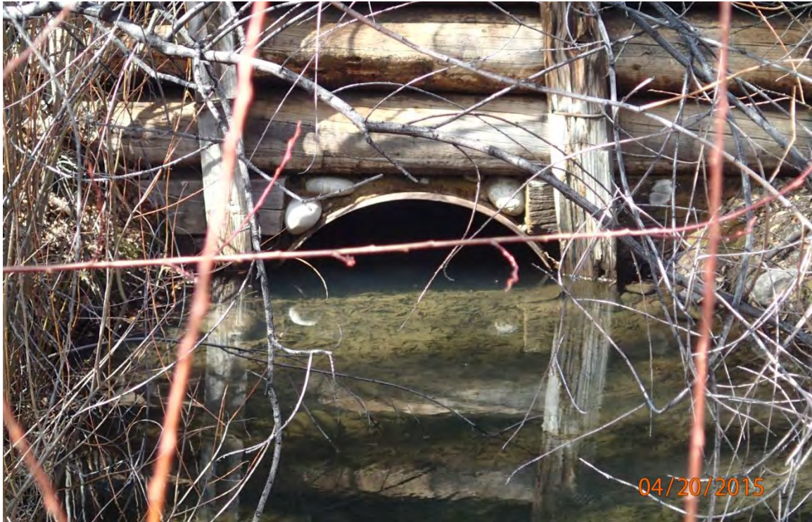
Figure 2. Outlet of the head gate culvert showing accumulation of sediment with adverse impacts on flows into the Piloni Ditch.
