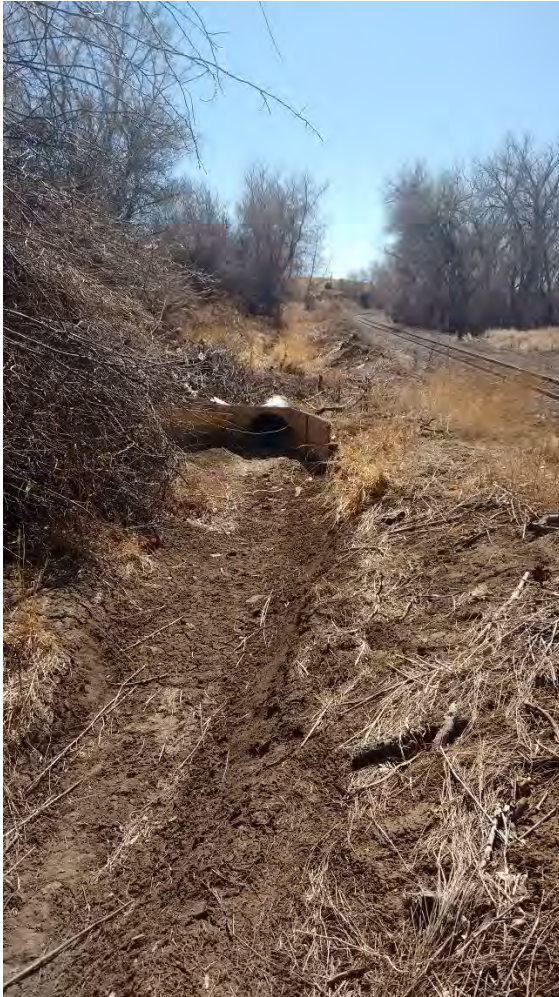
Chilili Ditch section – pre-construction.
