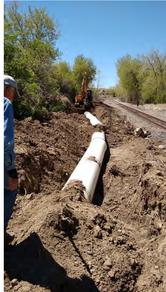
Chilili Ditch section – 30" diameter pipe construction.
