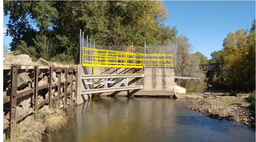
Picketwire Ditch headgate – post-construction.
