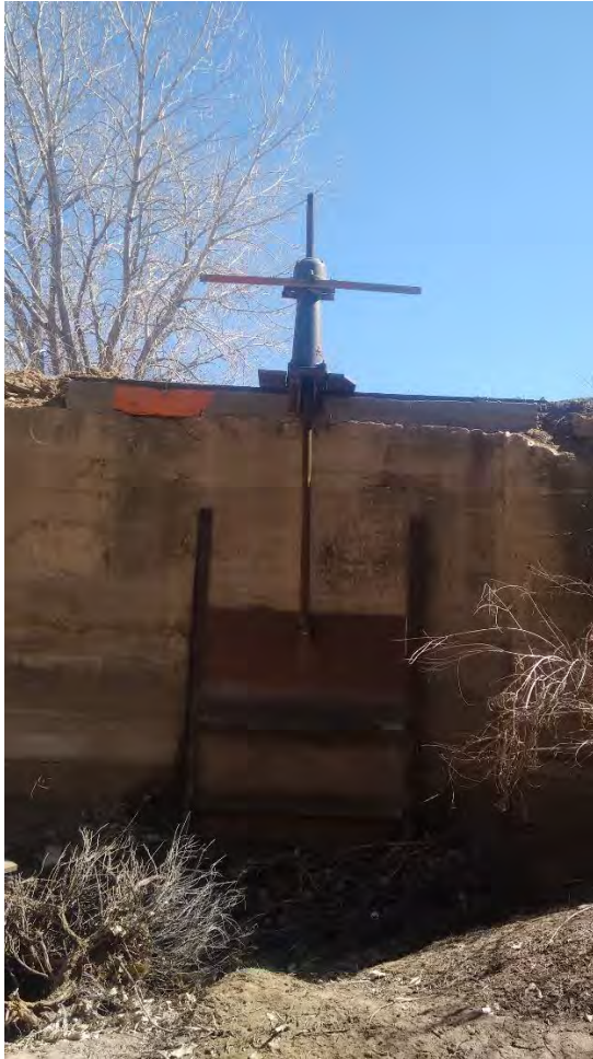
John Flood Ditch headgate pre-reconstruction.
