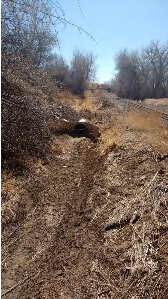
Chilili Ditch section – pre-construction.
