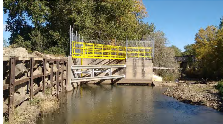
Picketwire Ditch headgate – post-construction.
