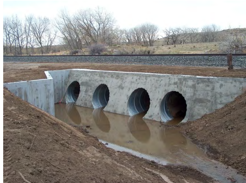
Enlarged Southside Irrigation Ditch Railroad Crossing, pre-construction and post-construction.
