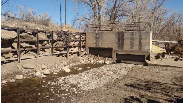
Picketwire Ditch headgate – pre-construction.
