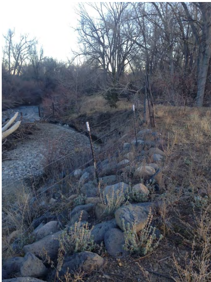
Southside Ditch headgate downstream area – pre-construction.
