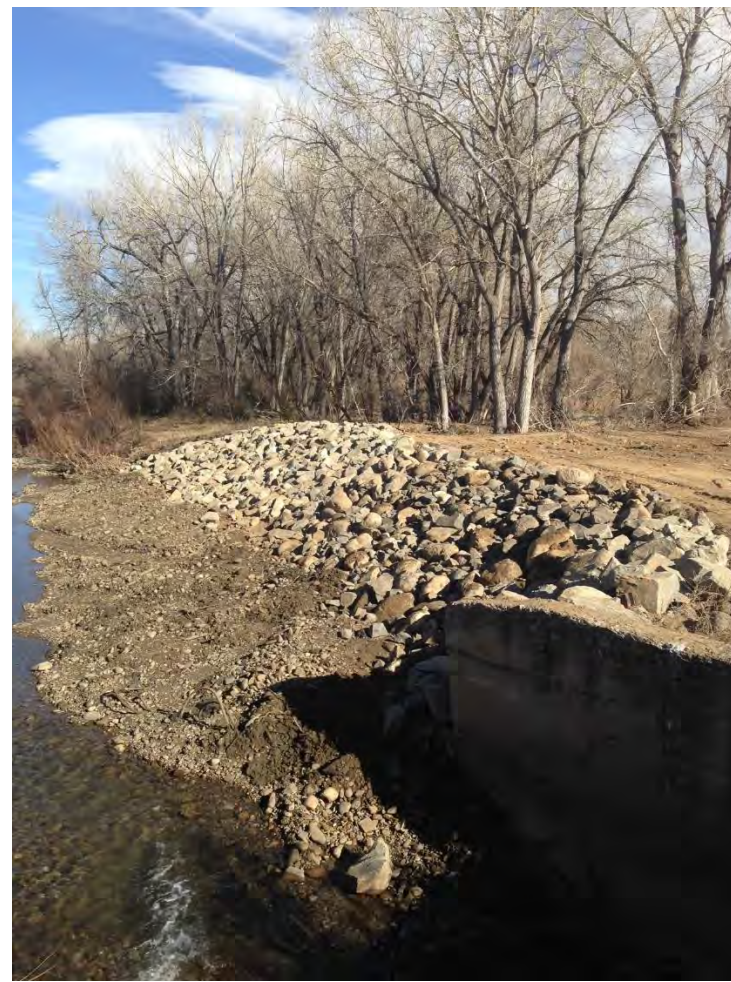
Southside Ditch headgate downstream area – post-construction.
