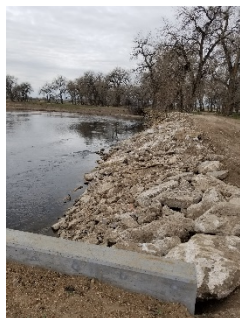
Figures 4 & 5 - Bank stabilization upstream and downstream of diversion structure.
