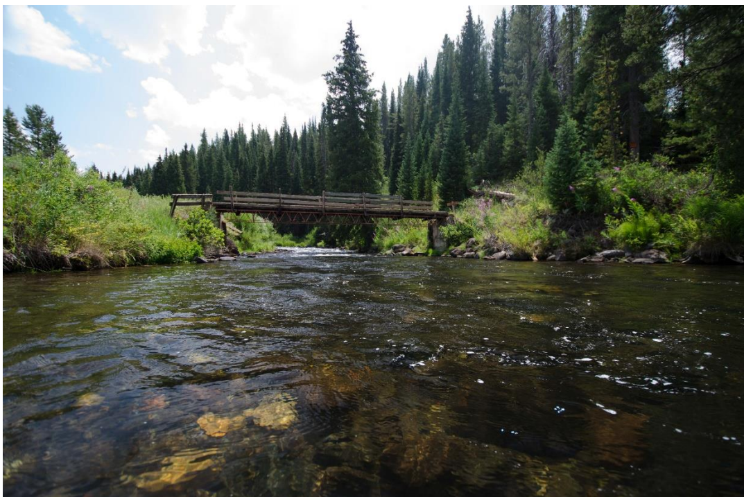
North Fork White River above Ripple Creek, Cross Section 2, looking upstream.
