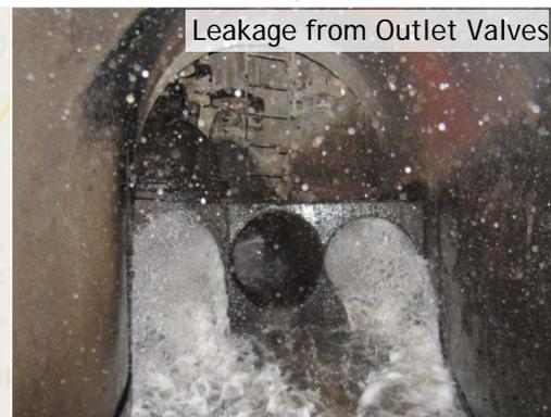
Leakage from Outlet Valves
