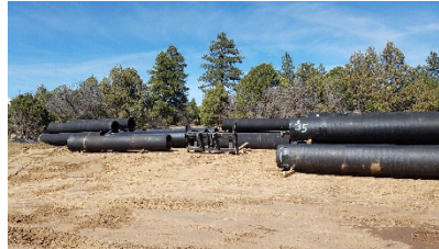
Figure 2 - 30 in. DIP pipe
