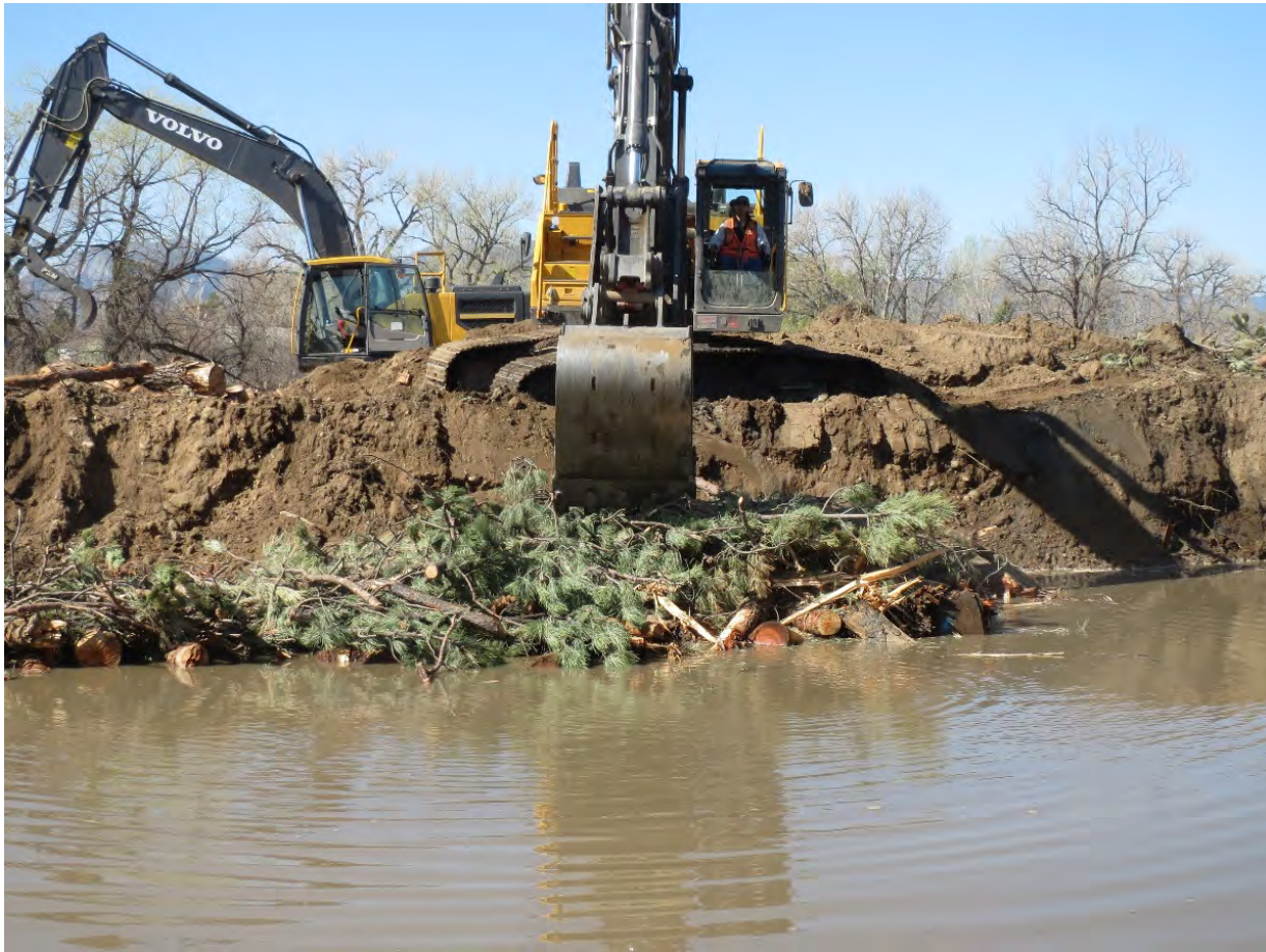
Photo 13. Installing base of wood toe structure.
