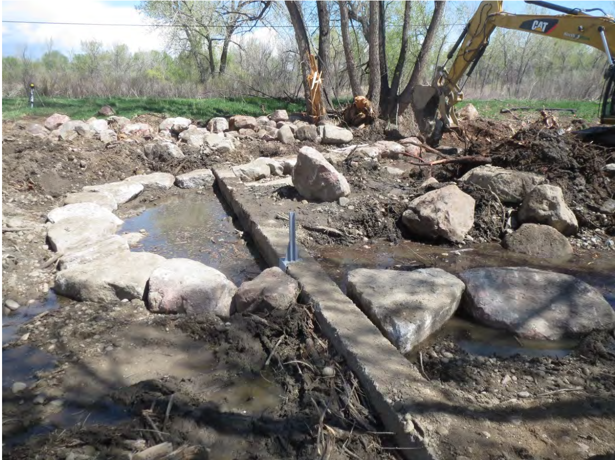
Photo 7. Constructing the rock “A” cross vane that will allow diversion. Note existing low head diversion dam around which the cross vane is being built. View looking right bank to left bank.
