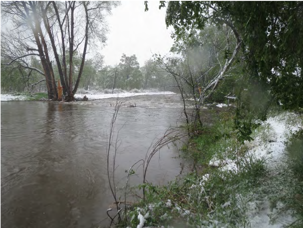
Photo 9. Rock cross vane under high flow (approximately 500 cfs). View facing downstream.
