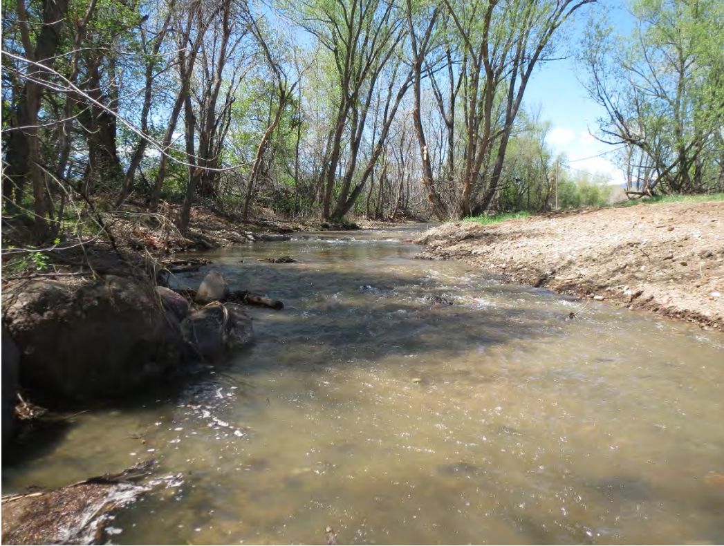
Photo 5. Constructed riffle at low flow. View looking upstream from end of project reach.
