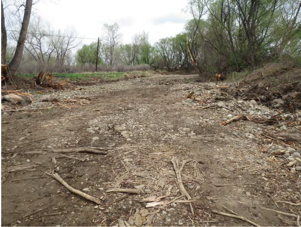
Photo 3. Raised creek bed. View looking downstream from the existing low head diversion dam.
