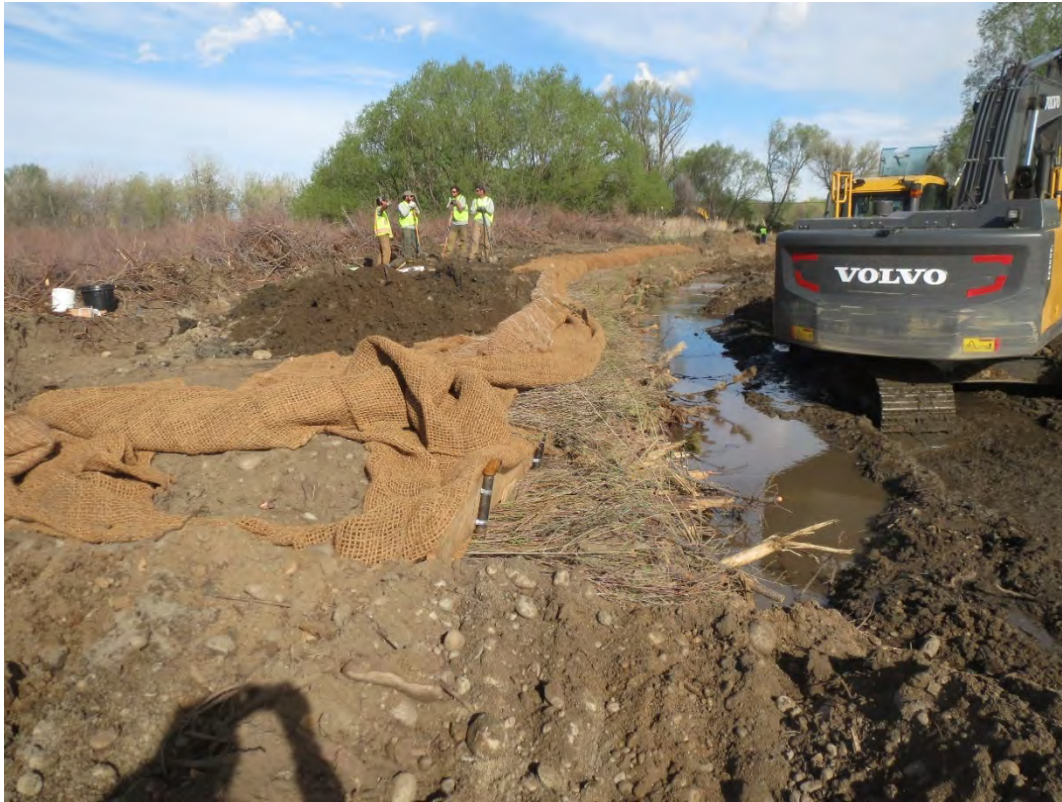
Photo 14. Installing soil encapsulated lifts with live willow and cottonwood branches on top of wood toe structure.
