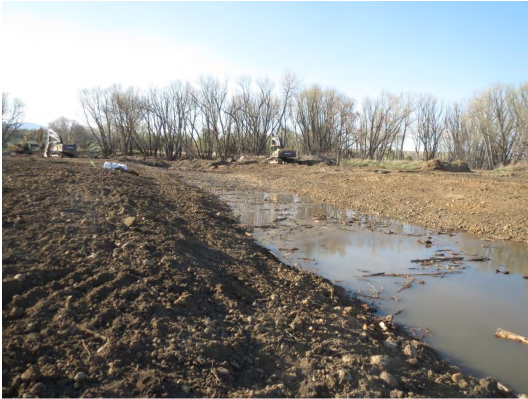
Photo 11. New channel prior to water flowing in it. Inner berm and gently sloping banks to bankfull are clearly visible on the river right bank. View facing upstream.
