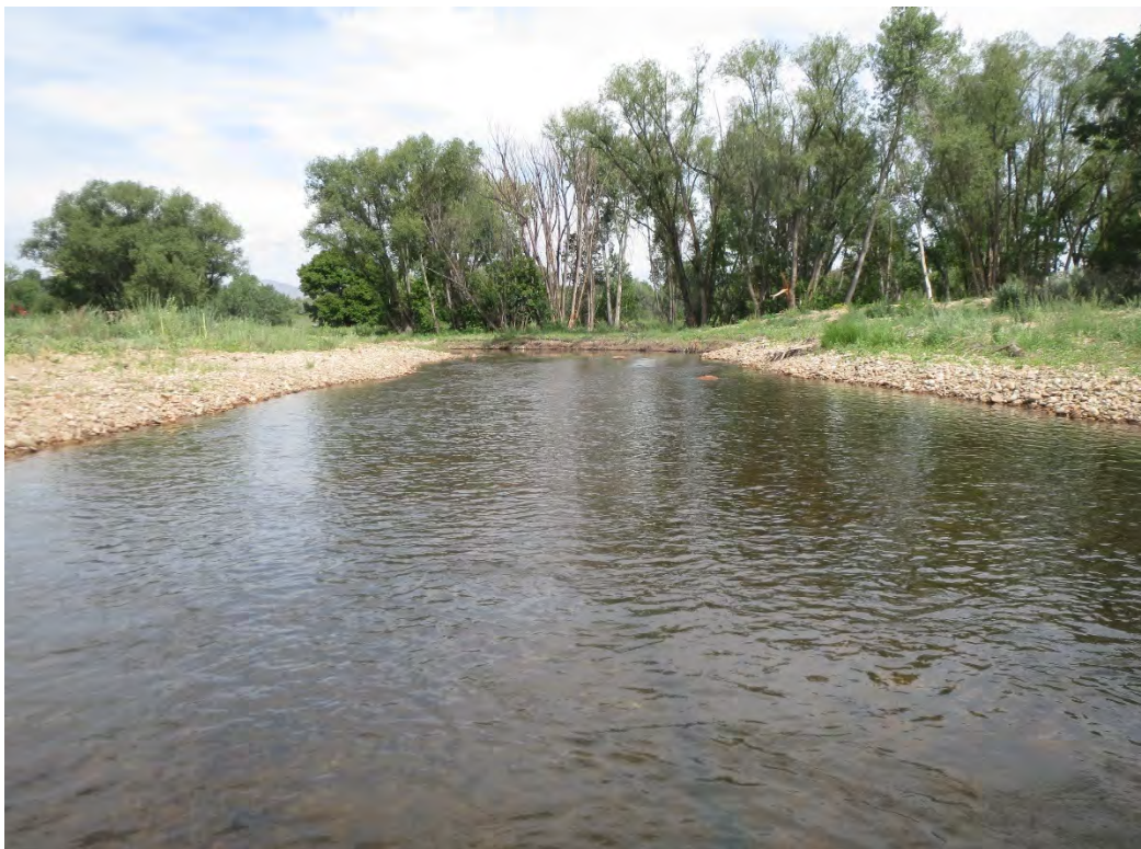
Photo 33. Re-aligned reach constructed with a more stable plan view and dimension. Wood toe visible at bend in background. View facing upstream August 17, 2017.
