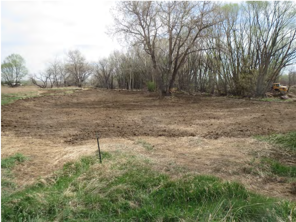
Photo 16. Lowering of left floodplain. View facing east from 61 st Street.
