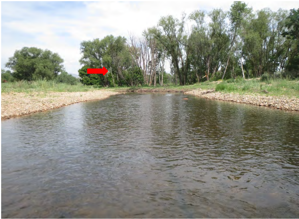
Photo 25. Following restoration wood toe replaces riprap (left bank), creek channel dimensions more closely approximate reference conditions, and riparian corridor seeded and planted with native vegetation. View facing upstream August 17, 2017.
