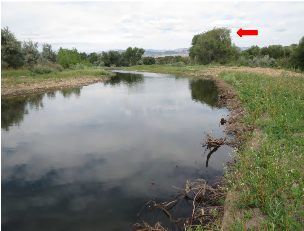
Photo 31. Close up of wood toe and realigned plan form of restored creek. View facing upstream August 17, 2017.
