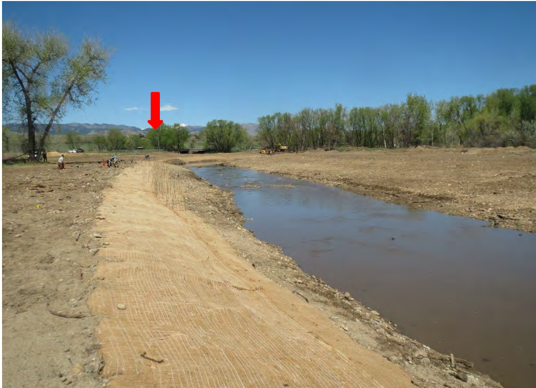
Photo 17. New floodplain along creek. Note levee in background of the photo on the left bank. Prior to the project, the levee bordered the creek's left edge. Floodplain grading and relocation of the creek has expanded the floodplain. View facing downstream.
