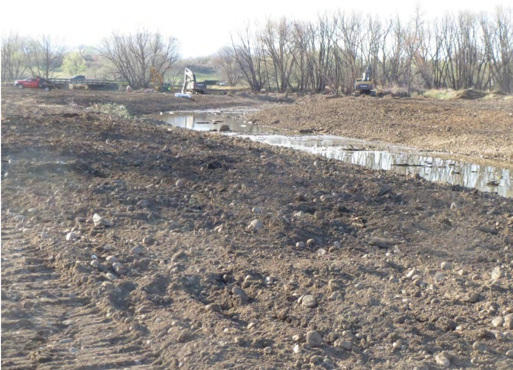
Photo 12. Sinuosity is returned to the channel. View facing upstream.
