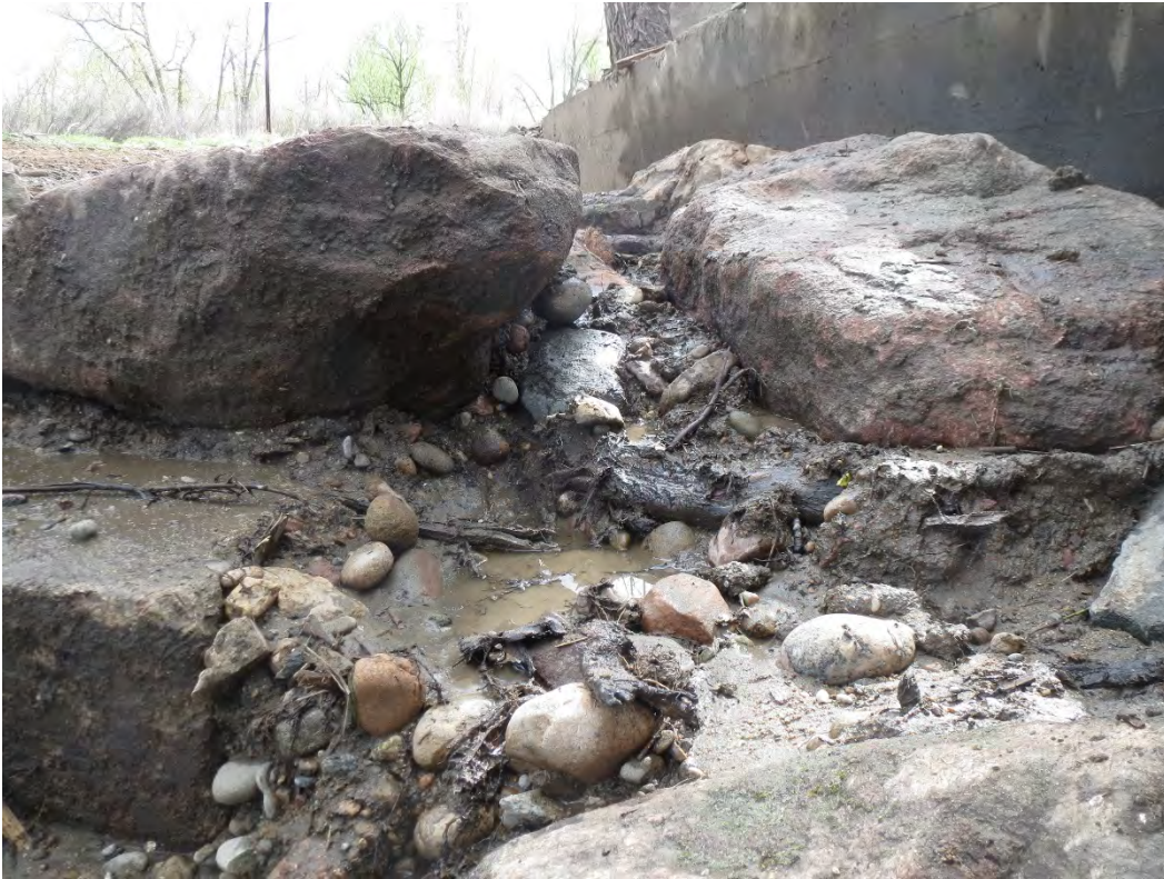
Photo 8. Fish “escape path” in the rock cross vane adjacent to the new headgate.
