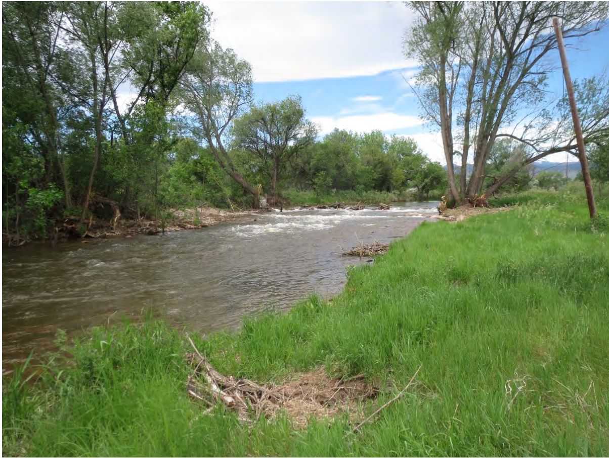
Photo 10. Rock cross vane and raised creek bed. View facing upstream.
