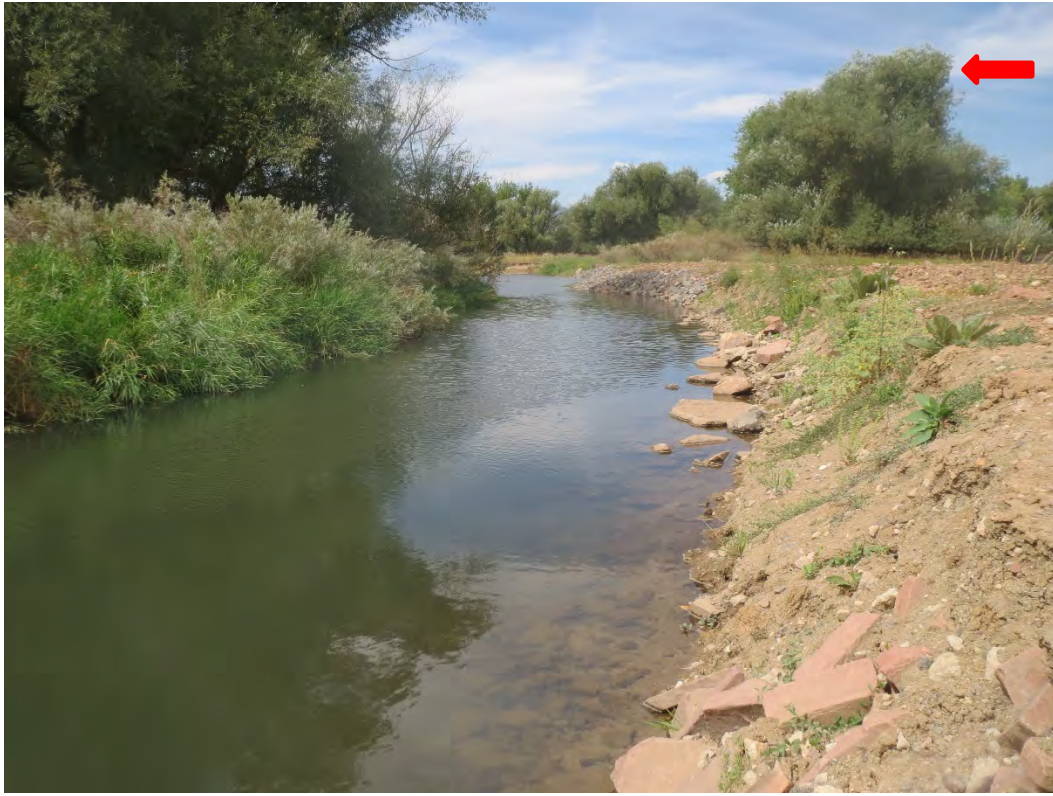
Photo 30. Close up of temporary riprap berm. View facing upstream September 7, 2016.
