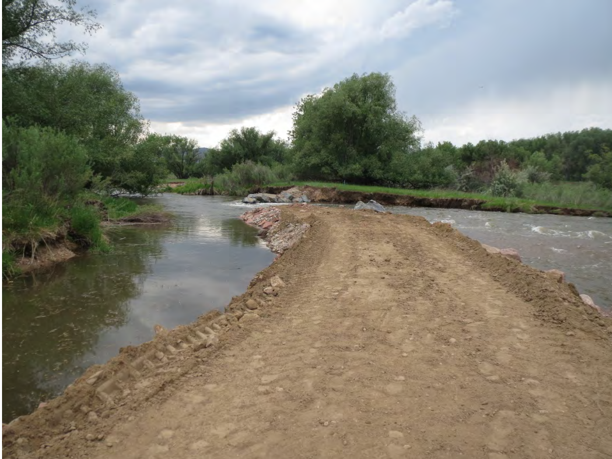
Photo 1. Temporary berm being constructed across the Boulder Creek breach to redirect the creek back into its pre-flood channel.
