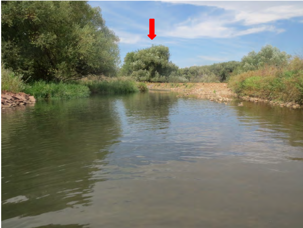
Photo 22. Second view of temporary riprap and entrenched channel. View facing upstream September 7, 2016.
