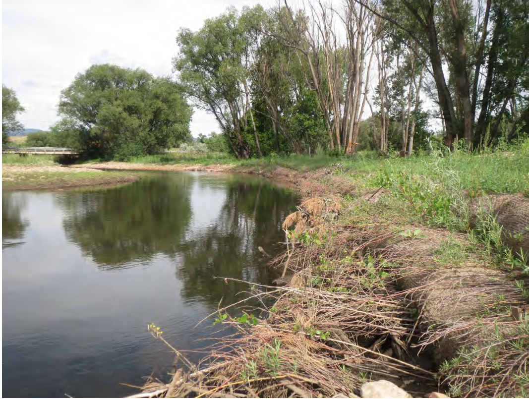
Photo 19. Willow and cottonwood cuttings sprouting in the soil lifts above a wood toe structure. View facing upstream.
