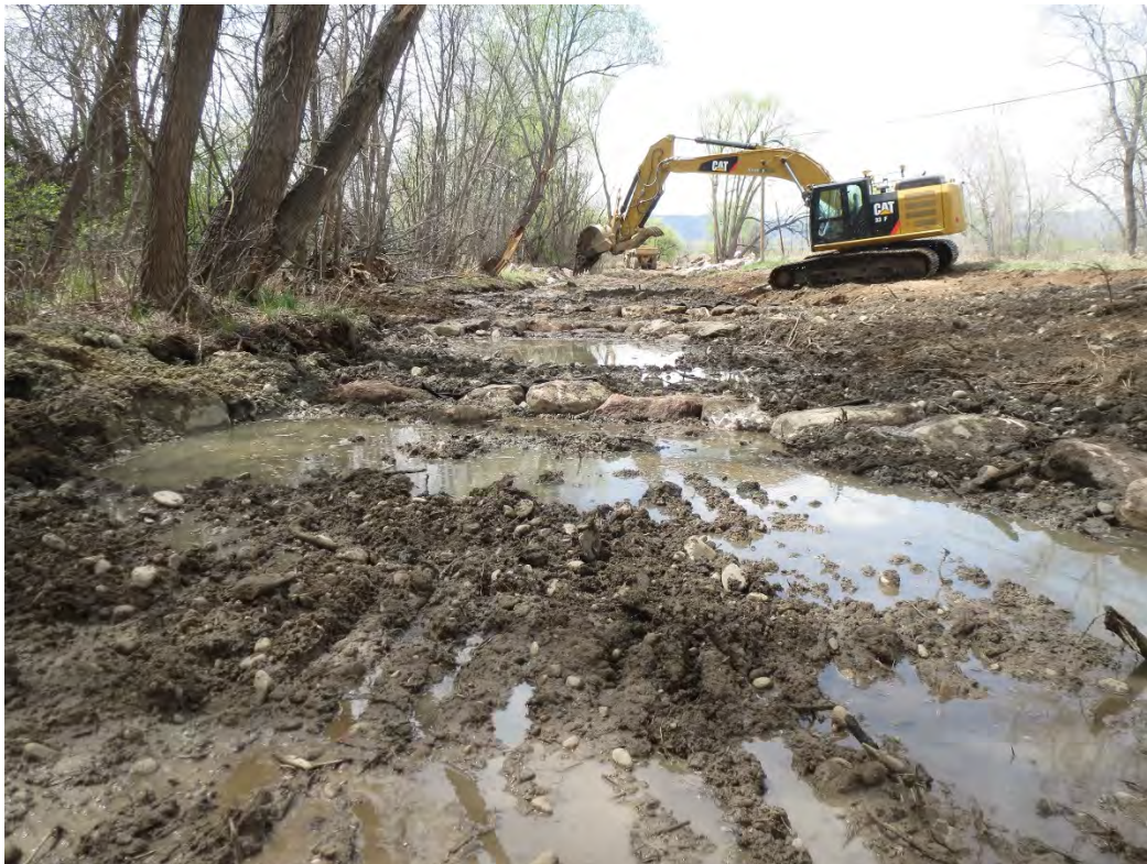
Photo 4. Boulder vanes being installed in the constructed riffles immediately downstream of the existing low head diversion dam. View looking upstream from end of project reach.
