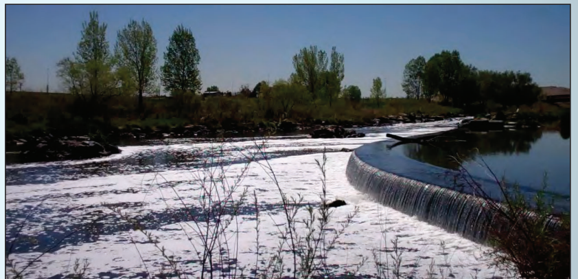
Drop structure adding oxygen to Segment 15 of the South Platte River
