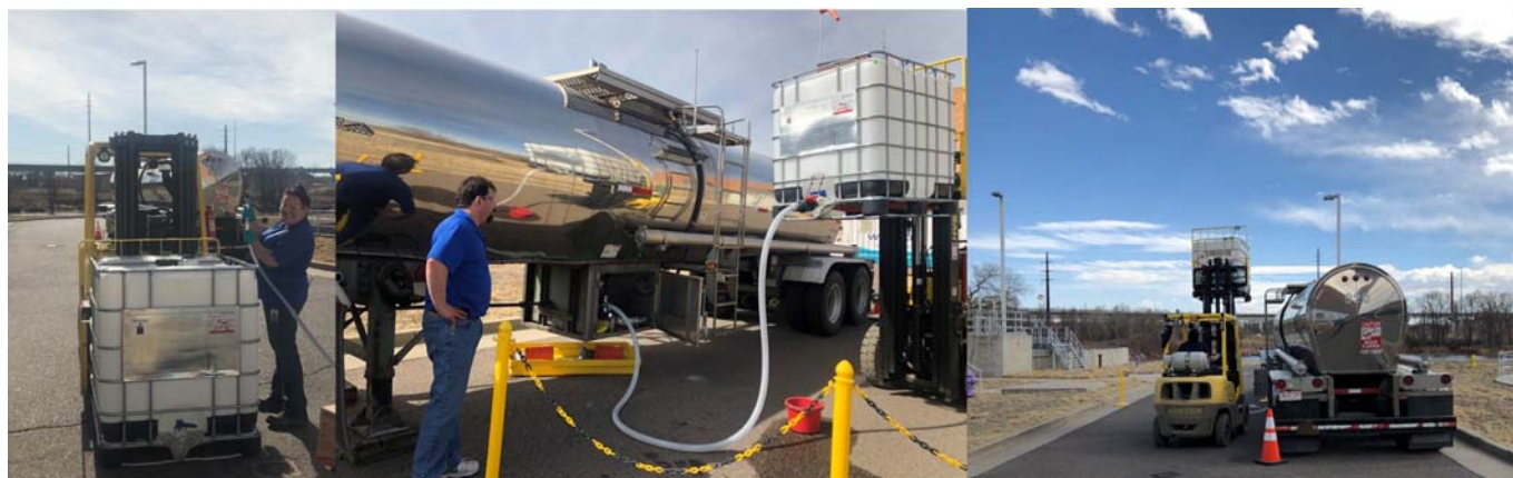
Figure 2. Purified Finished Water Collection and Tanker Filling
