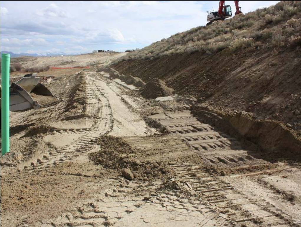
Photo 80. View looking right along the right side of the Main Dam seepage collection system from MTD Sta. 0+00 where the chimney drain and stability berm is still being constructed. Oct. 20, 2017.
