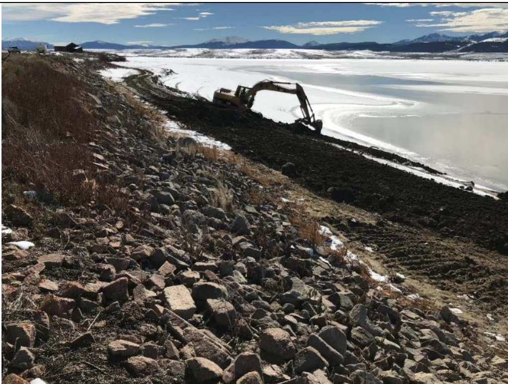
Photo 114. View looking right from Station 10+00 at the access road removal and upstream slope grading. Nov. 9, 2017.
