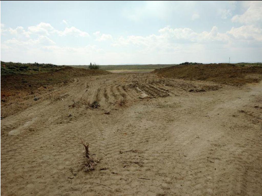
Photo 4. View looking upstream at the cleared and grubbed spillway from ES Station 2+75. Aug. 2, 2017.
