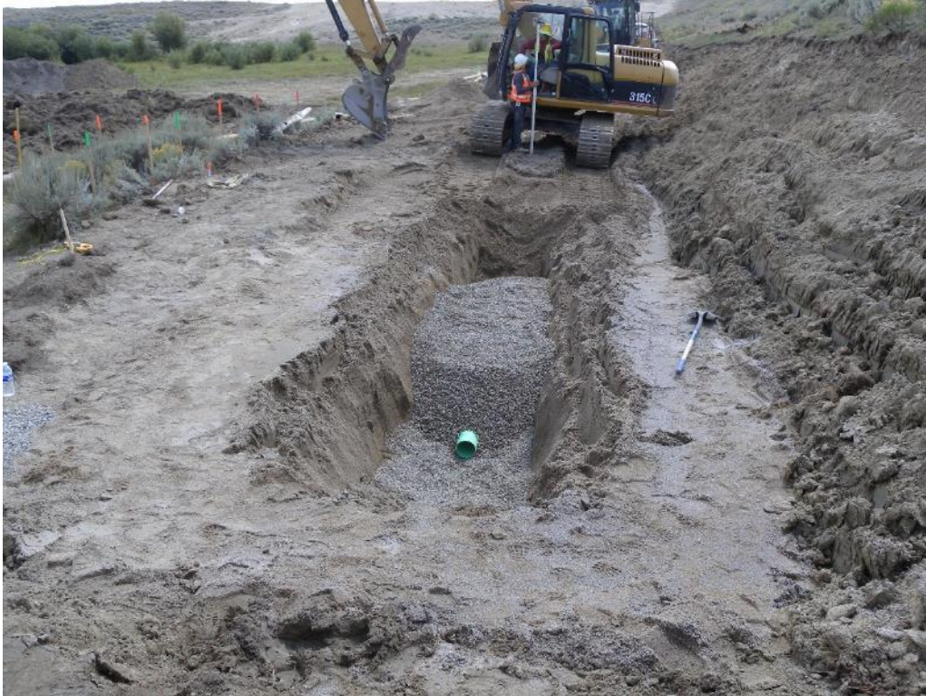
Photo 27. View looking right from MTD Sta. 2+50 and the first section of chimney drain and seepage collection pipe placed from MTD Sta. 2+55 to 2+70. Aug. 29, 2017.
