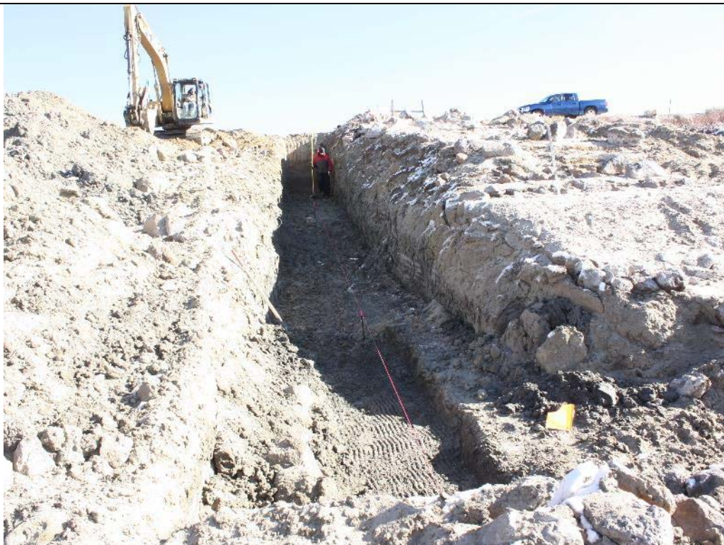
Photo 80. View looking downstream along the excavation for the Air Vent Encasement Wall and RME establishing the final required bottom grade. Oct. 22, 2017.
