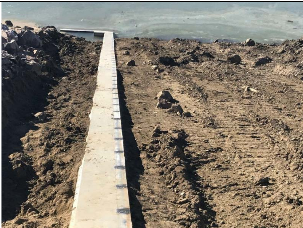
Photo 116. View looking down the air vent grade beam and staff gage. Note that the staff gage numbers are welded on the angle iron at 0.5-foot intervals. Note the additional grading and riprap that needs to be installed prior to completion. Nov. 13, 2017.
