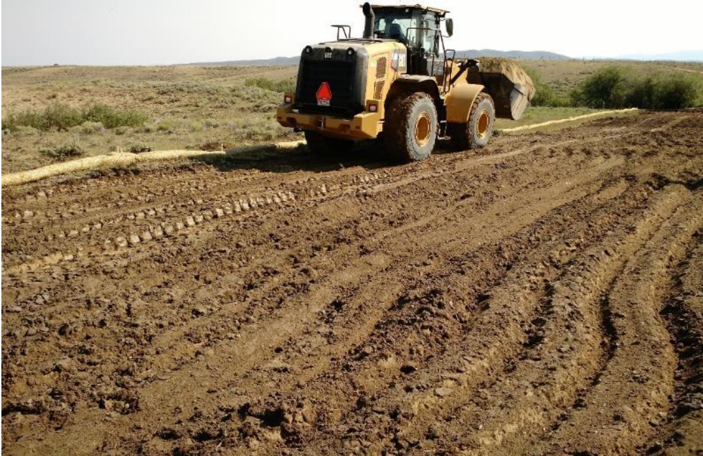
Photo 5. View of the spillway proof-rolling from approximate ES Stations 4+50 to 6+50. Aug. 3, 2017.
