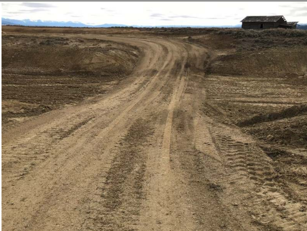
Photo 118. View looking right across the access road of the Emergency Spillway with basecourse placed on the road. Nov. 28, 2017.
