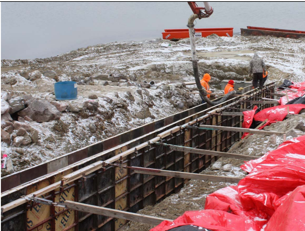
Photo 90. View looking upstream from near the dam crest at the placement of concrete by the pump truck into the Air Vent Encasement Wall. Oct. 30, 2017.
