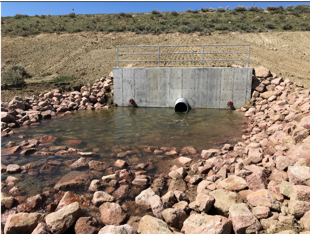
Photo 122. View of the terminal structure and plunge pool. Plunge pool was reworked and the water level lowered. Additional riprap armoring was installed on the right and left side of the headwall. May 17, 2018.
