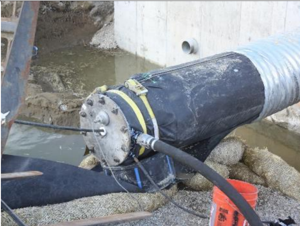
Photo 99. View looking right from the left side of the downstream end of the outlet conduit at the sealed end of the CIPP liner during inflation. C&L slowly raised the pressure within the CIPP liner to 450 mbar (6.2 psi) to expand the liner to fill the host pipe. Nov. 1, 2017.
