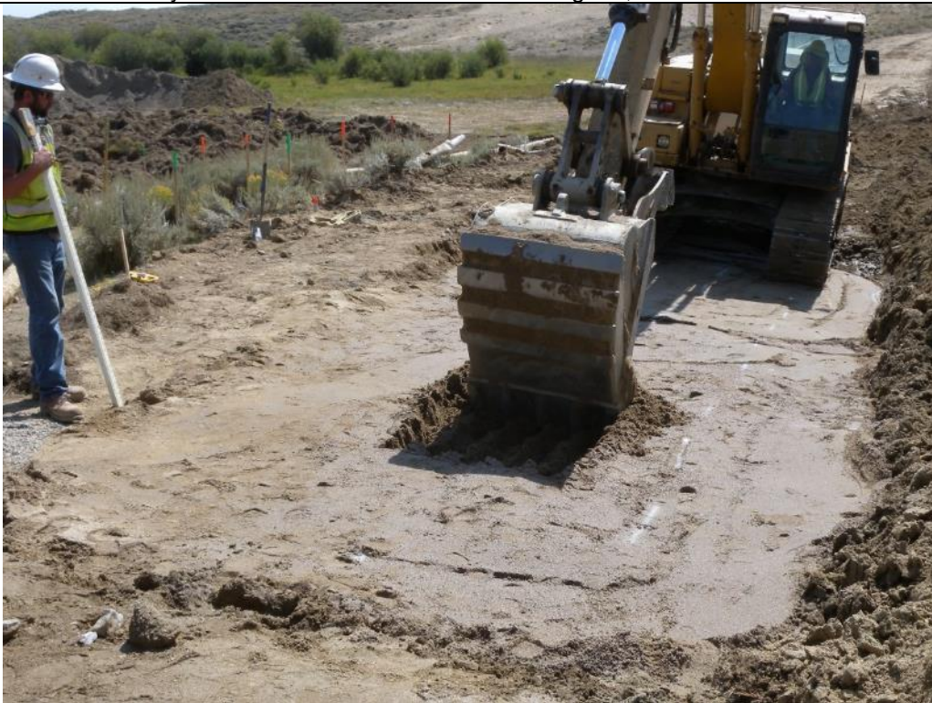
Photo 26. View looking right from MTD Sta. 2+45 at the compacted Type A Filter Sand and the start of the excavation for the Type B Gravel Drain for the chimney drain. Aug. 29, 2017.
