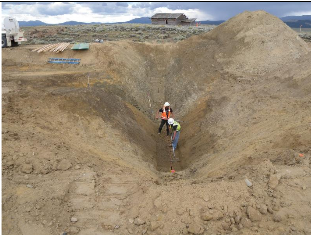
Photo 13. View looking right at the foundation preparation of the upstream cutoff spillway at ES Sta. 2+20. Aug. 14, 2017.
