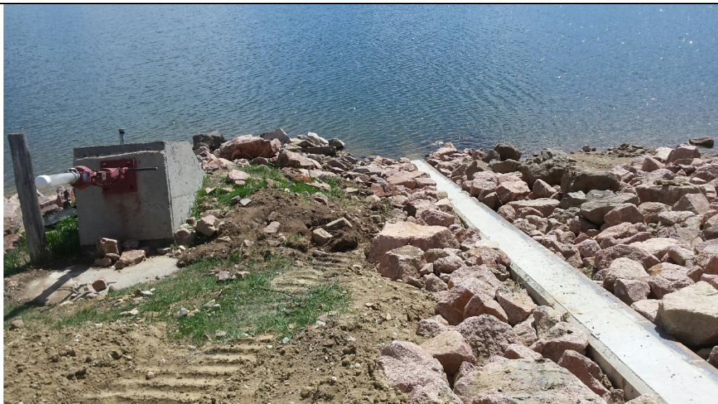
Photo 124. View of the air vent grade beam and staff gage. Note the riprap that was installed on both sides of the grade beam and the slope between the operator and grade beam was better graded. May 22, 2018.
