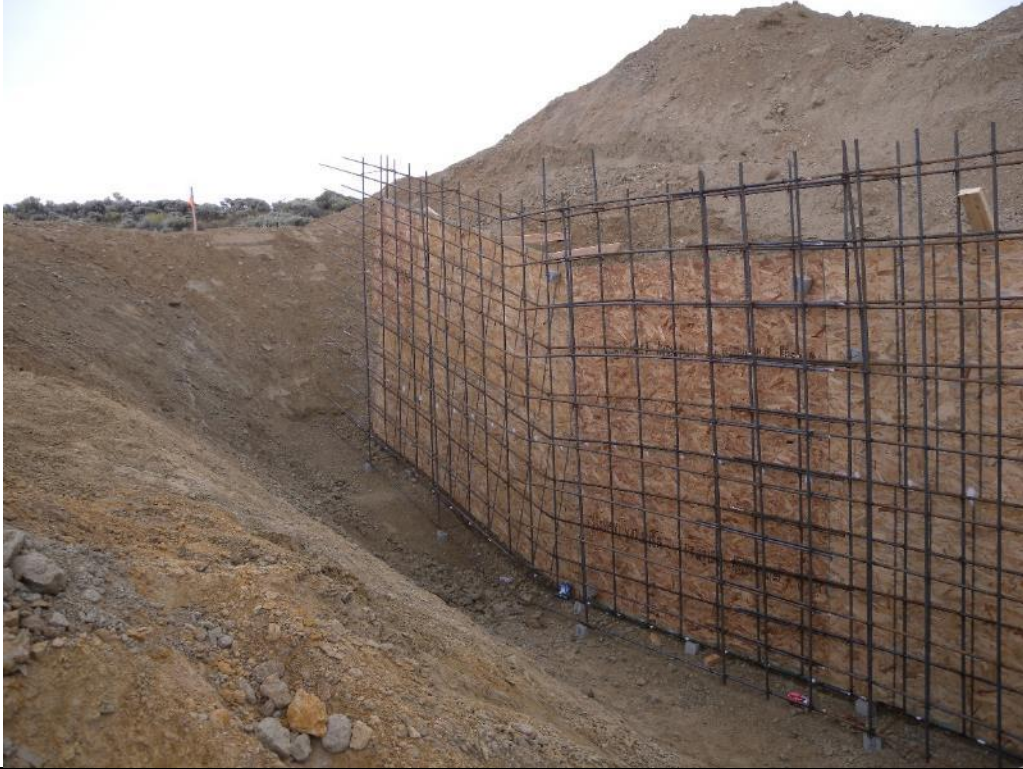
Photo 17. View of the formwork and rebar installation for the upstream spillway cutoff wall at ES Sta. 2+20. Aug. 16, 2017.
