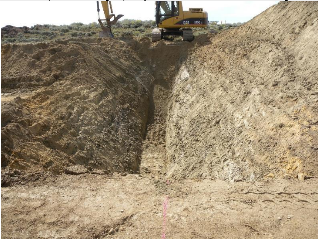
Photo 12. View looking right of the excavated foundation for the upstream spillway cutoff wall at ES Sta. 2+20. Aug. 14, 2017
