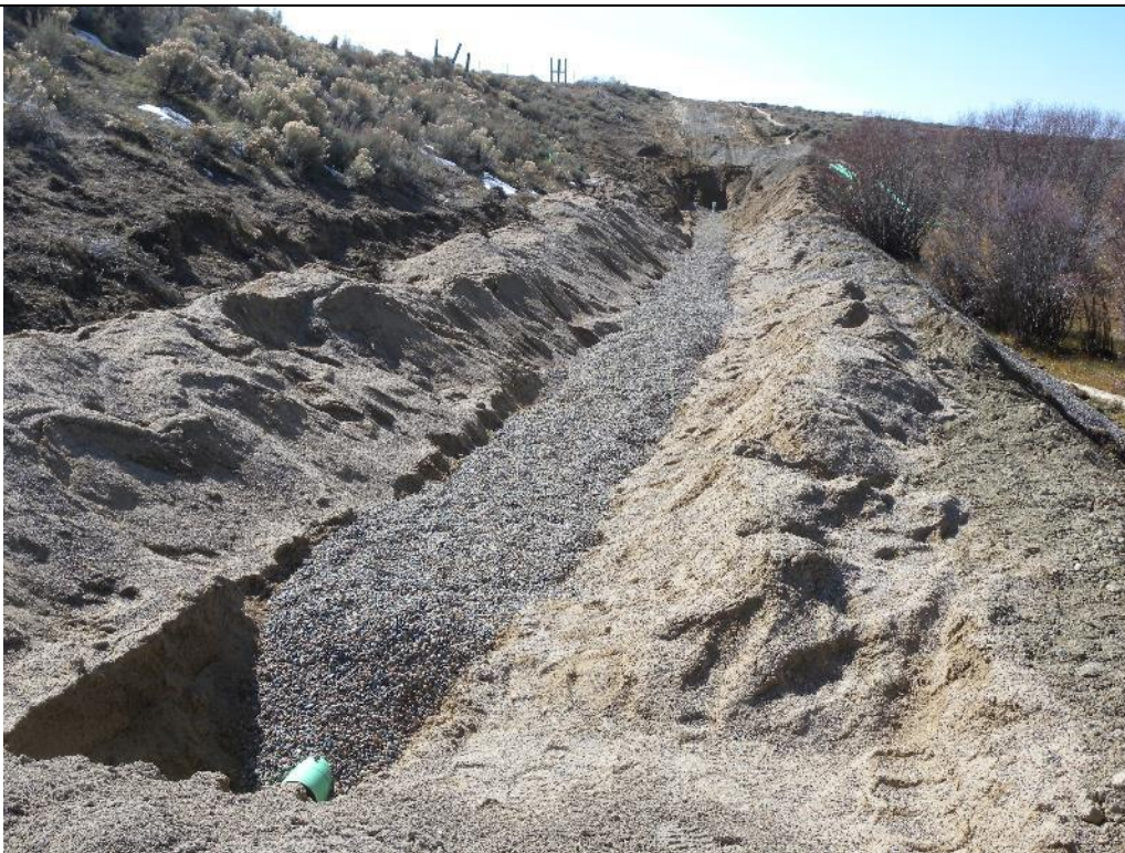
Photo 72. View looking left from NTD Sta. 1+85 at the installation of the slotted drain pipe and toe drain cleanout for the left side of the North Dam seepage collection system. Oct. 13, 2017.
