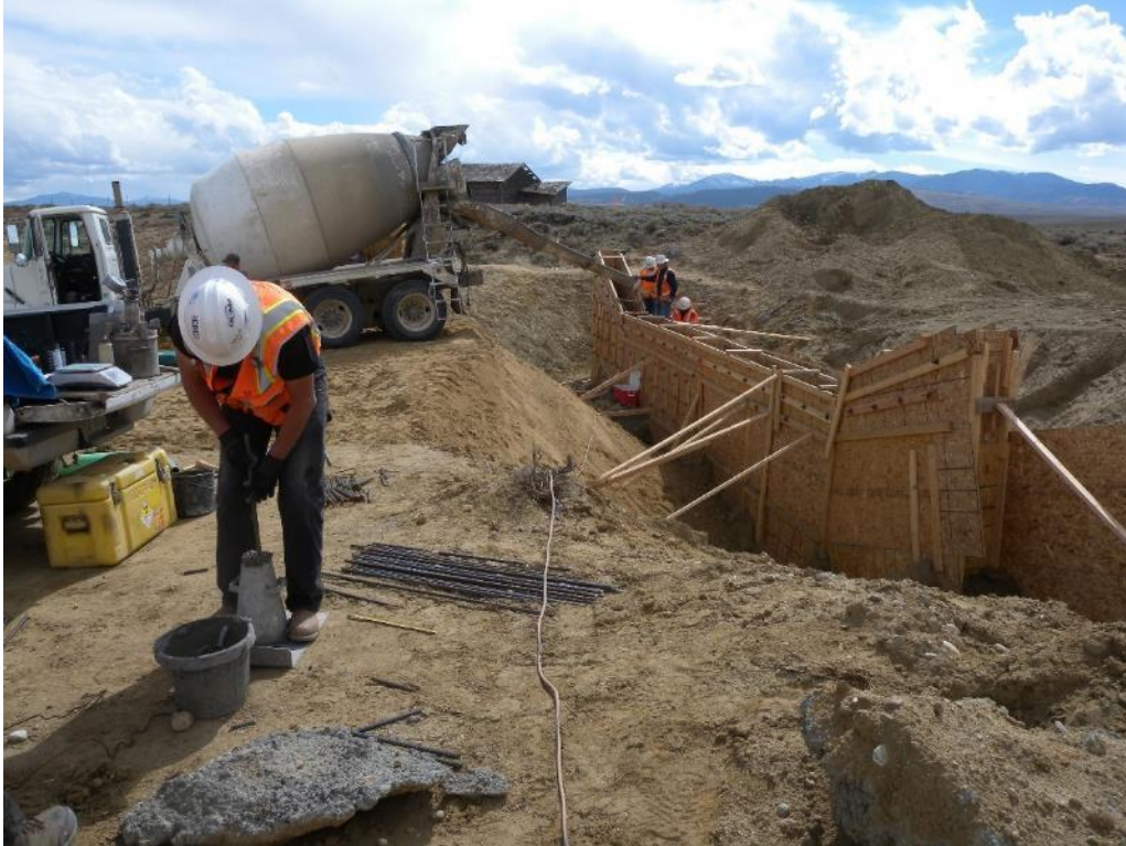
Photo 63. View of the concrete placement and concrete testing for the upstream spillway cutoff wall located at ES Sta. 2+20. Sept. 27, 2017
