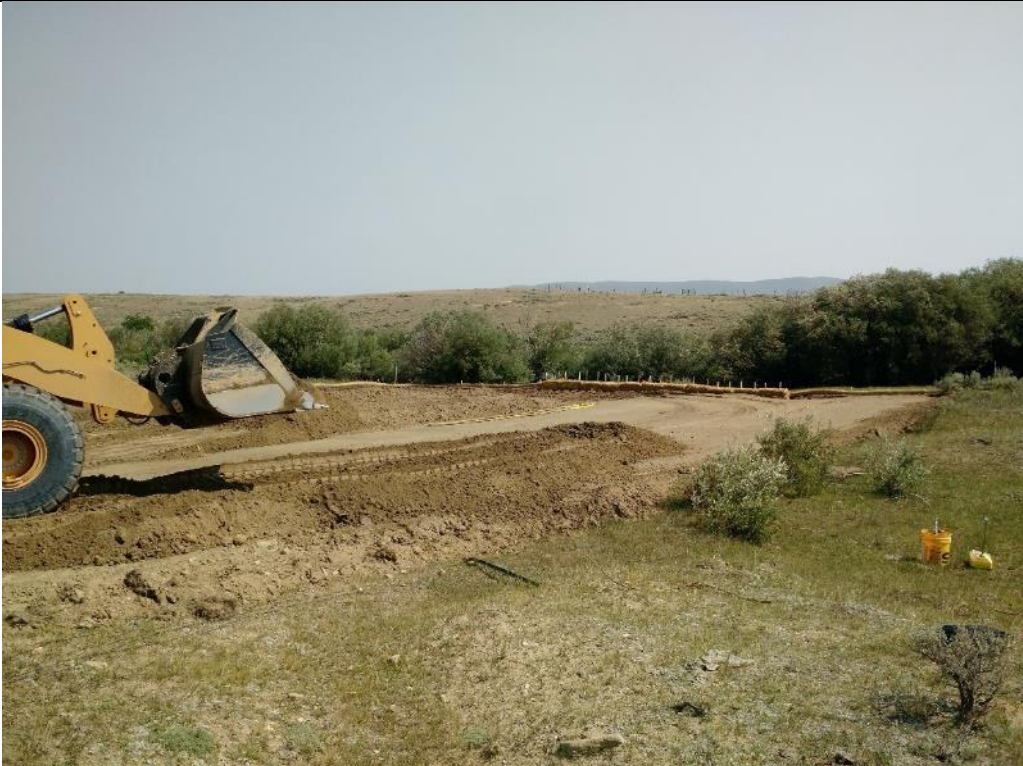
Photo 6. Placement of Embankment Fill for the first lift of the right spillway berm between ES Stations 5+50 and 6+50. Aug. 4, 2017.
