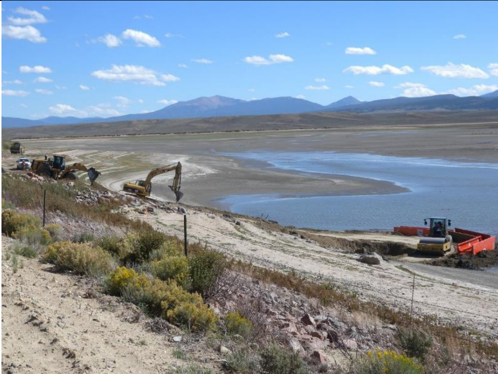
Photo 52. View looking upstream from Sta. 10+50 at the trench boxes and work on the coffer dam as well as construction of the temporary access road and platforms for the dewatering pumps on the upstream side of the reservoir. Sept. 20, 2017.
