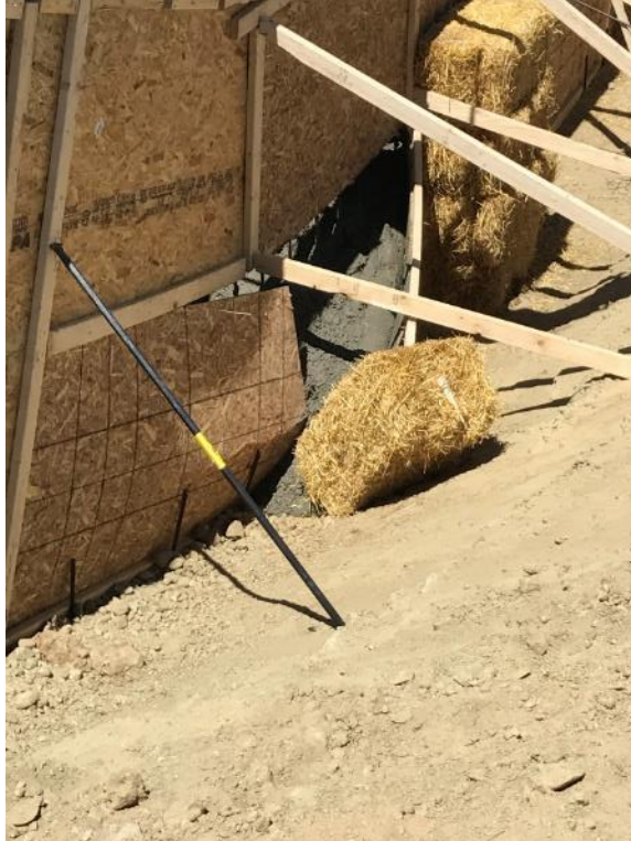
Photo 19. View looking at the form work blowout on the downstream side of the upstream spillway cutoff wall at ES Sta. 2+20. Aug. 18, 2017.
