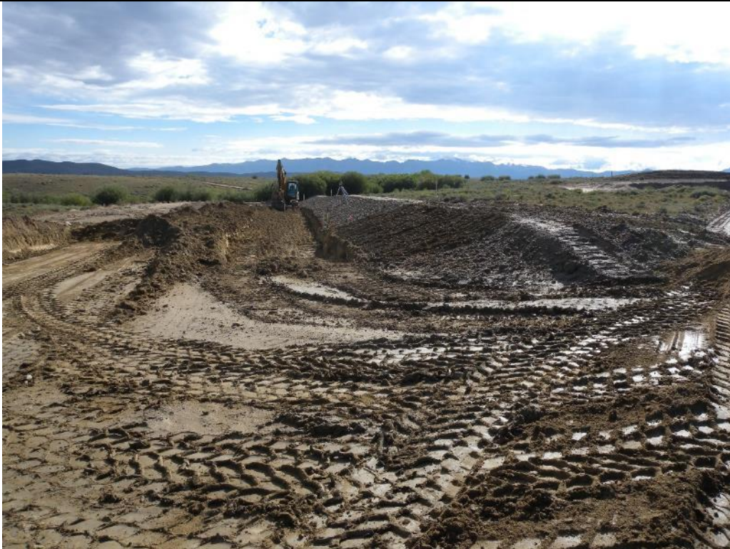
Photo 9. View from ES Sta. 3+00 looking downstream along the right spillway berm toe of RME shaping the right spillway berm. Aug. 10, 2017.
