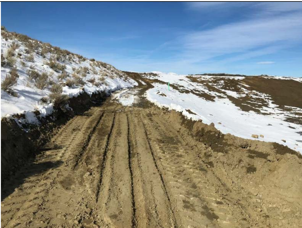
Photo 116. View looking left from Station 2+00 MTD of the final lift of Embankment Fill on the Main Dam Stability Berm. Nov. 9, 2017.
