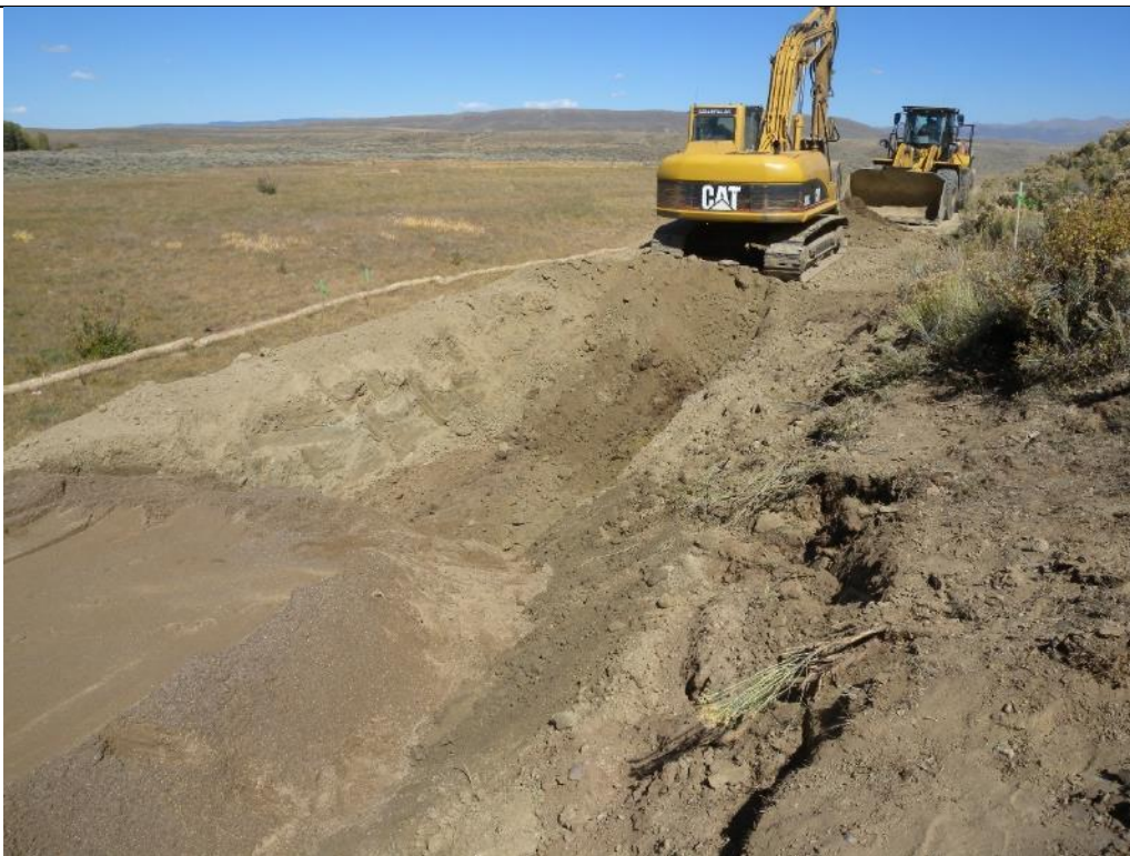
Photo 56. View looking right and downstream at NTD Sta. 1+50 to 1+75 at the excavation into the stability berm and construction of the Type A Filter Sand layer of the seepage collection system. Sept. 21, 2017.
