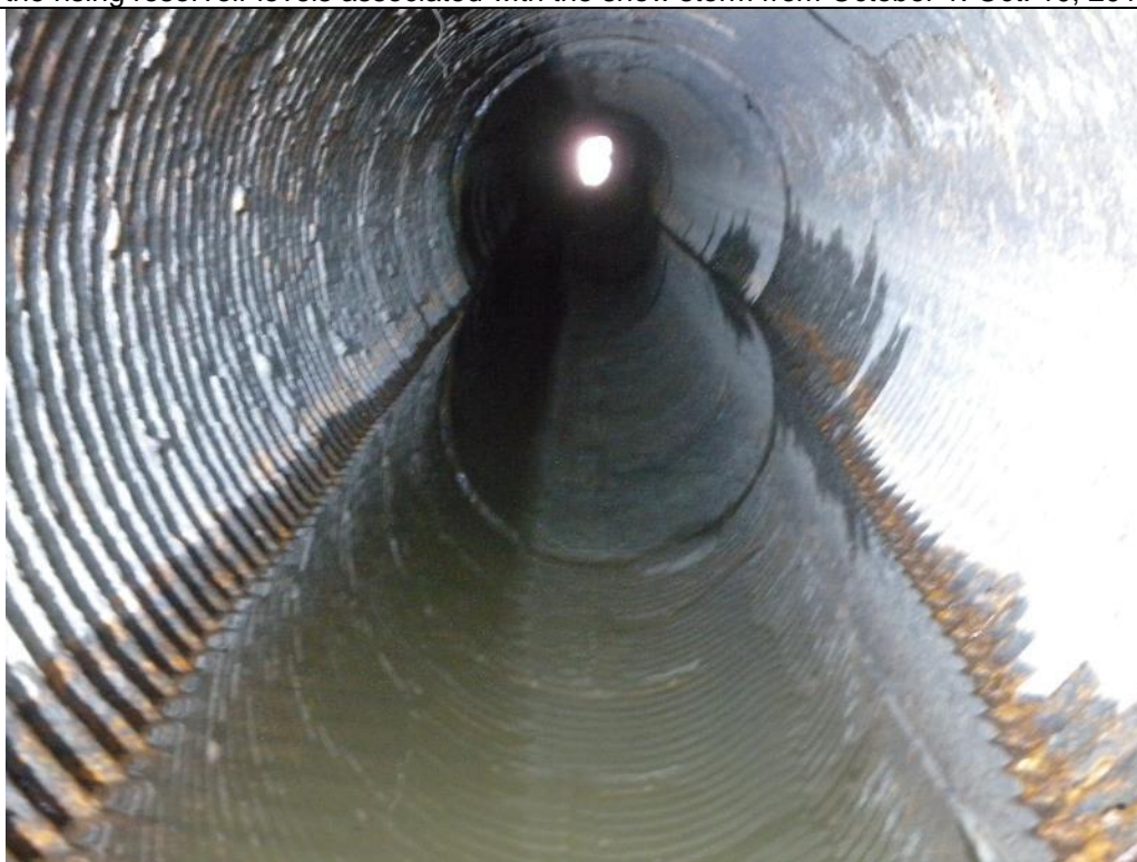
Photo 69. View looking upstream from the downstream end of the outlet works conduit at ponded water in the conduit due to overtopping of the coffer dam. The approximate depth of water was in excess of 4 inches in some areas. Oct. 10, 2017.
