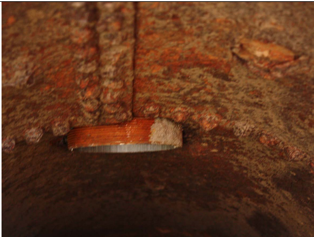
Photo 84. Close-up view of the Air Vent Pipe which was inserted into the original riveted steel outlet works conduit. Oct. 23, 2017.
