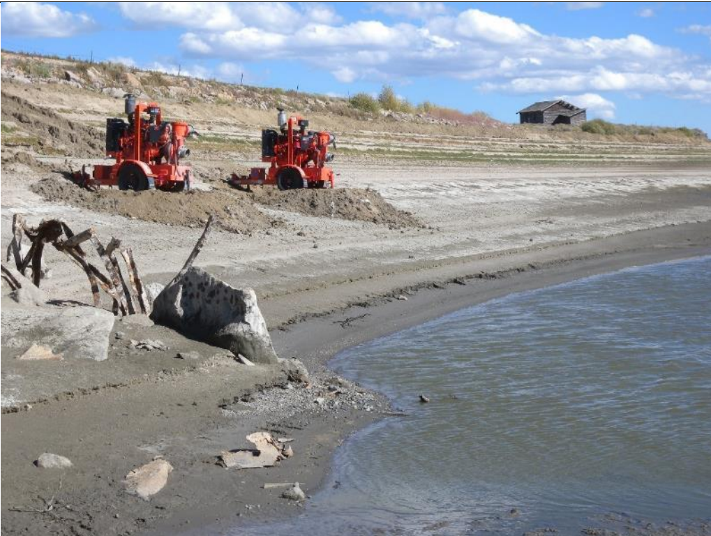
Photo 54. View looking right from the top of the coffer dam at the two reservoir dewatering pumps placed on the upstream side of the Main Dam Embankment near Sta. 11+00. Sept. 20, 2017.
