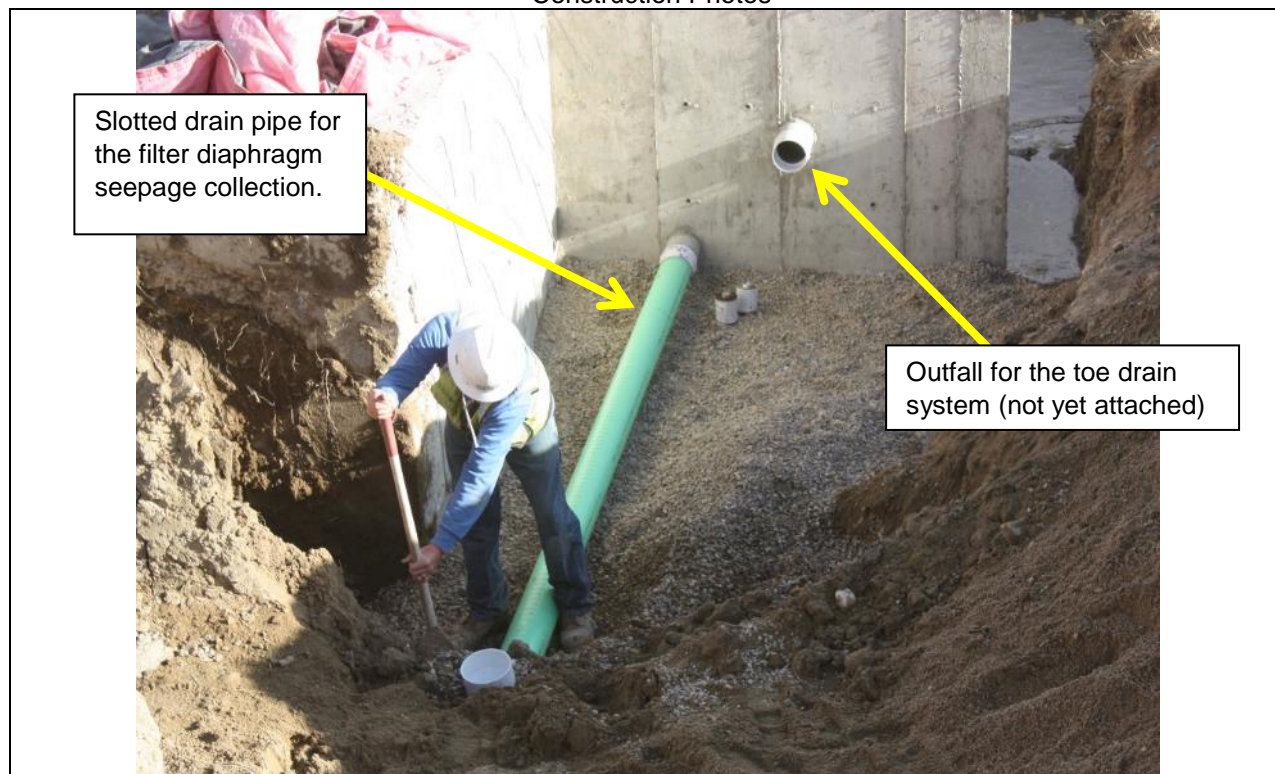
Photo 102. View looking downstream at the right side of the outlet works terminal structure headwall. The filter diaphragm slotted drain pipe was being installed and buried by Type B Gravel Drain. Nov. 2, 2017.
