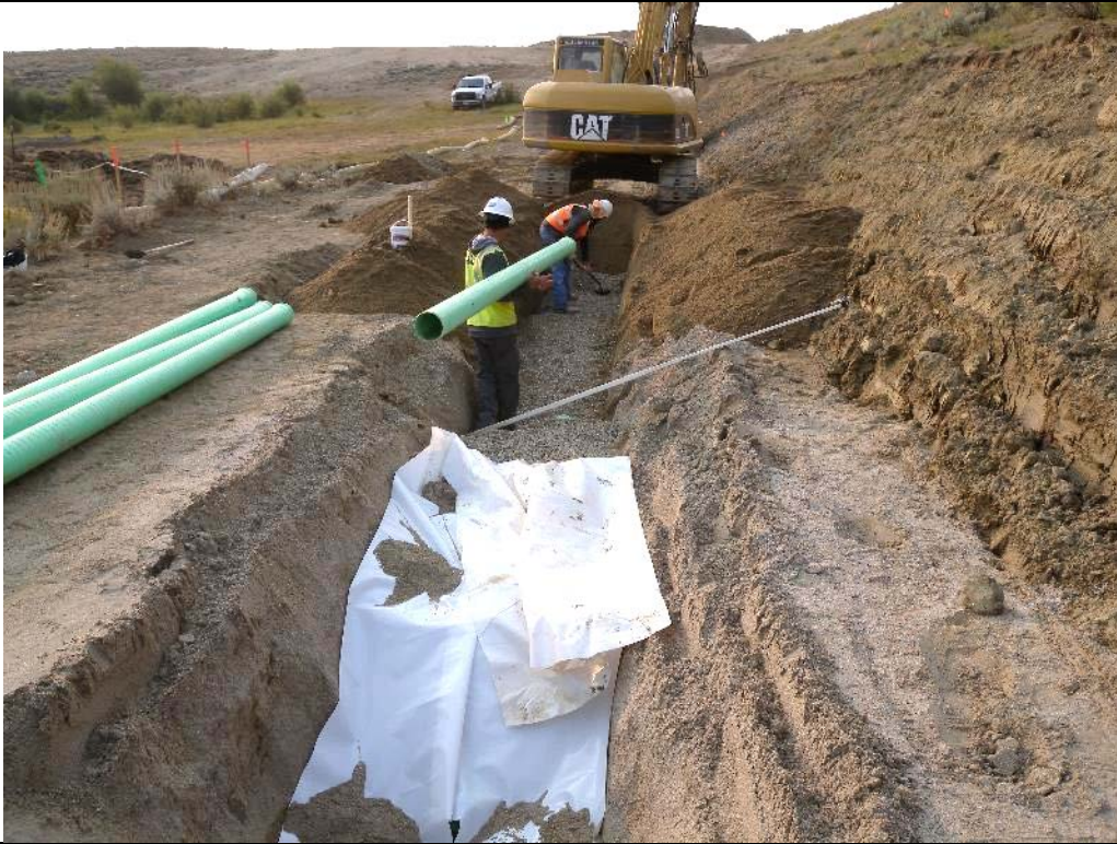
Photo 33. View looking right from MTD Sta. 2+50 at the start of placement of the slotted drain pipe. The excavator was used to dig into the compacted layer of Type A Filter Sand, Type B Gravel Drain was placed at the bottom of the excavation to the invert of the slotted drain pipe and the drain pipe was then added and buried with 1-foot of Type B Gravel Drain. Sept. 7, 2017.
