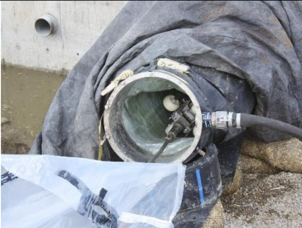
Photo 98. View looking upstream from the downstream end of the outlet works conduit at the roller device which houses the UV lamps and was now inserted into the partially inflated, downstream end of the pipe. Nov. 1, 2017.
