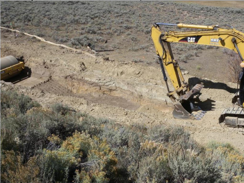
Photo 50. View of the excavation of the stability berm and installation and compaction of the Type A Filter Sand in the North Dam chimney drain near NTD Sta. 0+00 to 0+80. Sept. 19, 2017.
