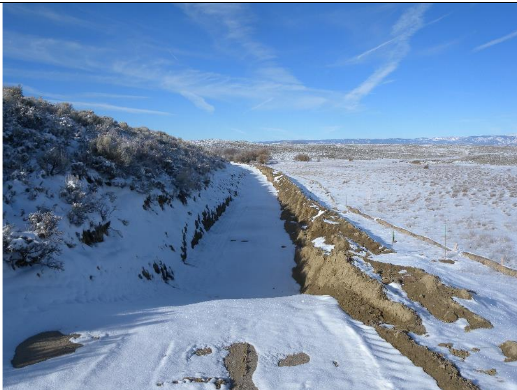
Photo 70. View looking left at the North Embankment seepage collection system from NTD Sta. -0+10. Snow is currently covering the top layer of Type A Filter Sand. Oct. 10, 2017.
