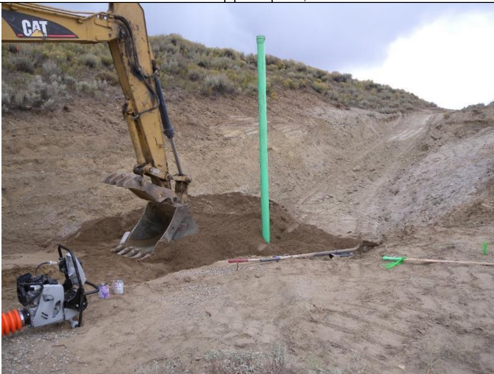
Photo 46. View from MTD Sta. 0+60 looking upstream at toe drain cleanout and placement of the Type A Filter Sand around the cleanout riser pipe. Sept. 14, 2017.
