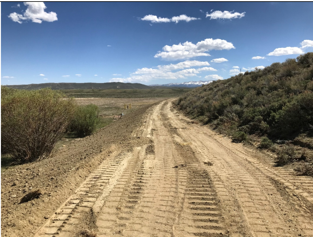
Photo 120. View looking right across the completed North Dam stability berm prior to reseeding. May. 17, 2018.
