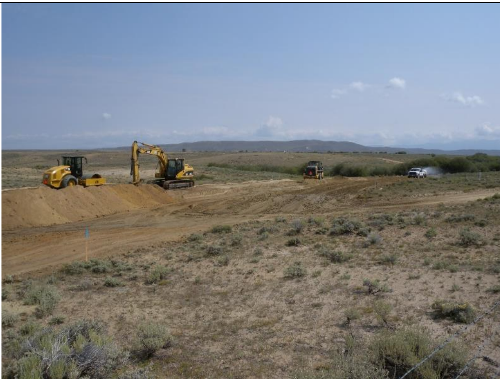
Photo 7. View looking downstream from ES Sta. 2+00 of soil placement and moisture conditioning on the left and right spillway berms. Aug. 7, 2017.
