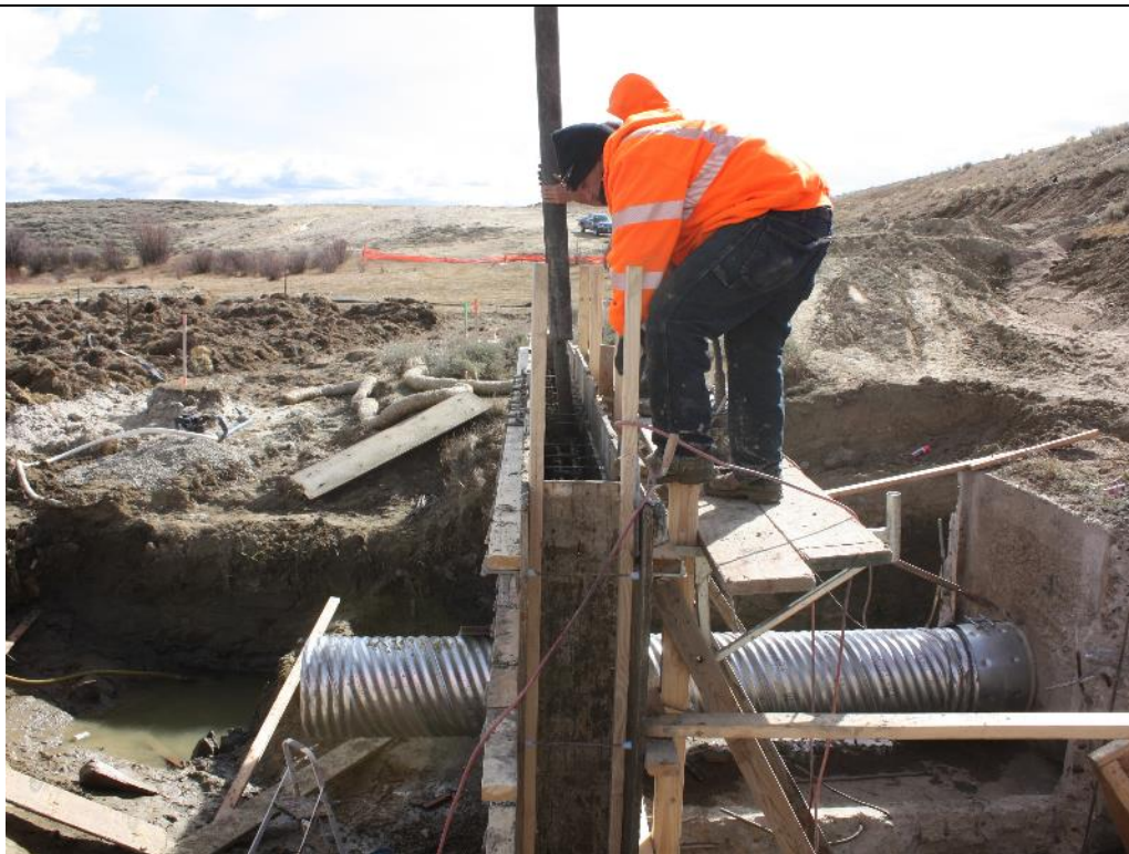
Photo 82. View looking right from the left side of the new outlet works terminal structure headwall at the concrete being placed from the pump truck. Oct. 23, 2017.
