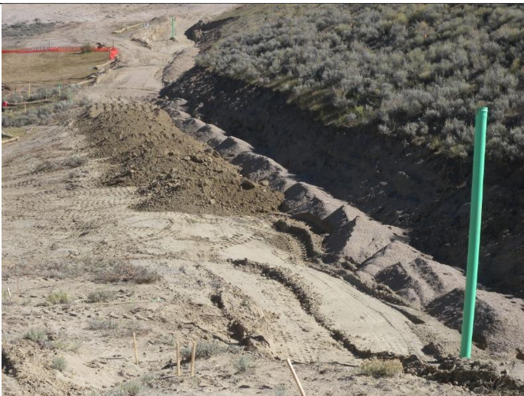
Photo 55. View looking right from approximate MTD Sta 0+00 at the Work in progress on the Main Dam which included placement of the chimney drain and lifts of Embankment Fill from MTD Sta 0+50 to 2+00. Sept 21, 2017.
