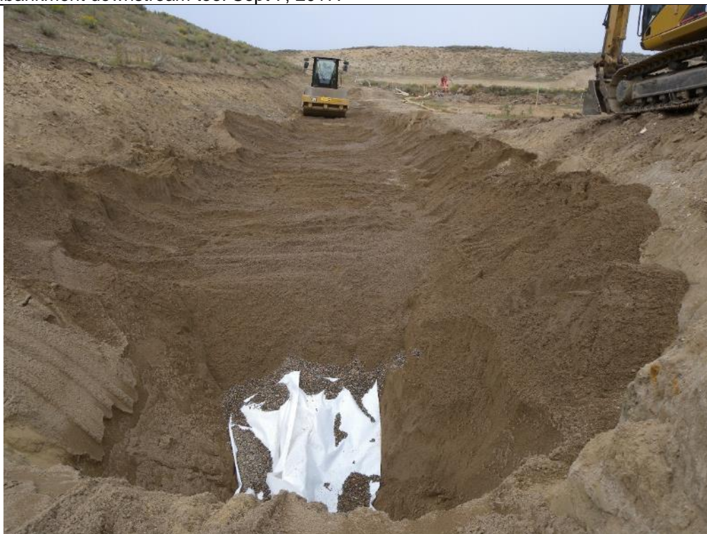
Photo 36. View looking left from approximate MTD Sta. 5+15 at the plastic cover over the location of where the Main Dam, Right Toe Drain clean-out will be located, and the compaction of a lift of Type A Filter Sand. Sept. 8, 2017.
