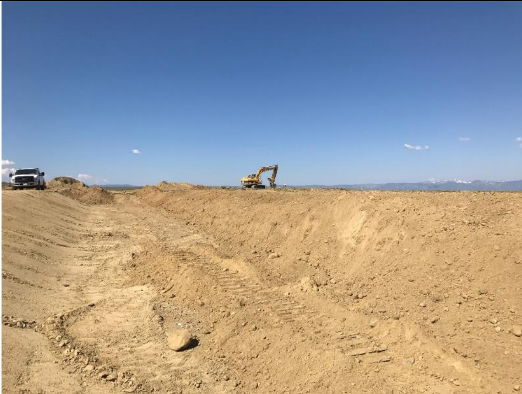
Photo 21. View looking upstream of the left spillway berm shaping and grading from ES Station 5+50. Aug. 22, 2017.
