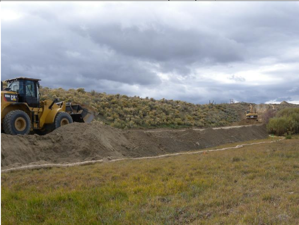
Photo 48. View looking left and upstream at the base of the North Embankment Stability Berm which was first constructed as shown above so the seepage collection system could then be constructed within the base of the berm. Shown above is the start of the excavation at NTD Sta. 0+00 and hauling of Type A Filter Sand for the placement of the seepage collection system Sept. 15, 2017.
