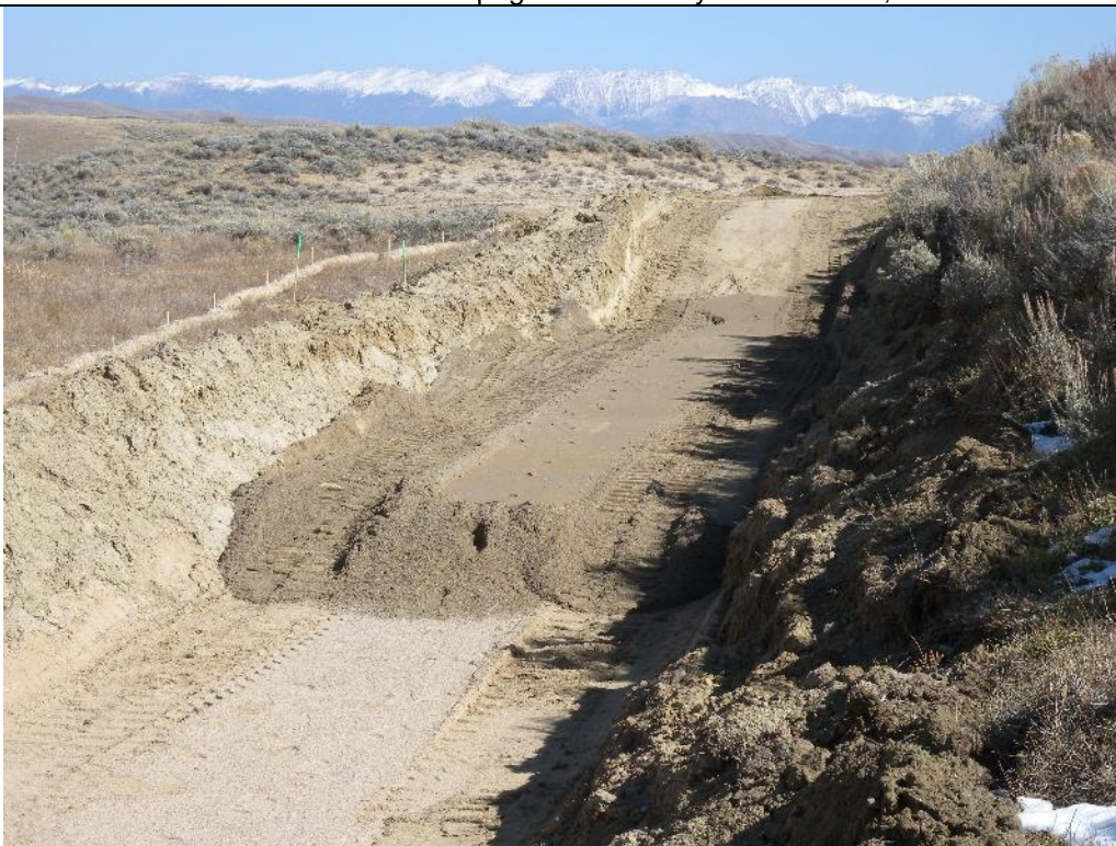
Photo 73. View looking right from approximate NTD Sta. 4+25 at the short lift of Type A Filter Sand placed from approximate NTD Sta. 4+50 to 5+10. Oct. 13, 2017.
