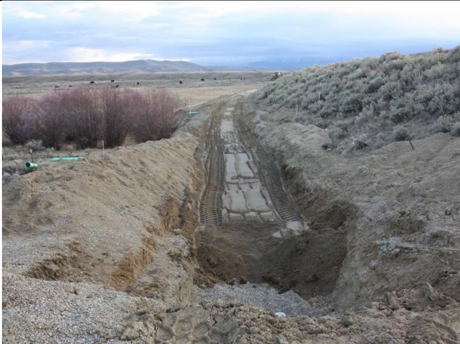
Photo 101. View looking right from NTD Sta. -0+15 at the Type A Filter Sand which is at the top of the toe drain elevation and ready to be covered with Embankment Fill. Nov. 2, 2017.
