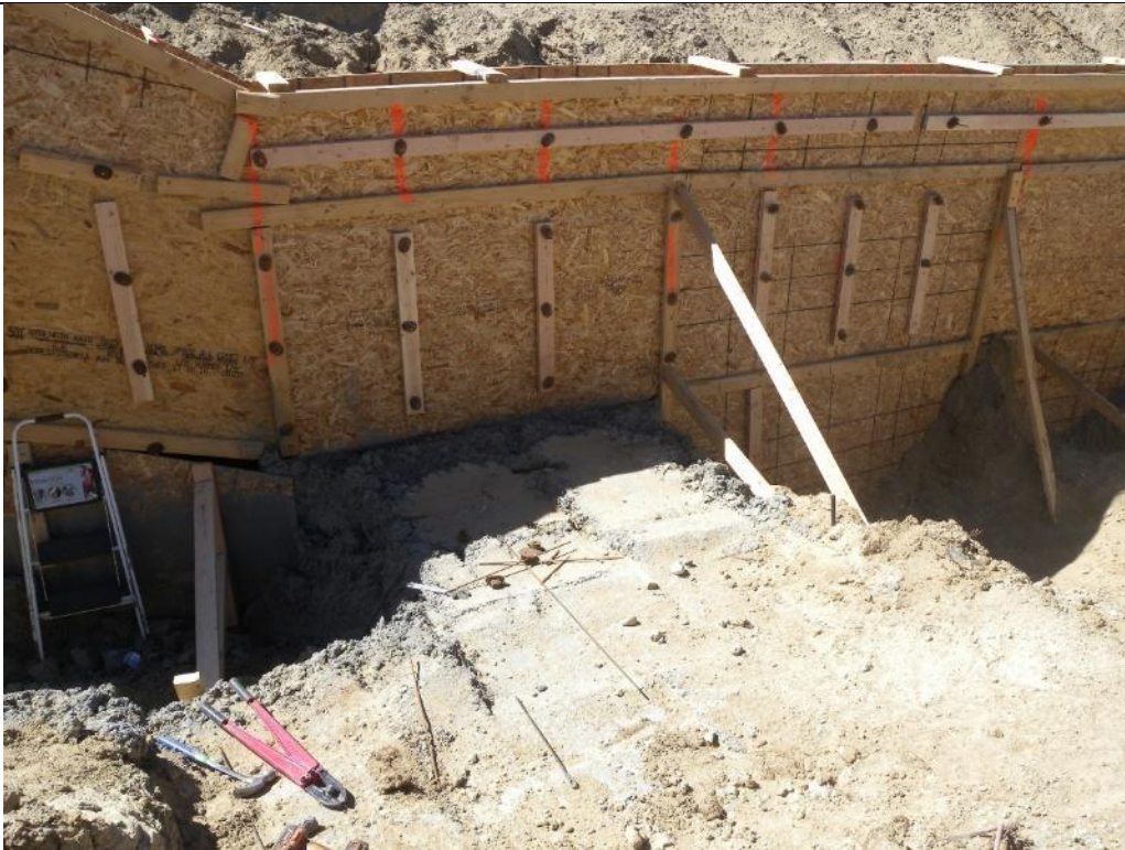
Photo 57. Representative view of the work completed by the concrete crew who added form ties and additional support to the upstream spillway cutoff wall at ES Sta. 2+20. Sept. 22, 2017.
