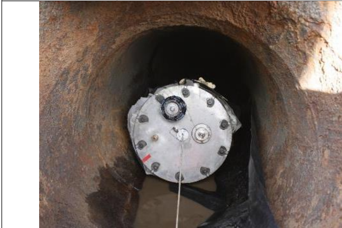
Photo 97. View looking downstream from the upstream inlet at the sealed upstream start of the CIPP liner. Nov. 1, 2017.
