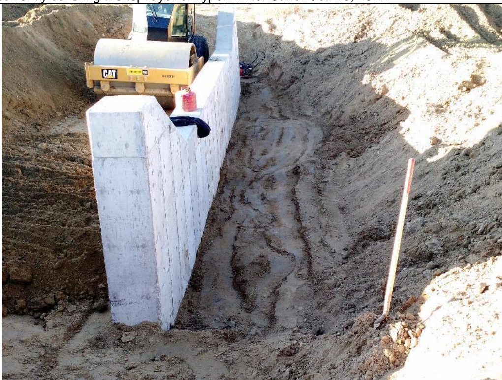
Photo 71. View looking left at upstream side of the downstream Spillway cutoff wall. RME used the roller to compact the majority of the lift and the Jumping Jack to compact along the cutoff wall. Oct. 11, 2017.
