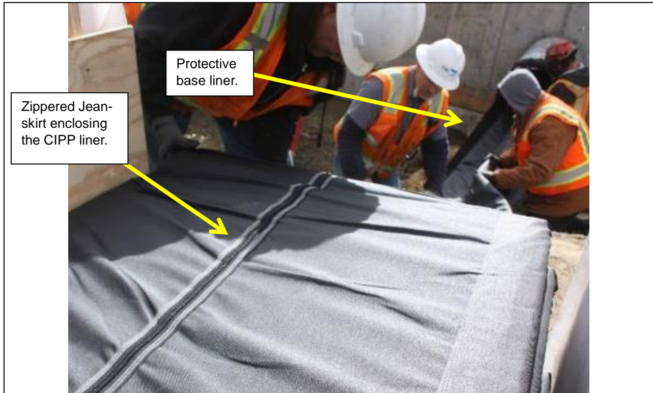
Photo 96. View looking at the CIPP liner being installed from the downstream end of the outlet works conduit. Note, a jean-skirt surrounds the CIPP liner for UV protection and to prevent over-expansion of the CIPP liner during inflation which was required for the upstream inlet transition section from 24 inches to 36 inches in diameter. Nov. 1, 2017.
