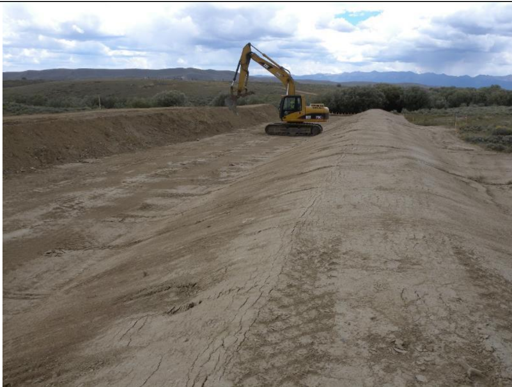
Photo 14. View looking downstream from ES Sta. 4+00 at the shaped and compacted right spillway berm and spillway discharge channel prior to excavation of the downstream cutoff wall at ES Sta. 5+20.
