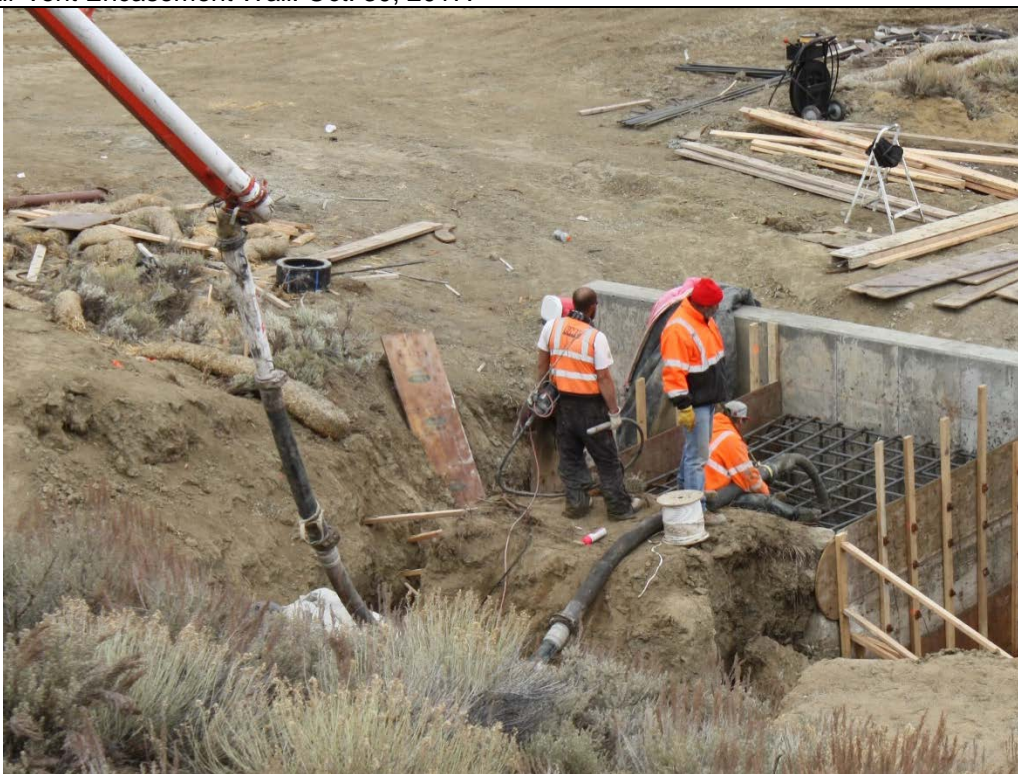
Photo 91. View looking downstream at the placement of concrete by the pump truck into the CMP outlet works conduit extension encasement section. Oct. 30, 2017.
