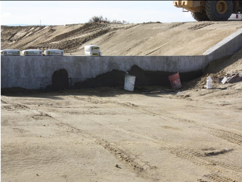
Photo 92. View looking upstream at the downstream side of the upstream spillway cutoff wall where RME patched the concrete from the initial partial concrete pour. Oct. 31, 2017.
