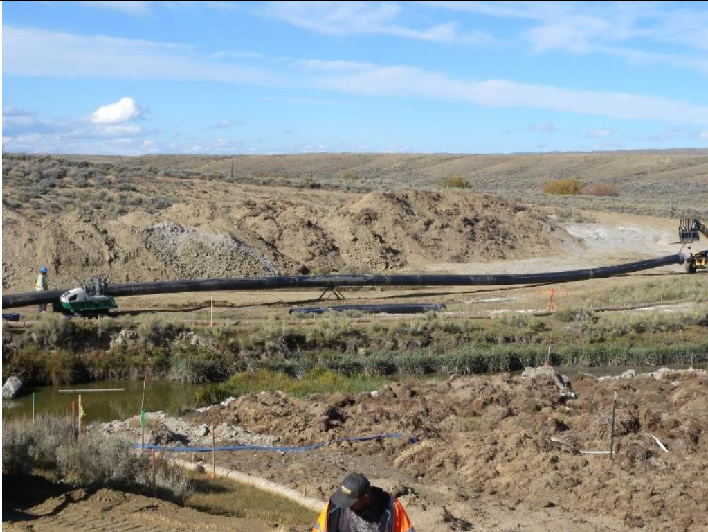
Photo 62. View of C&L fusing the 20-inch-diameter HDPE pipe. Sept. 26, 2017
