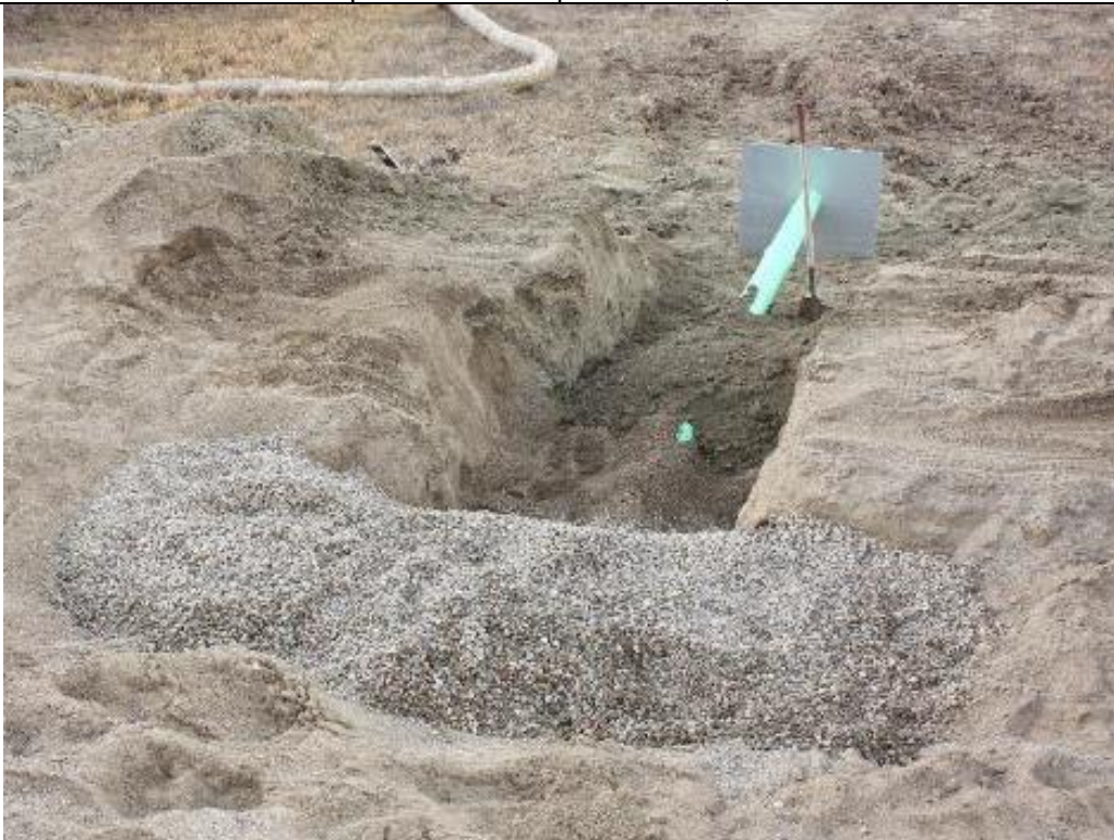
Photo 93. View looking downstream from NTD Sta. 1+75 at the North Embankment Toe Drain Outfall after installation of the discharge pipe and steel plate. Nov. 1, 2017.
