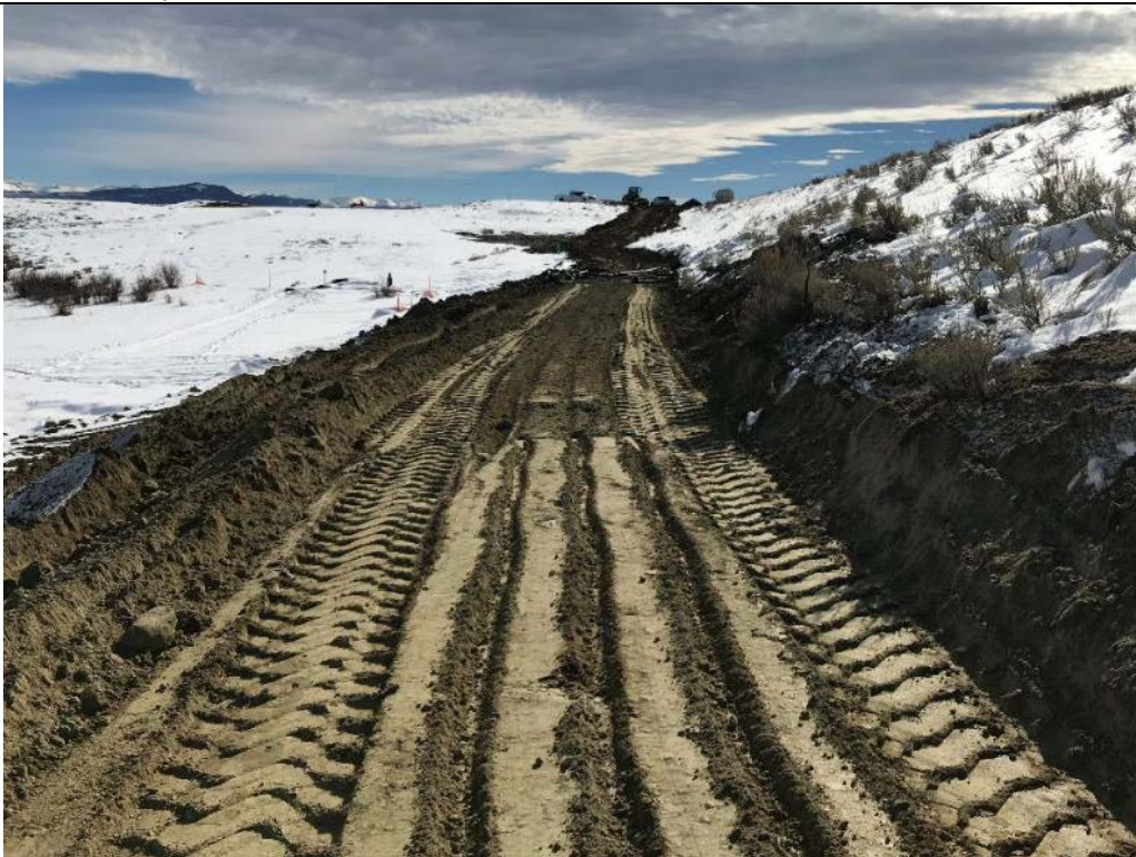
Photo 117. View looking right from Station 2+50 MTD of the final compacted Embankment Fill lift of the Main Dam Stability Berm. Nov. 9, 2017.
