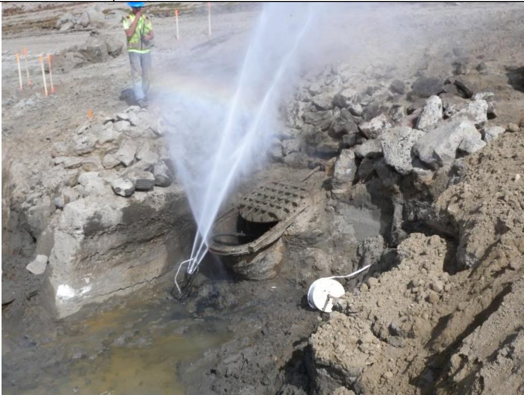
Photo 64. View of Snowbridge Inc. water jetting the outlet works conduit. Sept. 28, 2017
