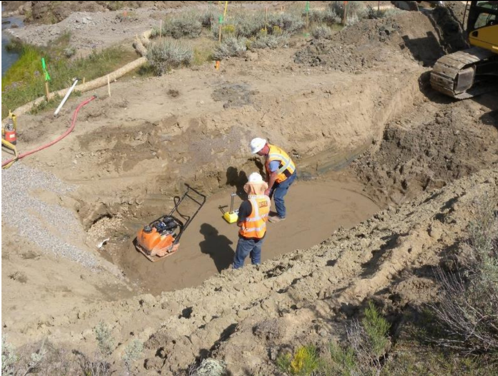
Photo 25. Representative view of the completed excavation and placement and compaction of Type A Filter Sand in the chimney drain at MTD Sta. 2+50 to 2+70. Aug. 28, 2017.
