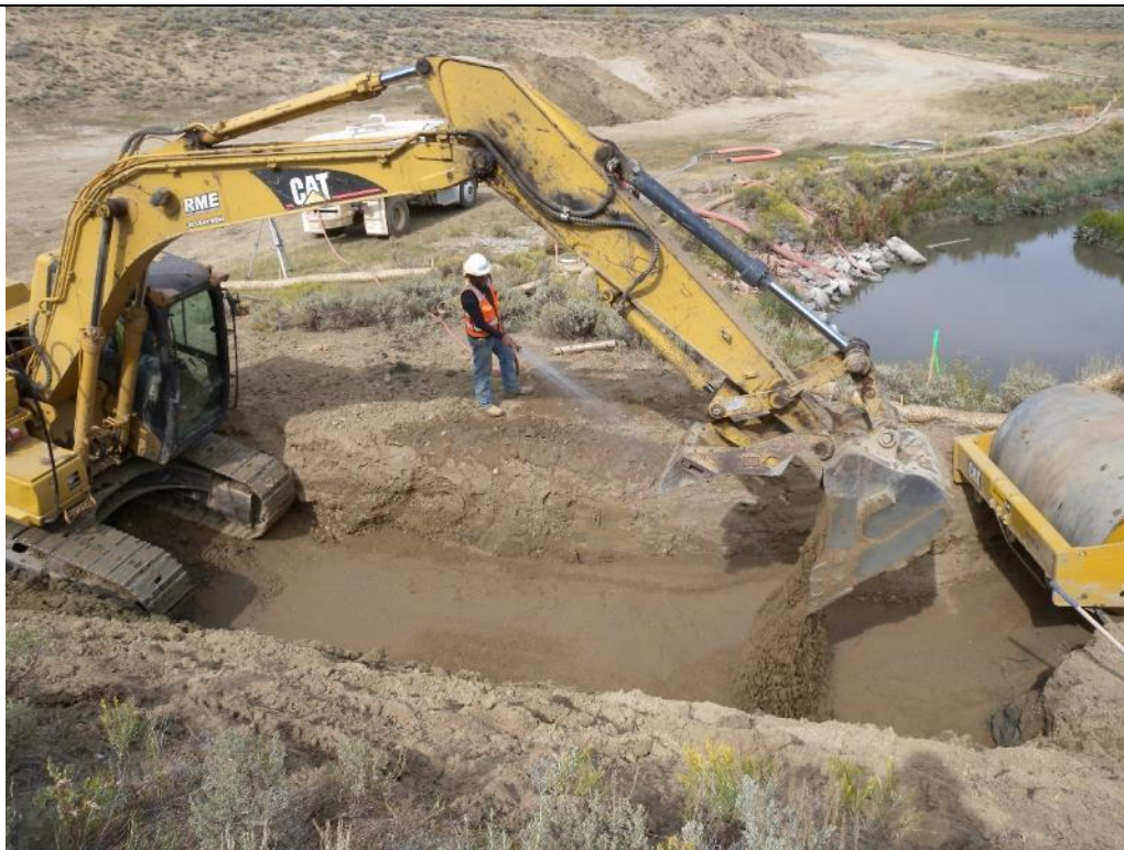
Photo 37. Looking downstream from approximate MTD Sta. 2+40 at the start of the seepage collection system for the left side of the Main Dam. Representative work included excavation into the toe of the Main Dam, removal of the old toe drain pipe, and placement, moisture conditioning and compaction of Type A Filter Sand shown above. Sept. 8, 2017.
