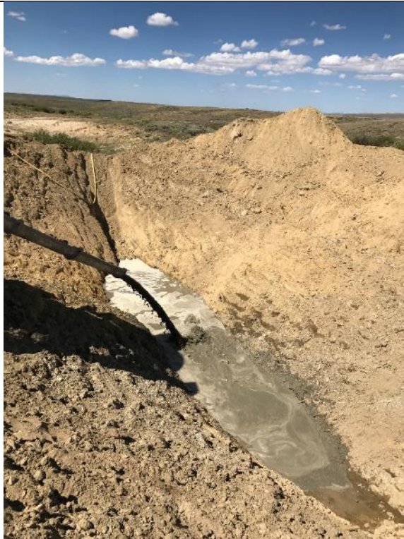
Photo 20. View looking left of the mud-mat placement in the foundation of the downstream spillway cutoff wall at ES Sta. 5+20. Aug. 18, 2017.
