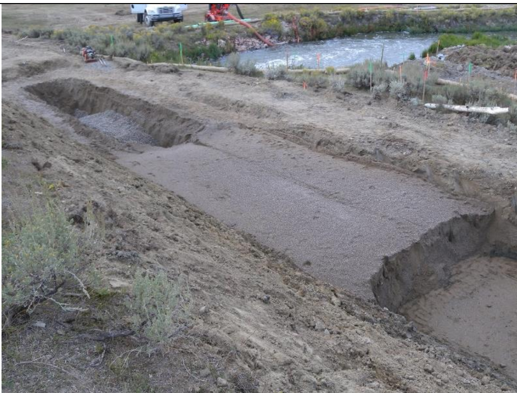
Photo 30. Representative view of the chimney drain installation work between MTD Sta. 2+55 and 3+20. Aug 29, 2017.
