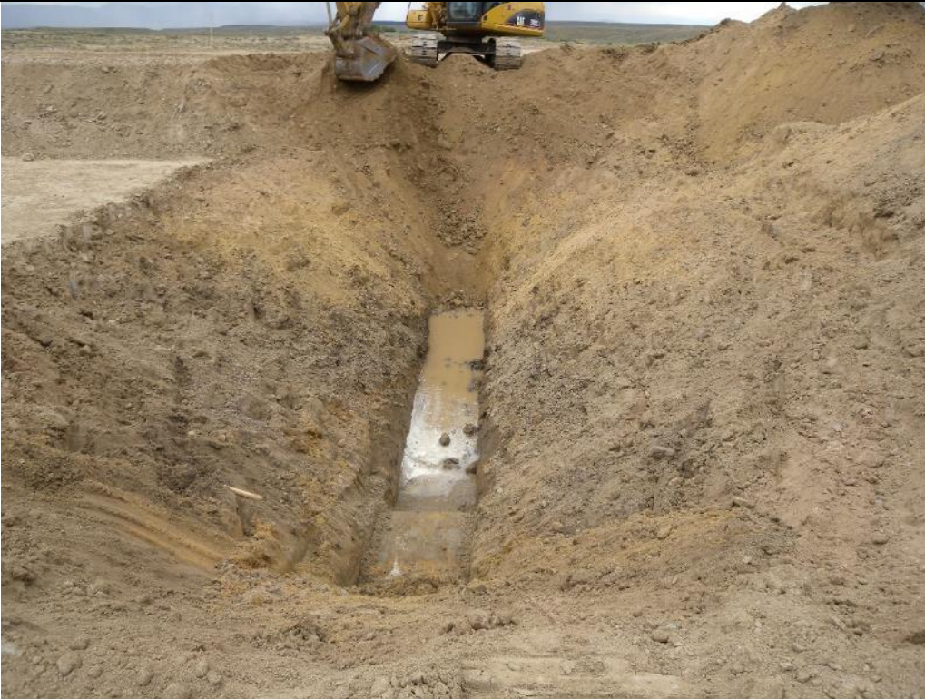
Photo 15. View looking left at the foundation excavation of the downstream spillway cutoff wall at ES Sta. 5+20. Note the seepage in the excavated foundation. Aug. 14, 2017
