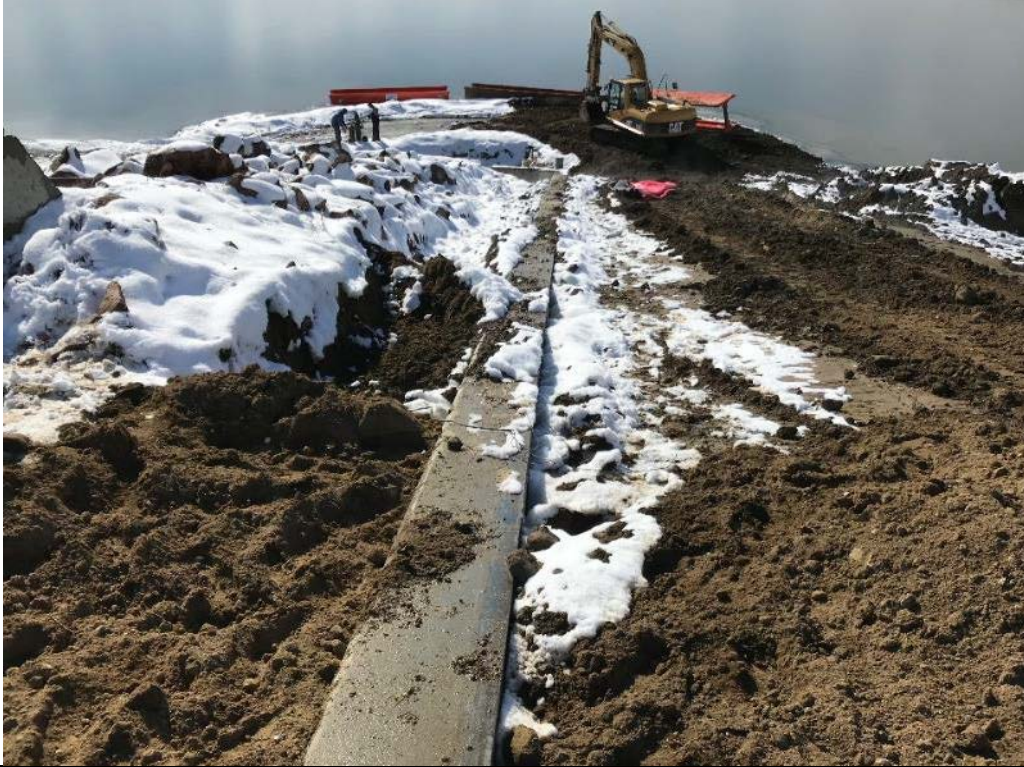
Photo 110. View looking down at the top of the air vent encasement wall containing the staff gage grade beam which had now been backfilled. RME completed the outlet works work and was preparing to start removing the cofferdam and begin re-filling the reservoir once permission to fill was granted by the Colorado Division of Water Resources. Nov. 7, 2017.
