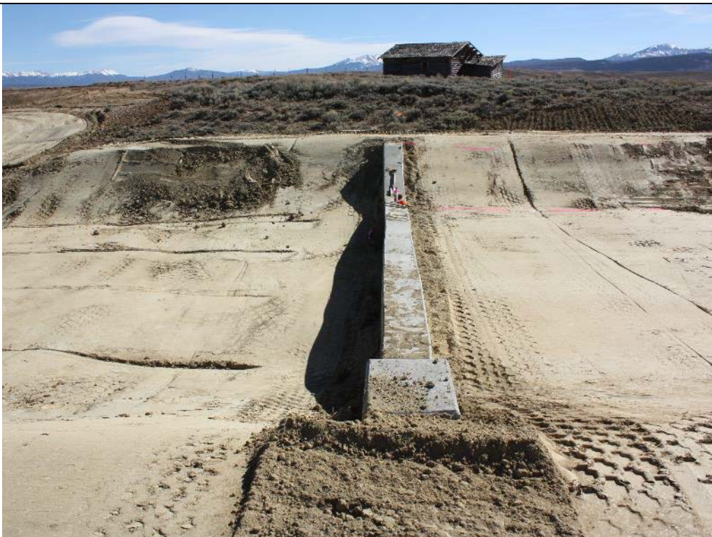
Photo 78. View looking right across the upstream spillway cutoff wall which has been backfilled. Oct. 17, 2017.
