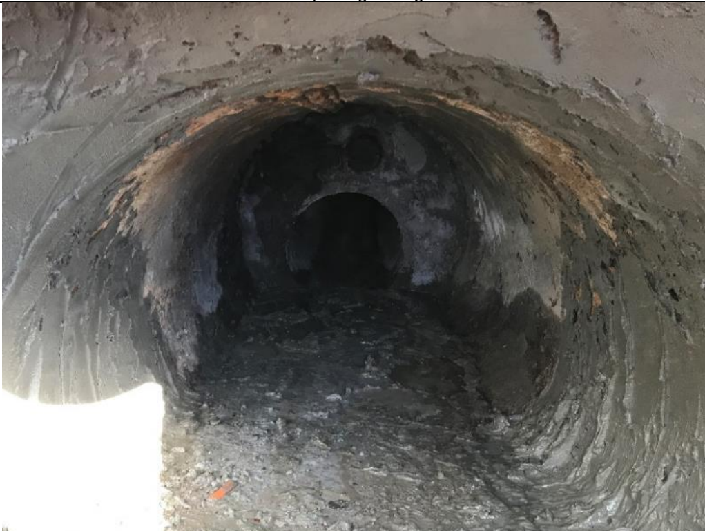
Photo 109. View looking downstream from the outlet conduit inlet gate at the non-shrink grout coating being installed in the invert and around the perimeter of the existing riveted steel outlet works pipe. Note, additional non-shrink grout was placed along the top of the existing riveted steel outlet works pipe after this picture was taken. Nov. 7, 2017.
