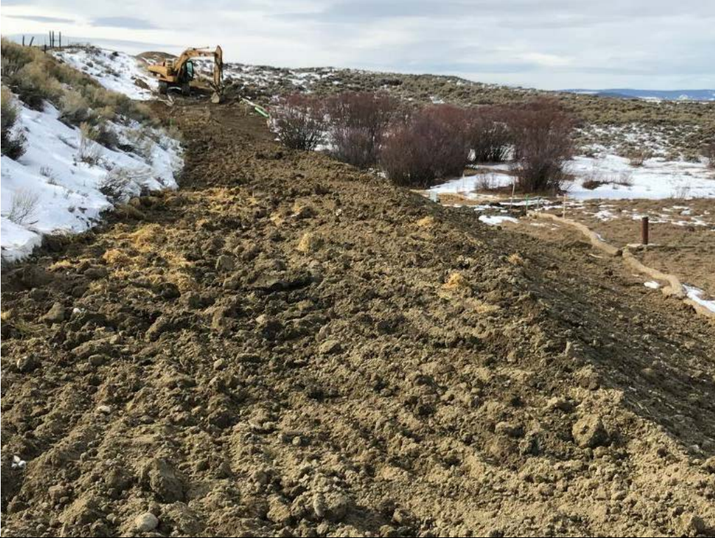
Photo 118. View looking left along the North Dam finished Stability Berm from approximate NTD Sta. 2+75 which has been shaped and scarified. Also shown is the downstream piezometer located to the right of the toe drain discharge outfall. Nov. 14, 2017.
