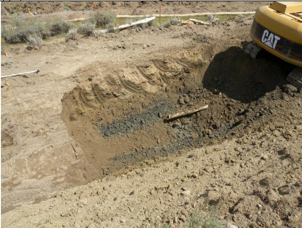
Photo 28. View looking downstream at the exposed, previous seepage collection system at approximate MTD Sta. 2+90. This pipe was removed during excavation of the chimney drain. Aug. 29, 2017.
