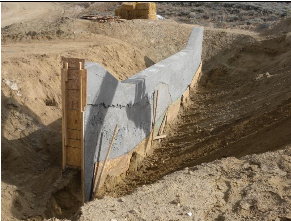
Photo 65. View looking at the upstream side of the upstream concrete cutoff wall after the forms were stripped. September 28, 2017.
