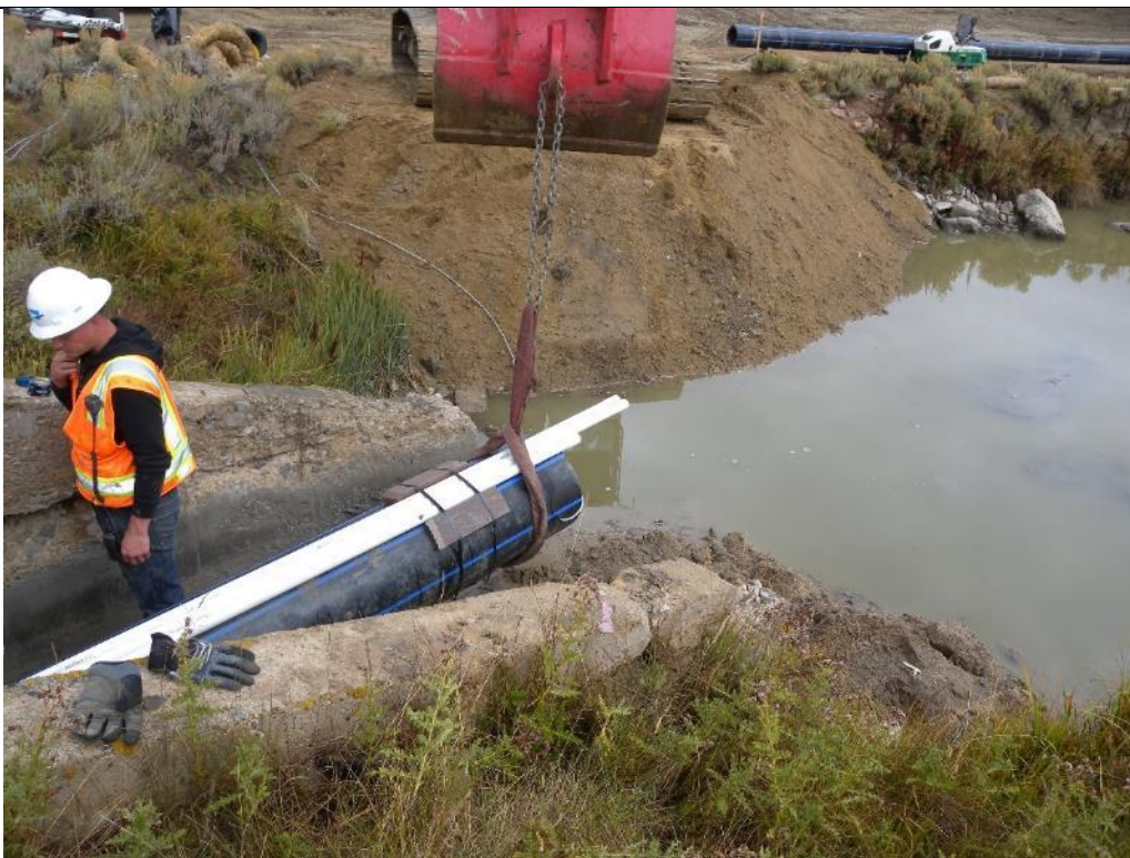
Photo 66. View of the 20-foot-long test section of HDPE pipe during the test pull which became stuck approximately 10-feet into the host pipe. Sept. 29, 2017.
