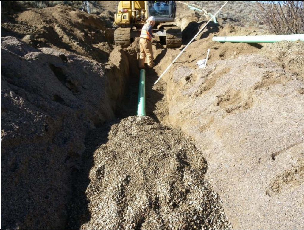
Photo 59. View looking left from NTD Sta. 0+80 at the installation of the slotted drain pipe and Type B Gravel Drain. Sept. 25, 2017.
