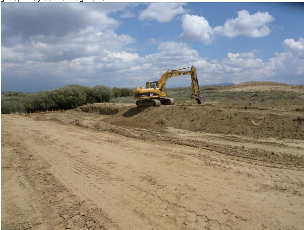
Photo 8. View from ES Sta. 5+00 looking right at the right spillway berm being shaped using the excavator. Aug. 9, 2017.
