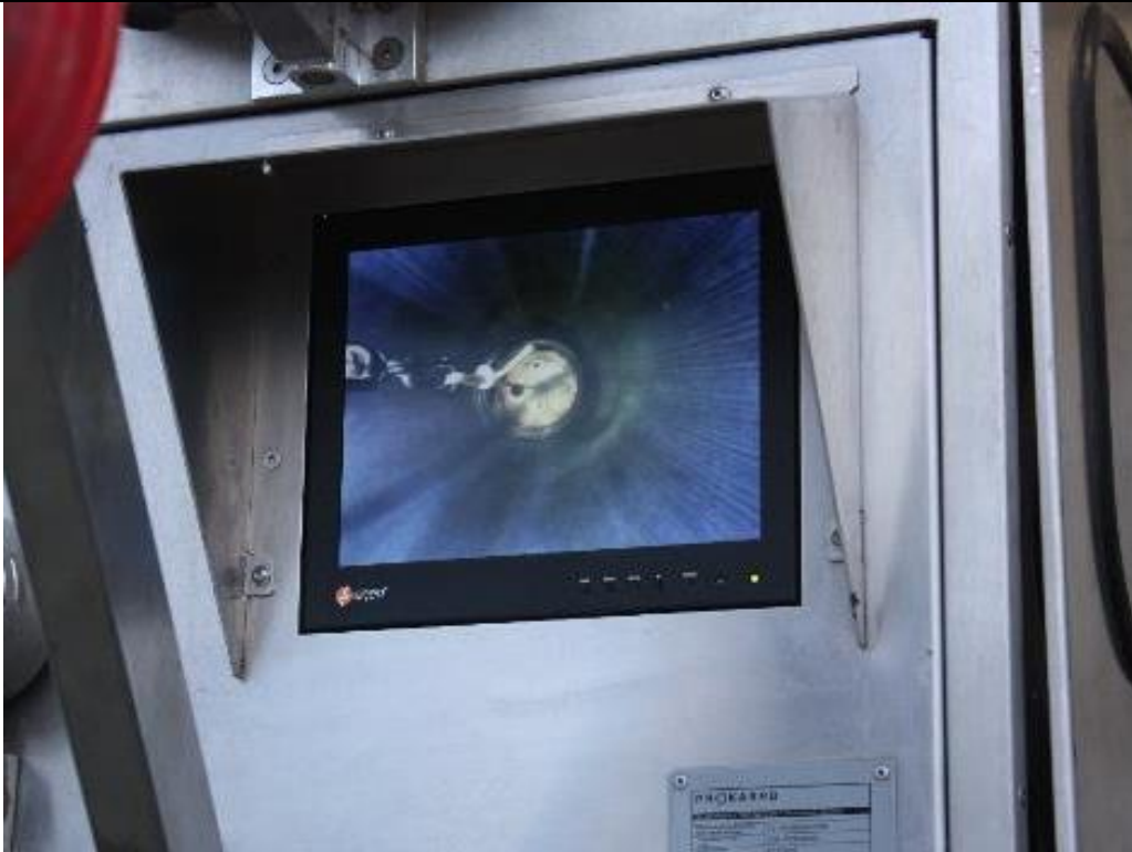
Photo 100. Once the internal pressure in the CIPP was achieved, C&L pulled the roller device which houses the UV lamps from the downstream side to the upstream side of the outlet pipe. During this time, C&L used an attached video camera to observe the condition of the CIPP. No issues were found within the inflated CIPP liner, so C&L then turned on the UV lamps to cure the CIPP pipe. The curing process lasted approximately 2.5 hours. Nov. 1, 2017.
