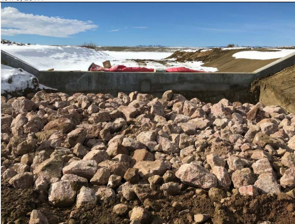
Photo 115. View looking upstream at the emergency spillway control sill located at Station ES 2+20. Note that the bedding and riprap has been installed downstream of the cutoff structure. Nov. 9, 2017.
