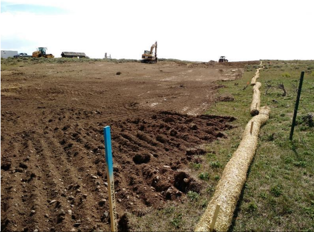
Photo 3. View looking upstream along the left side of the spillway channel at the clearing and grubbing work and the installed erosion control. Aug. 1, 2017.
