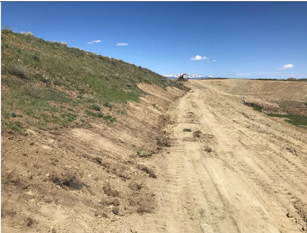
Photo 121. View looking left across the completed Main Dam Stability berm. Note that the berm and main dam slope transition was graded as per the SEO substantial completion comments. May 17, 2018.
