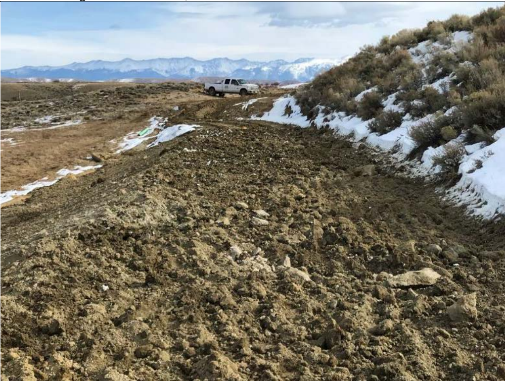
Photo 119. View looking right along the North Dam finished Stability Berm from approximate NTD Sta. 2+75 which has been shaped and scarified. Nov. 14, 2017.
