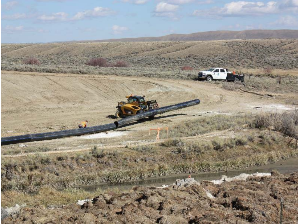
Photo 78. Photo of C&L cutting and removing the HDPE liner pipe from the Staging and Stock Pile Area. The HDPE pipe was loaded onto a trailer and removed from the site. Oct. 20, 2017.
