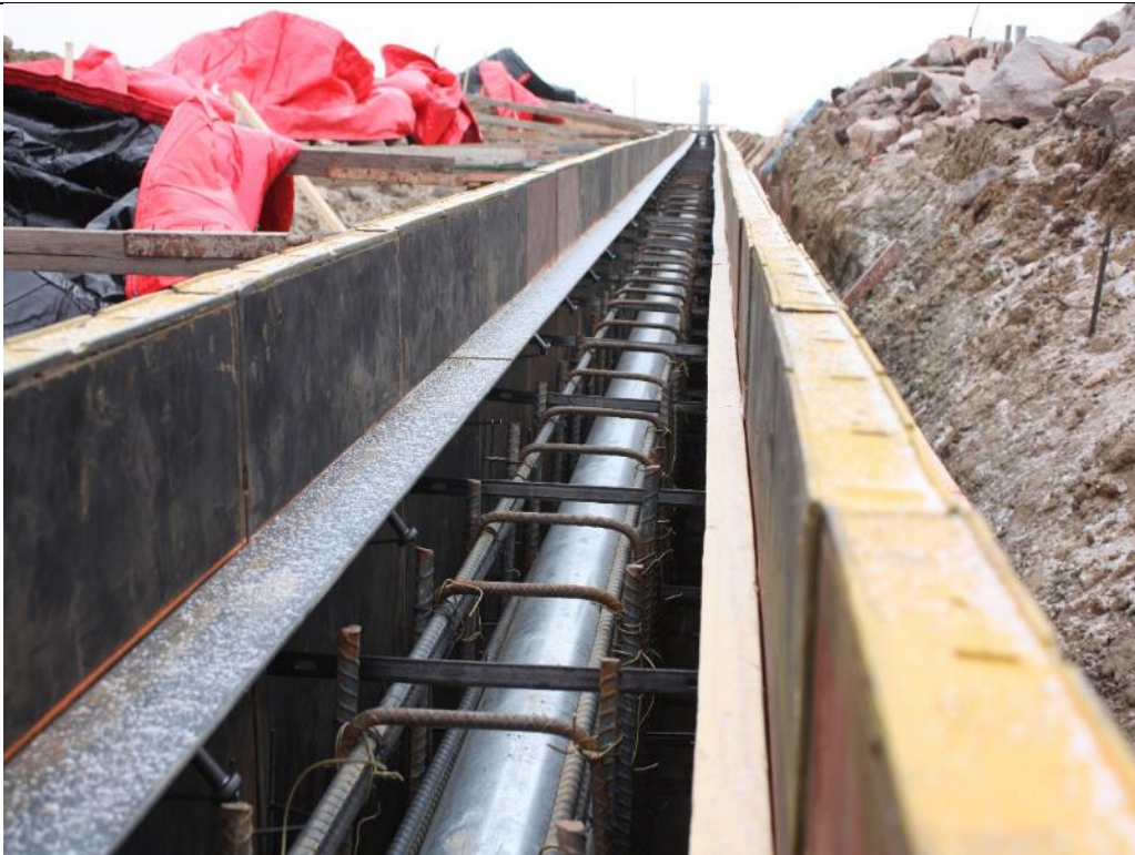
Photo 89. View looking downstream along the top of the Air Vent Encasement Wall extending parallel the gate operator along the upstream slope of the main dam. Oct. 30, 2017.
