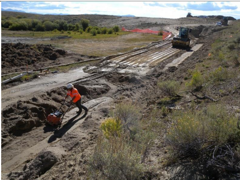
Photo 44. View looking right along the toe of the Main Dam at the compaction of the first layer of Type A Filter Sand covering the Type B Gravel Drain on the left side of the dam, and the chimney drain and start of stability berm on the right side of the Main Dam. Sept. 14, 2017.
