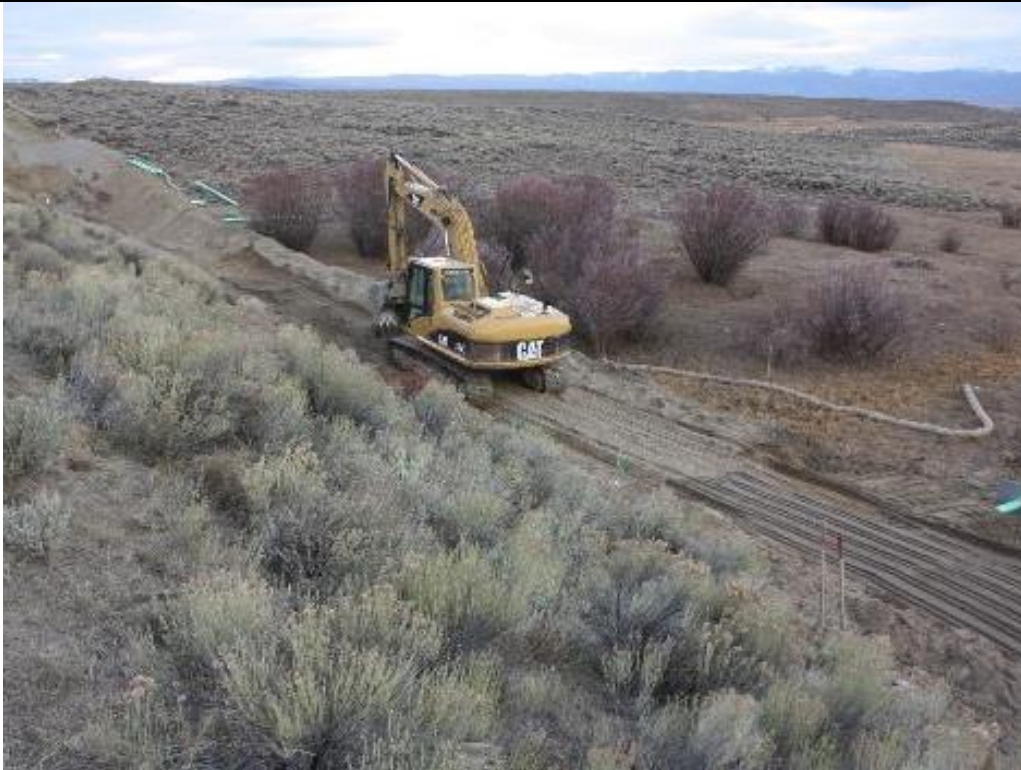
Photo 94. View looking left and downstream from approximate NTD Sta. 2+00 at the buried toe drain discharge pipe and galvanized steel plate, and the Work by RME to cover the Type B Gravel of the toe drain system. Nov. 1, 2017.
