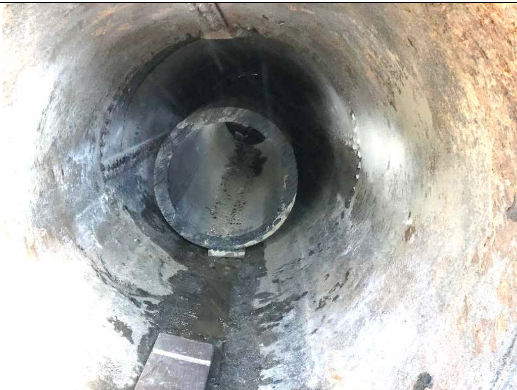
Photo 106. View looking downstream from the outlet works inlet where the HDPE liner section had been inserted into the CIPP liner at the riveted steel pipe diameter transition section. Decking was used to shim-up the base of the HDPE liner to achieve consistent annular space. Nov. 3, 2017.
