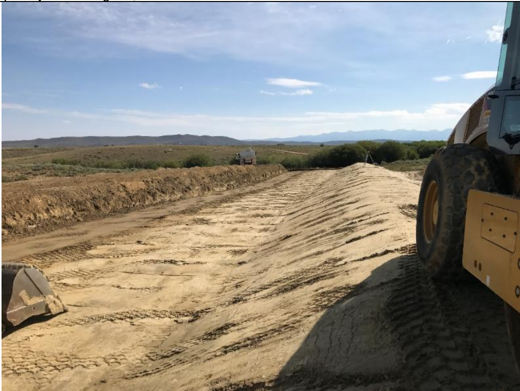
Photo 10. View from ES Sta. 3+00 looking downstream along the completed right spillway berm. Aug 11, 2017.
