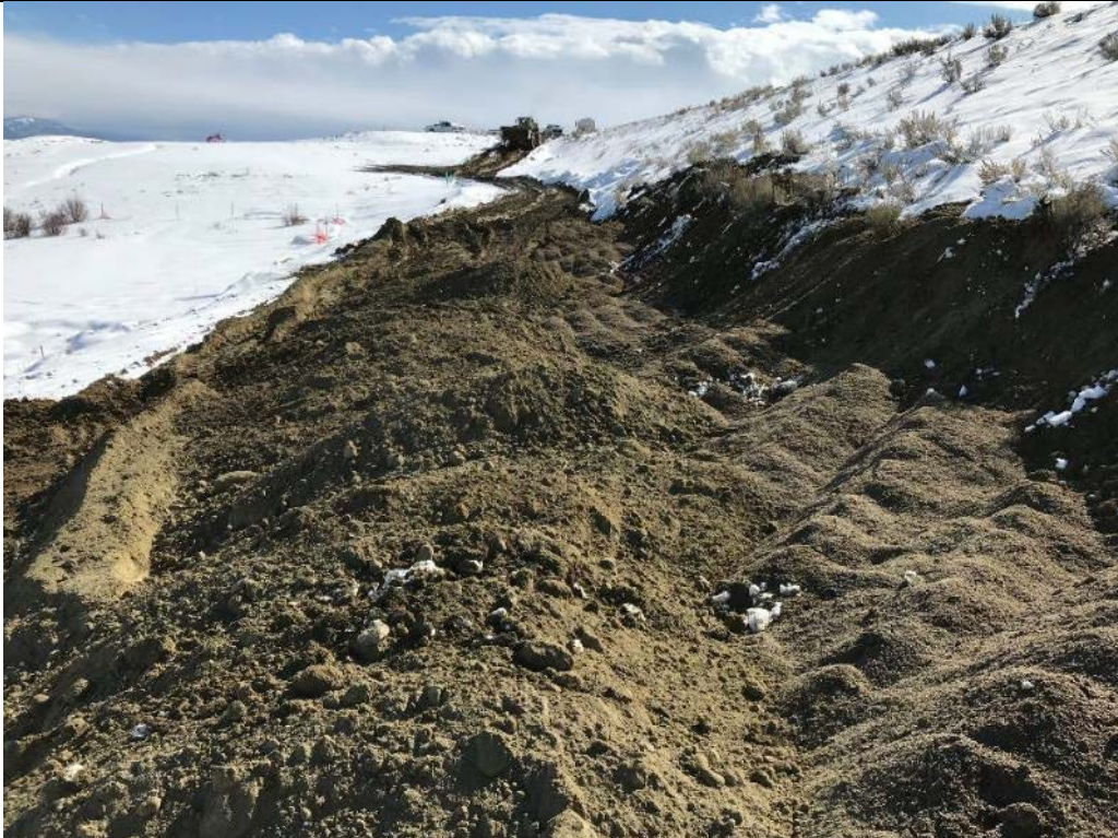
Photo 111. View looking right from Station 2+50 MTD at the final Embankment Fill lifts being installed prior to compaction along the Main Dam. Nov. 7, 2017.
