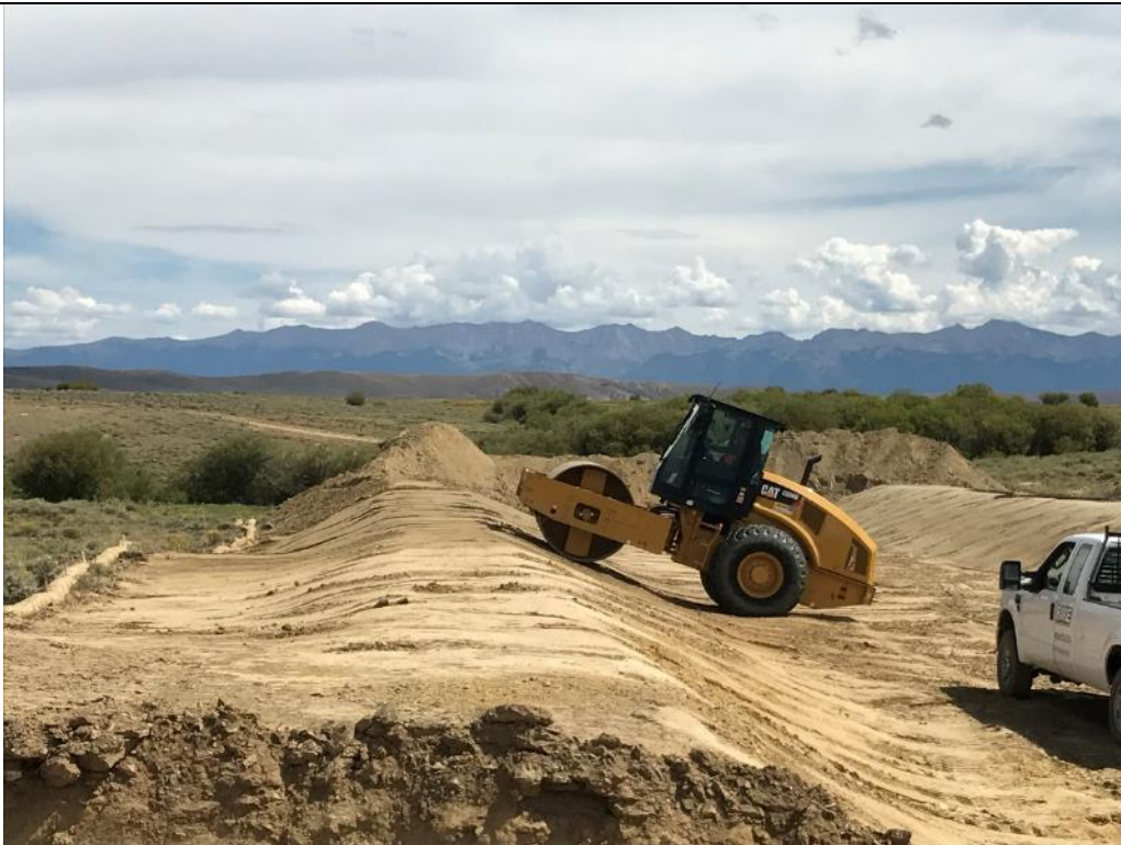
Photo 22. View looking downstream from ES Sta. 2+50 of the smooth drum rolling of the left downstream spillway berm. Aug. 24, 2017.
