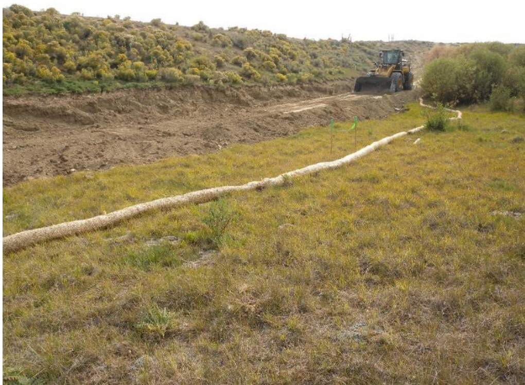
Photo 35. View looking upstream and left from approximate Sta. 4+50 at the foundation preparation work for the North Embankment Stability Berm, which included hauling and placing Embankment Fill along the North Embankment downstream toe. Sept 7, 2017.
