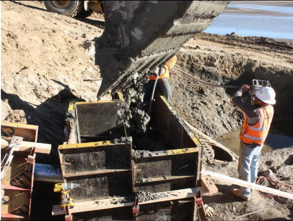
Photo 86. View of the concrete placement for the Air Vent Riser section and Air Vent Encasement Wall anchor section. Oct 24, 2017.
