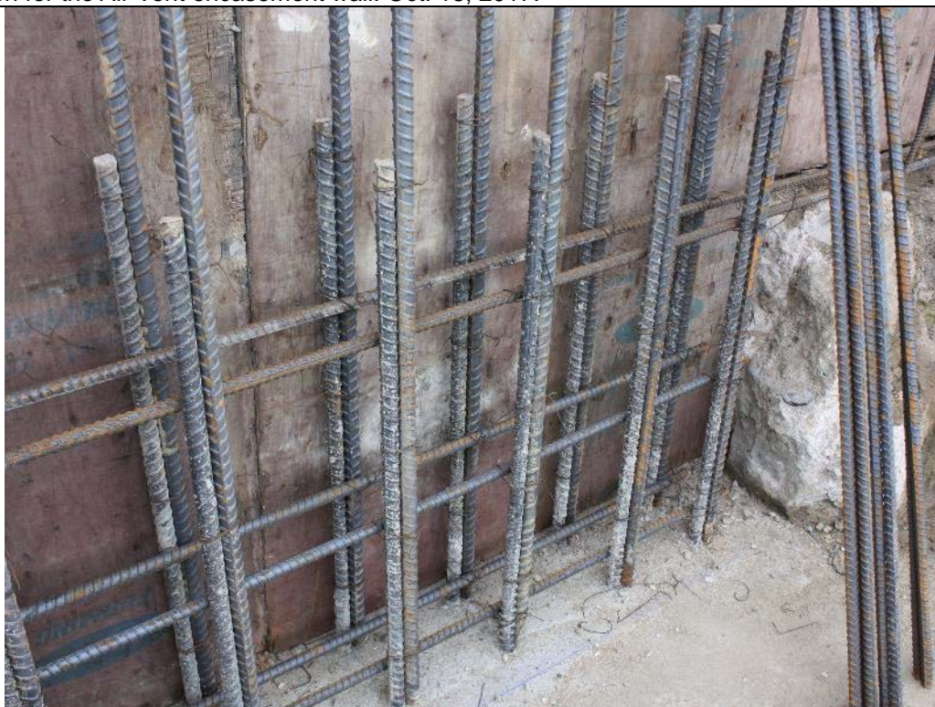
Photo 77. View looking down at the #8 rebar rising from within the wing wall foundation which was then tied to the vertical #8 rebar for the new outlet works terminal structure headwall. Oct. 19, 2017.
