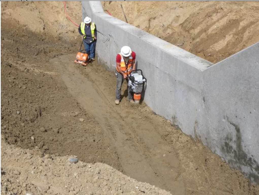
Photo 66. View of the special compaction around the upstream spillway cutoff wall during the backfilling process. Sept. 30, 2017.
