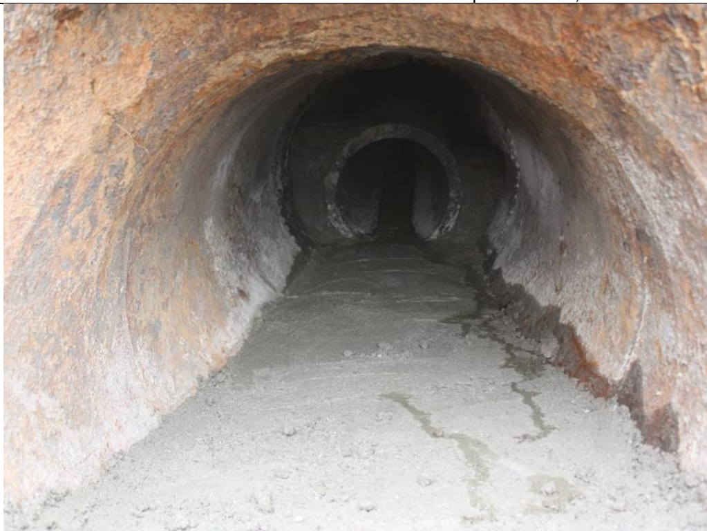
Photo 107. View looking downstream into the inlet of the outlet conduit at the original riveted steel host pipe transition section which had been filled in along the bottom up to the invert of the HDPE liner pipe with concrete. Nov. 4, 2017.
