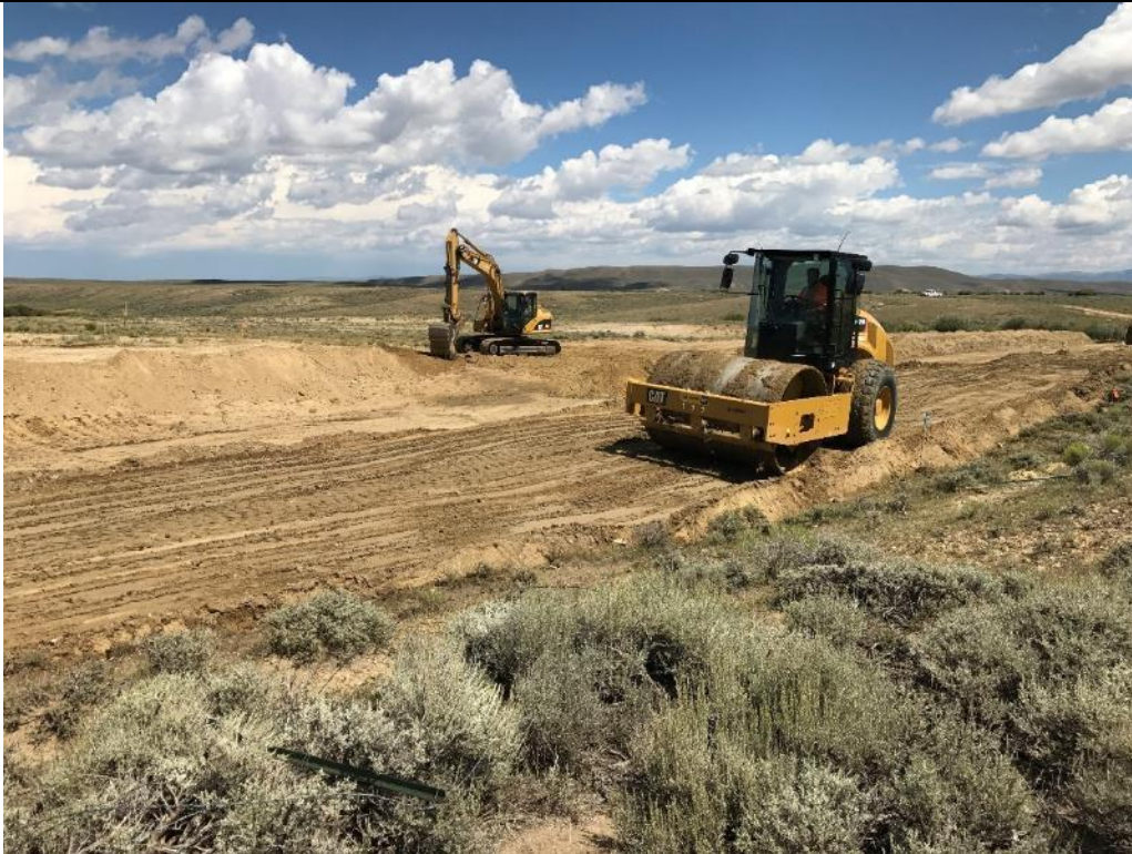
Photo 11. View of compaction of the right spillway berm from ES Sta. 1+00 to 3+00. Aug. 11, 2017.
