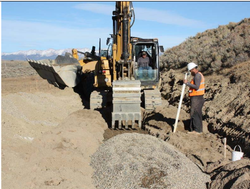
Photo 74. View of the method to install the toe drain on the North Embankment due to restricted access by construction equipment. The excavator used the bucket to obtain Type B Gravel Drain from the loader and place it into the trench and surround the slotted drain pipe. Oct. 16, 2017.
