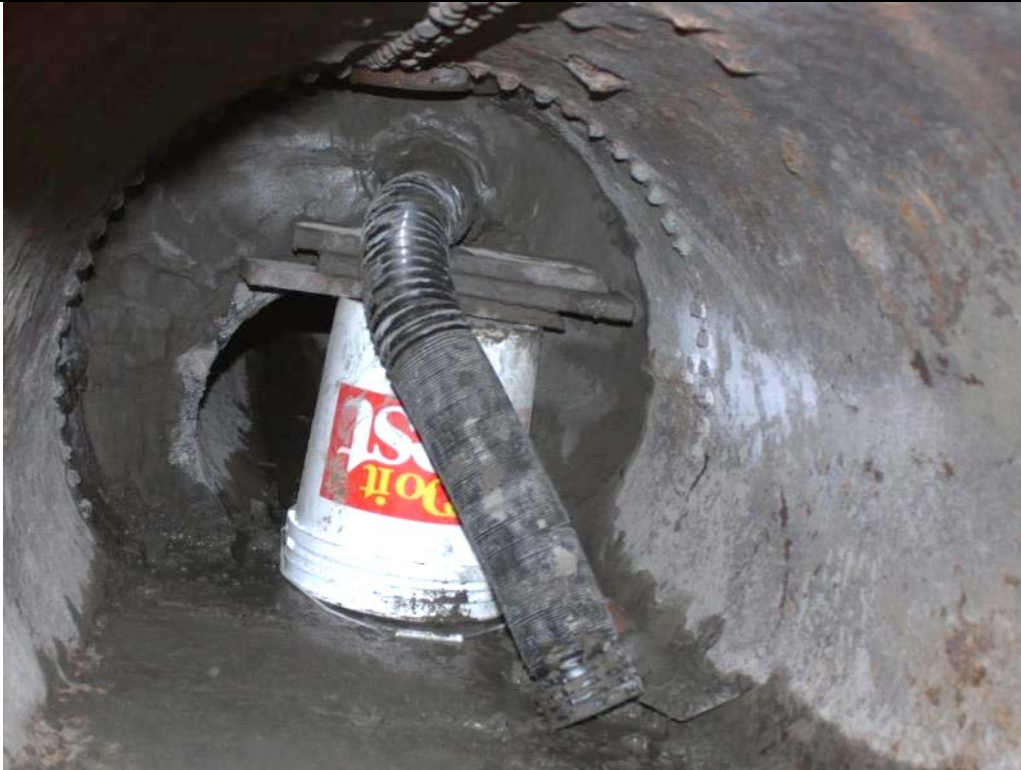
Photo 108. View looking downstream at the upper half of the bulkhead which was built after grouting the bottom half of the HDPE annular space. Note the 4-inch-diameter flexible hose was encased in the bulkhead and was used to finalize the annular space grouting once the bulkhead was set. Nov. 4, 2017.
