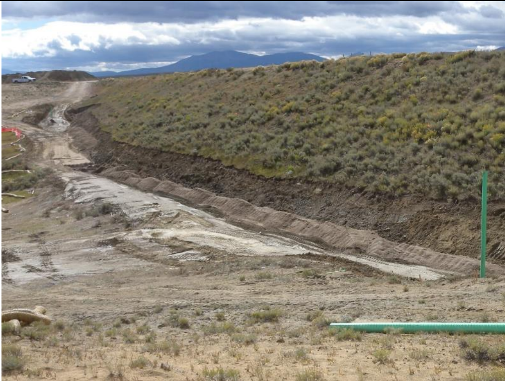
Photo 47. View looking right from the left abutment of the Main Dam at the continuation of the chimney drain and stability berm on the left and right side of the Main Dam outlet works. Note that the toe drain pipe sections at the location of the outlet works were left open. Sept. 15, 2017.
