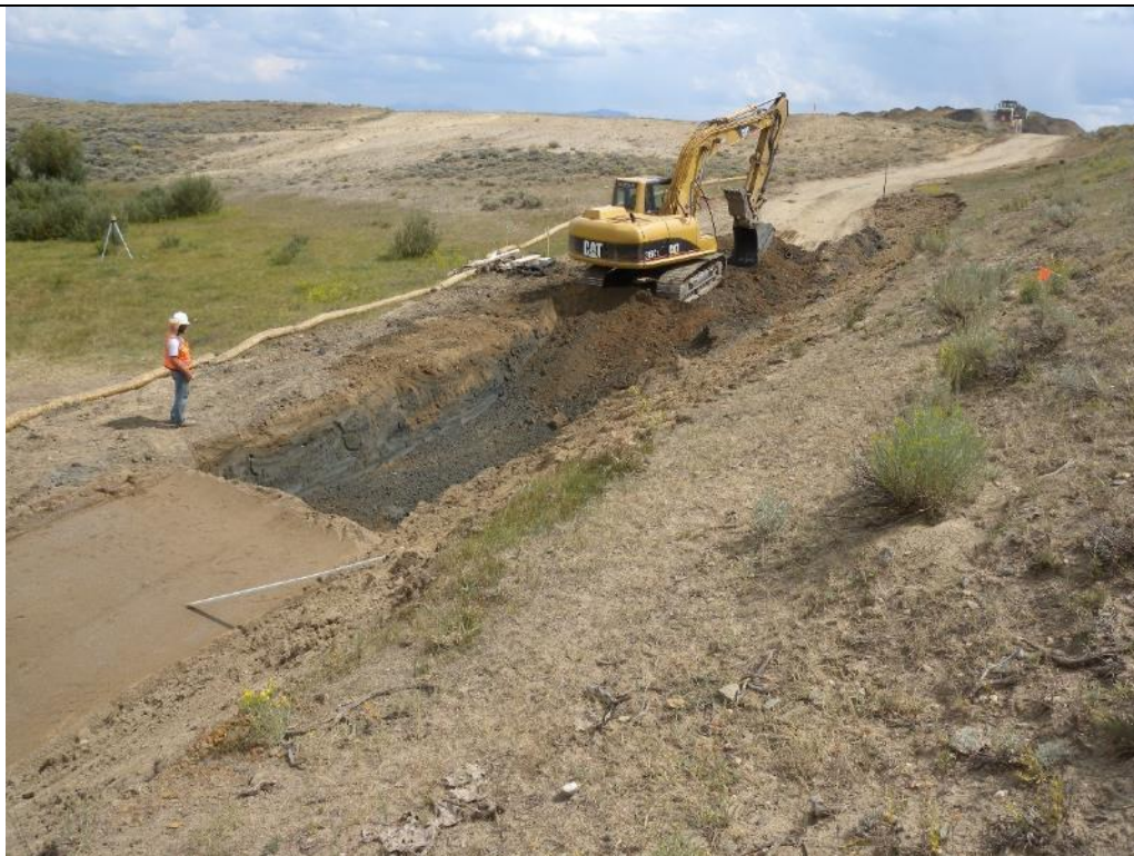
Photo 31. View looking right from MTD Sta. 3+50 at continued excavation into the Main Dam toe for the seepage collection system. The excavation is from MTD Sta. 4+00 to 4+30. Aug. 31, 2017.
