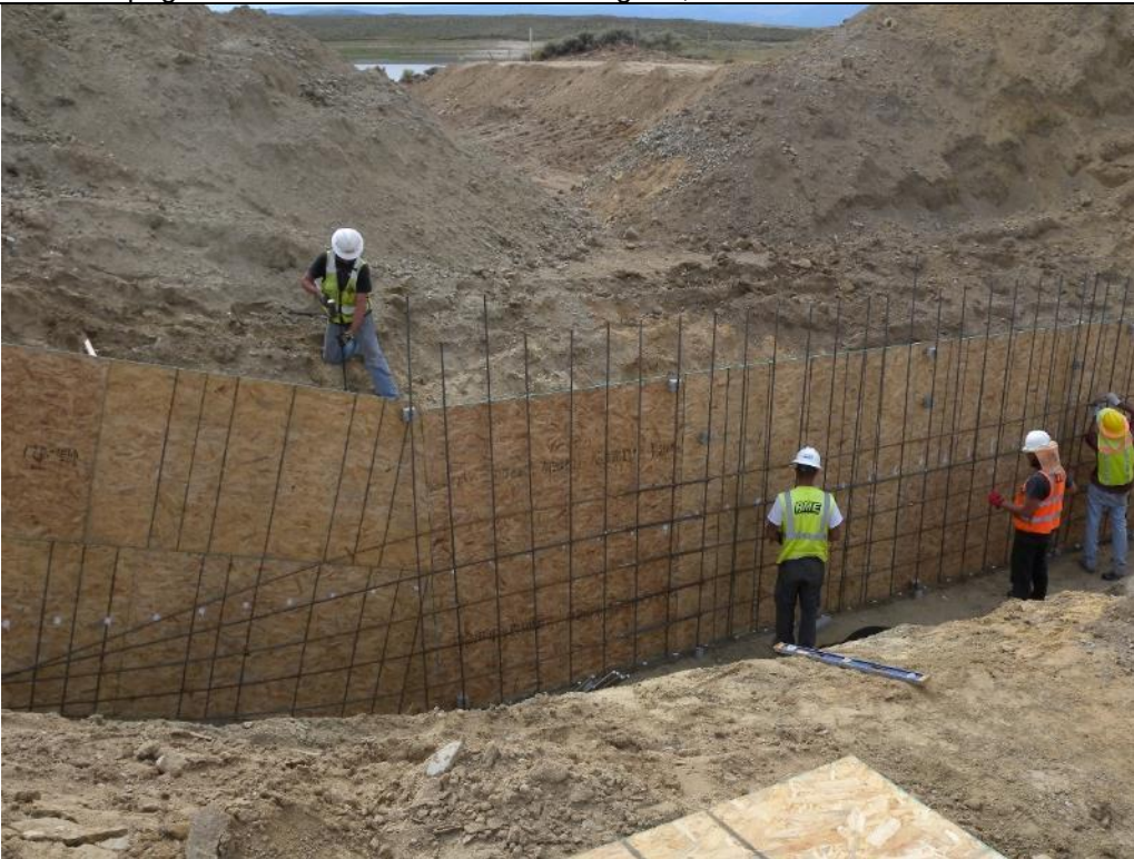
Photo 16. View of the formwork and rebar installation for the upstream spillway cutoff wall at ES Sta. 2+20. Aug. 15, 2017.
