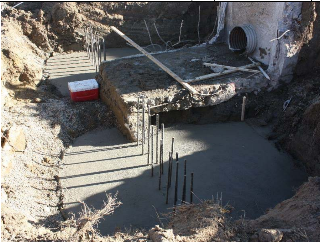
Photo 77. View looking right at the trowel finished surface of the bank poured left and right wingwall foundations. Note the test cylinders which are curing in the red cooler at the base of the old outlet works terminal structure. Oct. 18, 2017.
