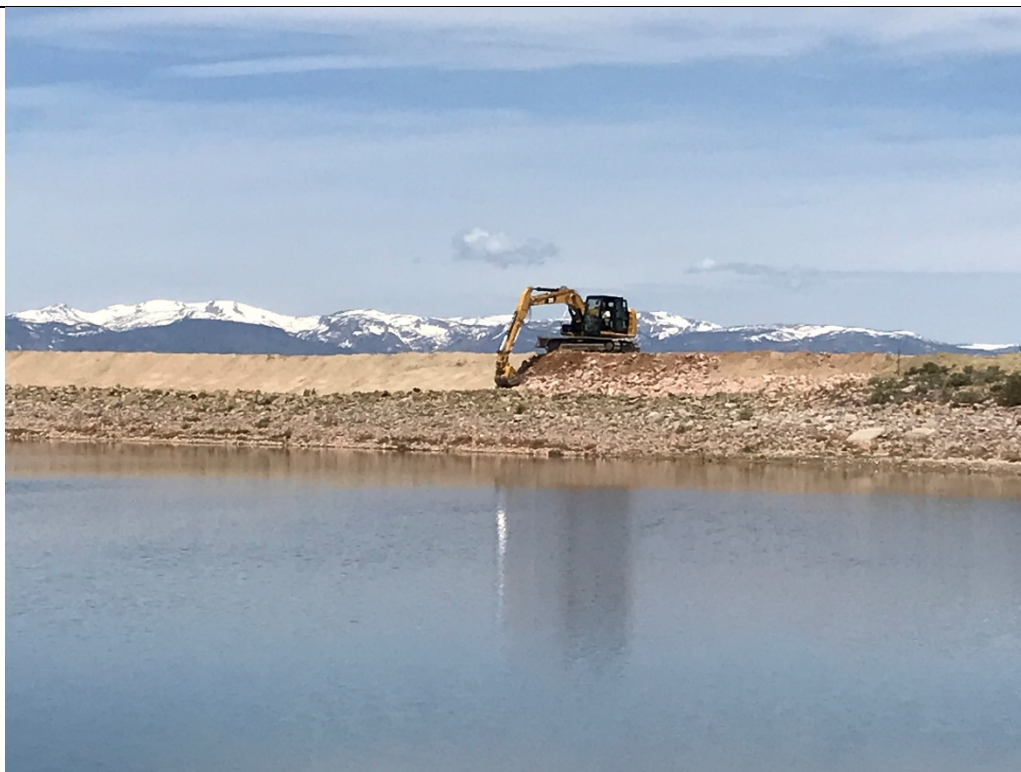
Photo 125. View looking left from the outlet works operator at the North upstream slope riprap repair being completed by the FWS maintenance crew. May 22, 2018.
