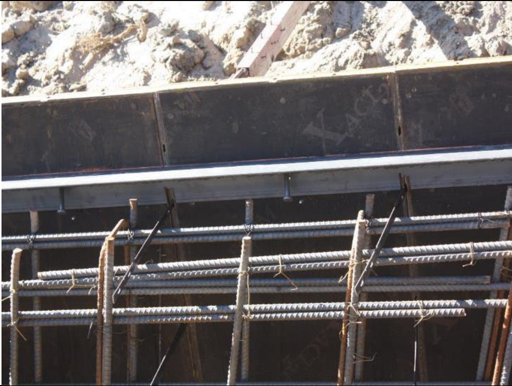
Photo 88. Close-up view of the angle iron, which to accommodate the form ties had a notch cut into the bottom portion. The angle iron was embedded into the concrete for the reservoir staff gage. Oct. 25, 2017.
