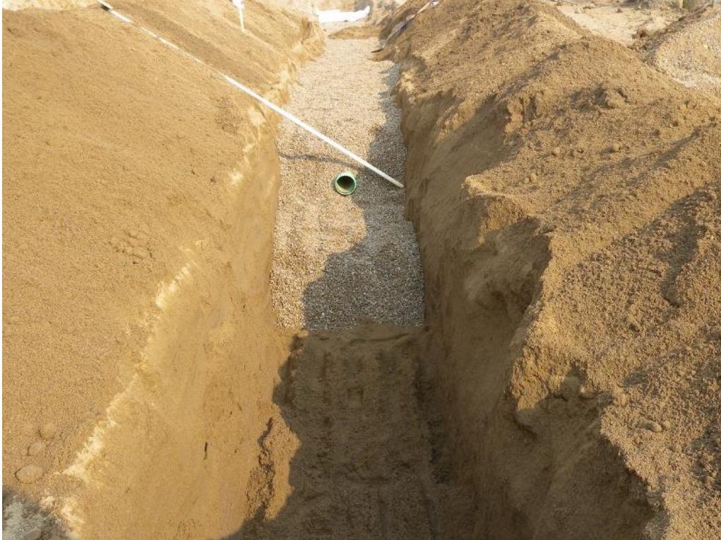
Photo 34. Representative view of the installation of the Type B Gravel Drain surrounding the slotted drain pipe. Sept. 7, 2017.
