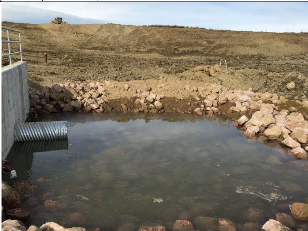
Photo 117. View looking left across the downstream terminal structure plunge pool. Note that the approximate invert elevation of the outlet pipe measured relative to the headwall is at Elevation 8281.2, which is 0.8 feet lower than the design elevation, and currently submerged by approximately 0.3 feet of water. The plunge pool was lowered in the spring of 2018. Nov. 14, 2017.
