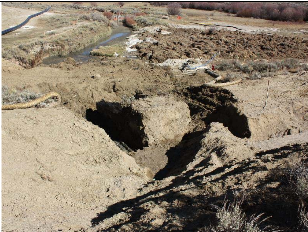
Photo 76. View looking downstream at the excavation around the existing outlet works headwall for the filter collar, which included the removal of the old toe drain discharge pipes, and the temporarily filled in section of the outlet plunge pool required for construction access. Oct. 17, 2017.
