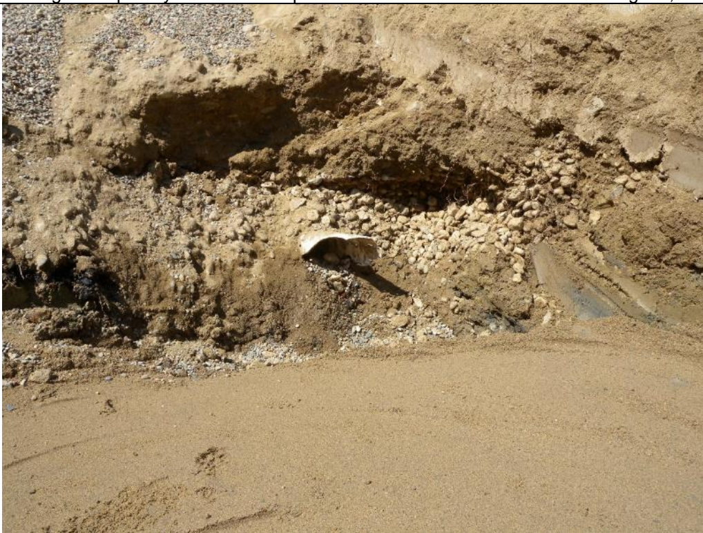
Photo 24. View looking left from approximate MTD Sta. 2+50 at the previous toe drain encountered during excavation of chimney drain. Aug. 28, 2017.
