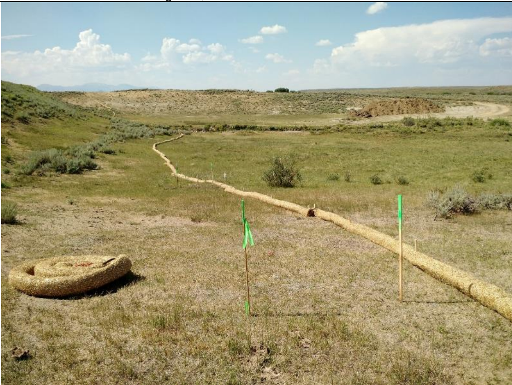
Photo 2. Erosion control wattles staked down at the toe of the Main Dam Embankment. View looking left along the toe of the Main Dam Embankment. August 1, 2017.
