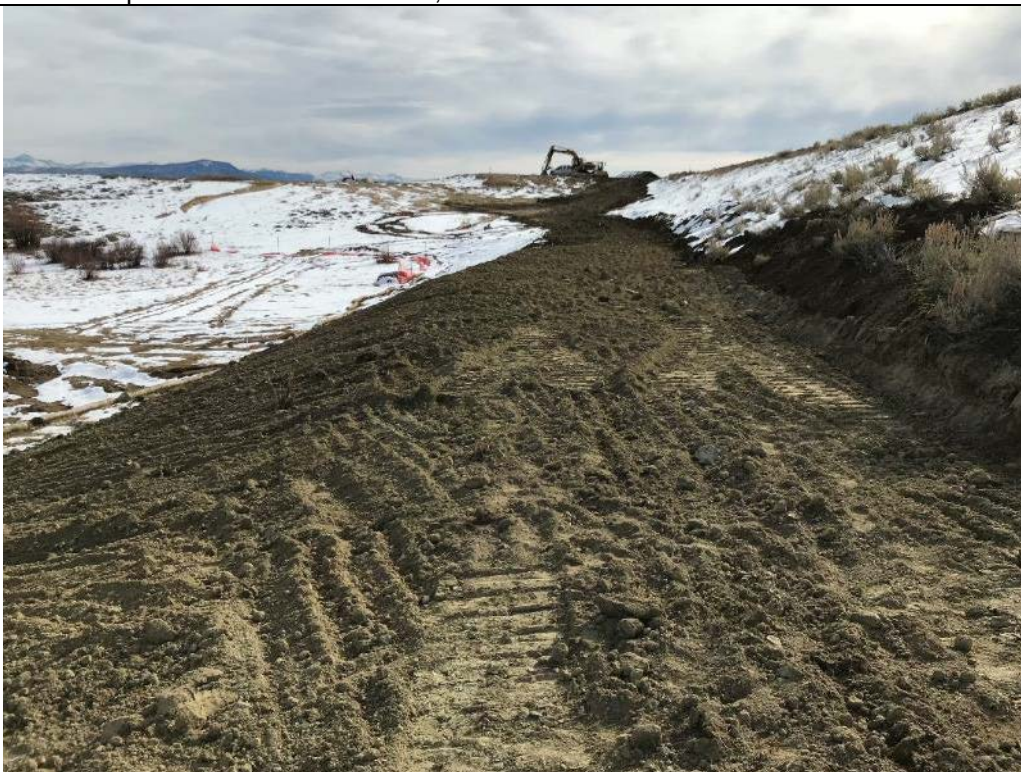
Photo 119. View looking right along the Main Dam finished Stability Berm from approximate NTD Sta. 2+50 which has been shaped and scarified. Nov. 14, 2017.
