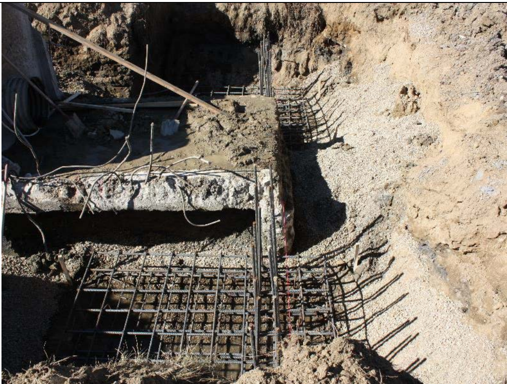
Photo 76. View looking left across the outlet works terminal structure at the left and right wingwall foundation rebar and head wall risers which were tied and in-place prior to the concrete bank pour.
