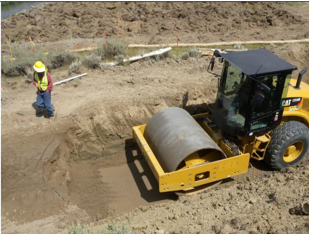
Photo 29. View looking downstream at the smooth drum roller compacting the Type A Filter Sand. Aug. 29, 2017.
