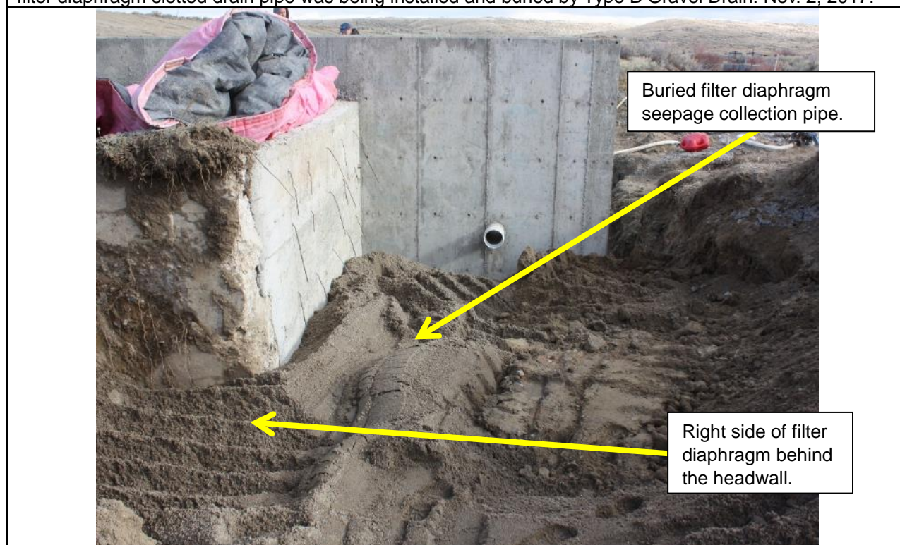
Photo 103. View looking downstream at the right side of the outlet works terminal structure headwall. The filter diaphragm slotted drain pipe was now buried by Type A Filter Sand, and the filter diaphragm was starting behind the old terminal structure headwall. Nov. 2, 2017.
