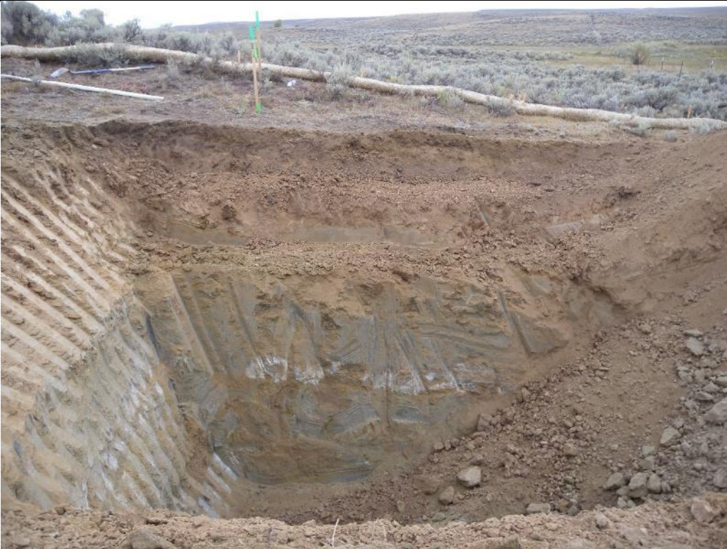
Photo 49. View looking downstream from NTD Sta. 0+00 at the excavation down to the base of the seepage collection system at the left toe drain cleanout. Sept. 15, 2017.
