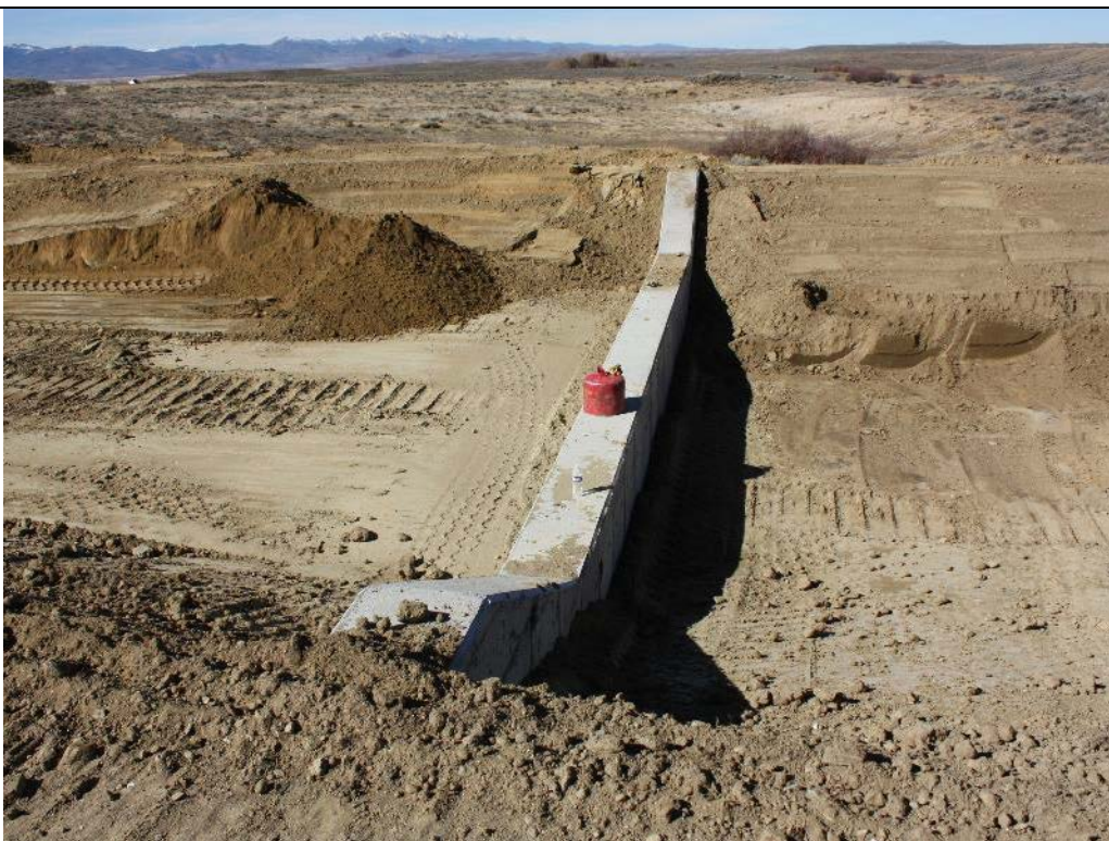
Photo 79. View looking left across the downstream spillway cutoff wall which has been backfilled. Oct. 17, 2017.
