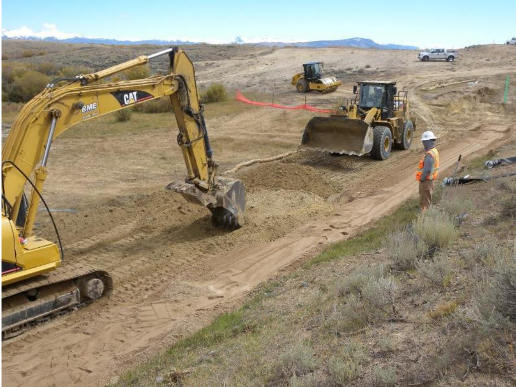
Photo 61. View looking downstream from approximate MTD Sta. 3+75 of the Embankment Fill placement in the Stability Berm. Sept. 26, 2017.
