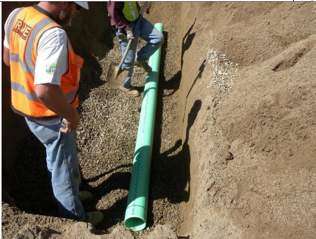
Photo 42. View looking left from MTD Sta. 2+45 at the placement of the first section of slotted drain pipe for the left side of the Main Dam seepage collection system from MTD Sta. 2+40 to 2+26. Sept. 13, 2017
