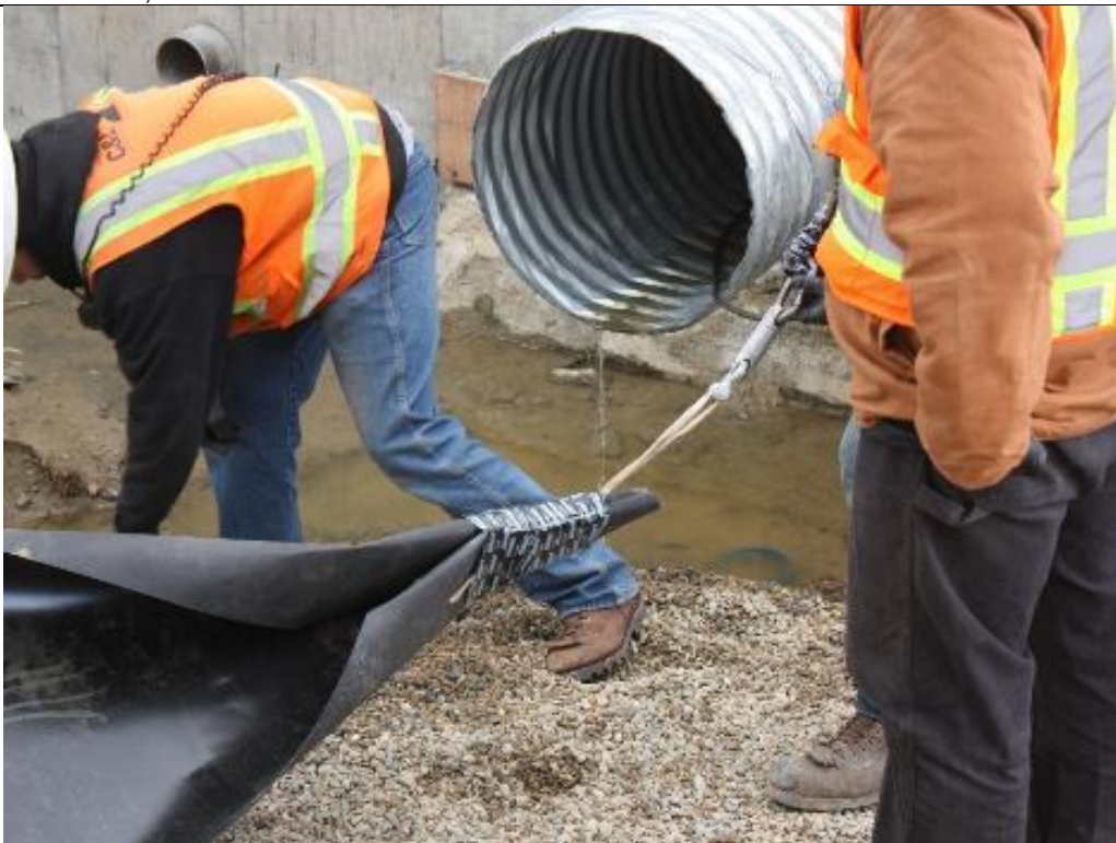
Photo 95. View of the protective liner which was pulled through the original outlet works conduit prior to pulling through the CIPP liner. This base material covered the bottom half of the host pipe and provided a smooth surface and protection for when the CIPP liner was subsequently pulled through the conduit. Nov. 1, 2017.
