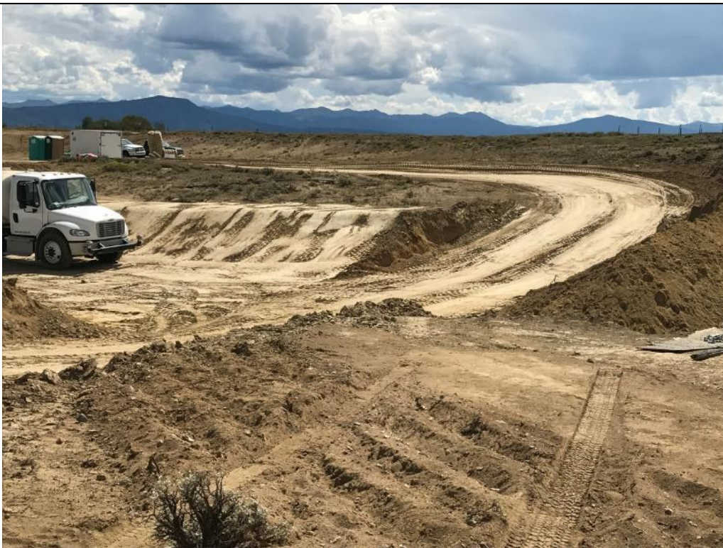
Photo 23. View looking from the left side of the spillway at the right spillway berm and new access road alignment through the spillway between the upstream and downstream cutoff walls. Aug. 24, 2017.
