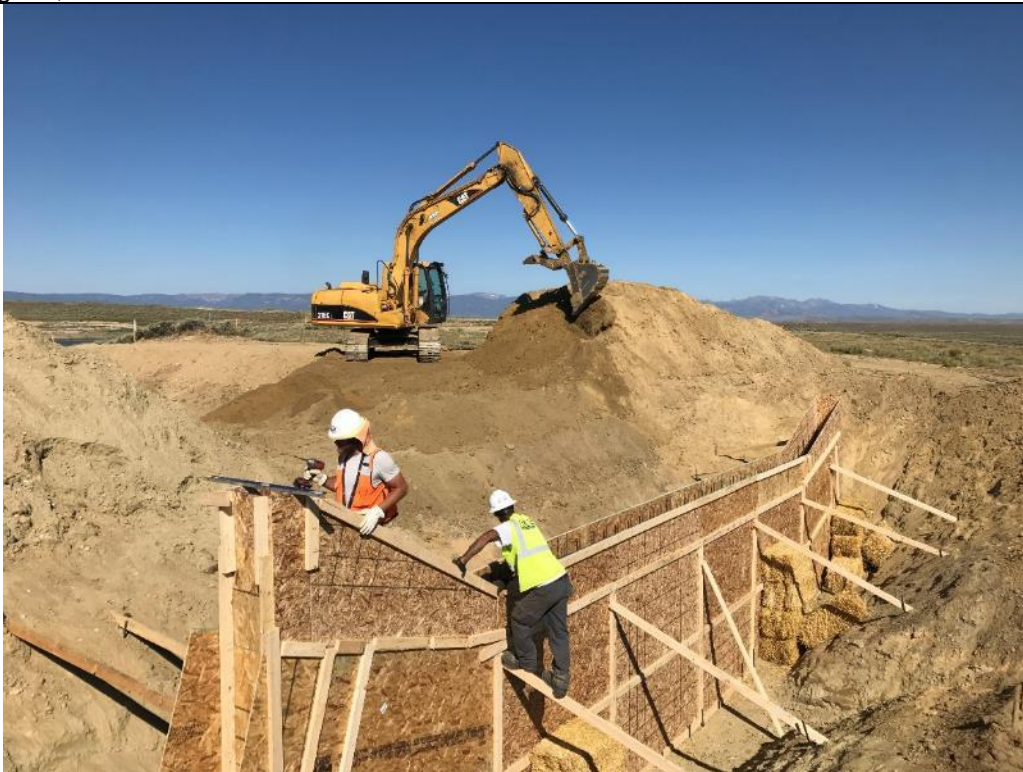
Photo 18. View of the completed formwork for the upstream spillway cutoff wall at ES Sta. 2+20. Aug. 18, 2017.
