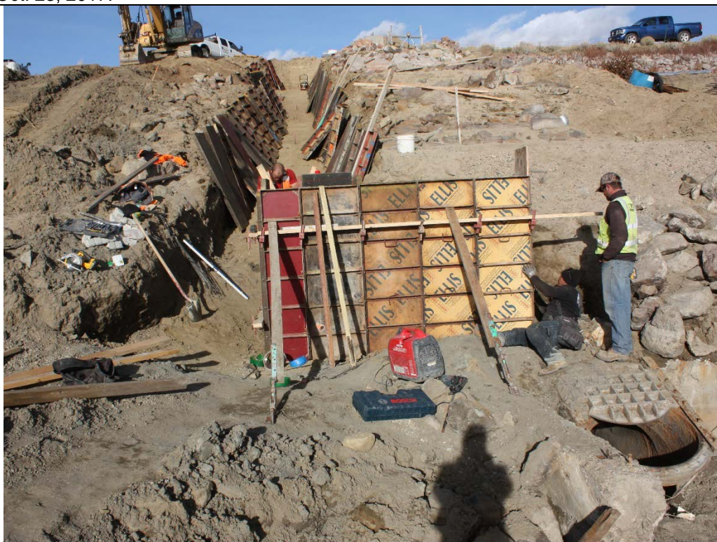
Photo 85. View from the coffer dam looking downstream at the riser section of the Air Vent encasement wall which extends from the attachment to the original riveted steel outlet works conduit to the start of the air vent pipe encasement wall. Oct. 23, 2017.
