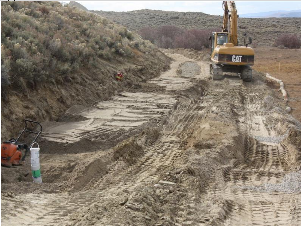
Photo 79. View looking left from NTD Sta. 5+15 at the top layer of Type A Filter Sand being placed and spread by the excavator which represents the top of sand layer for the North Dam Toe Drain. Oct. 20, 2017.
