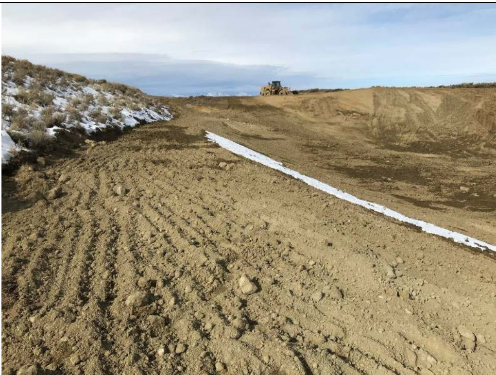
Photo 118. View looking left along the Main Dam finished Stability Berm from approximate MTD Sta. 2+50 which has been shaped and scarified. Nov. 14, 2017.
