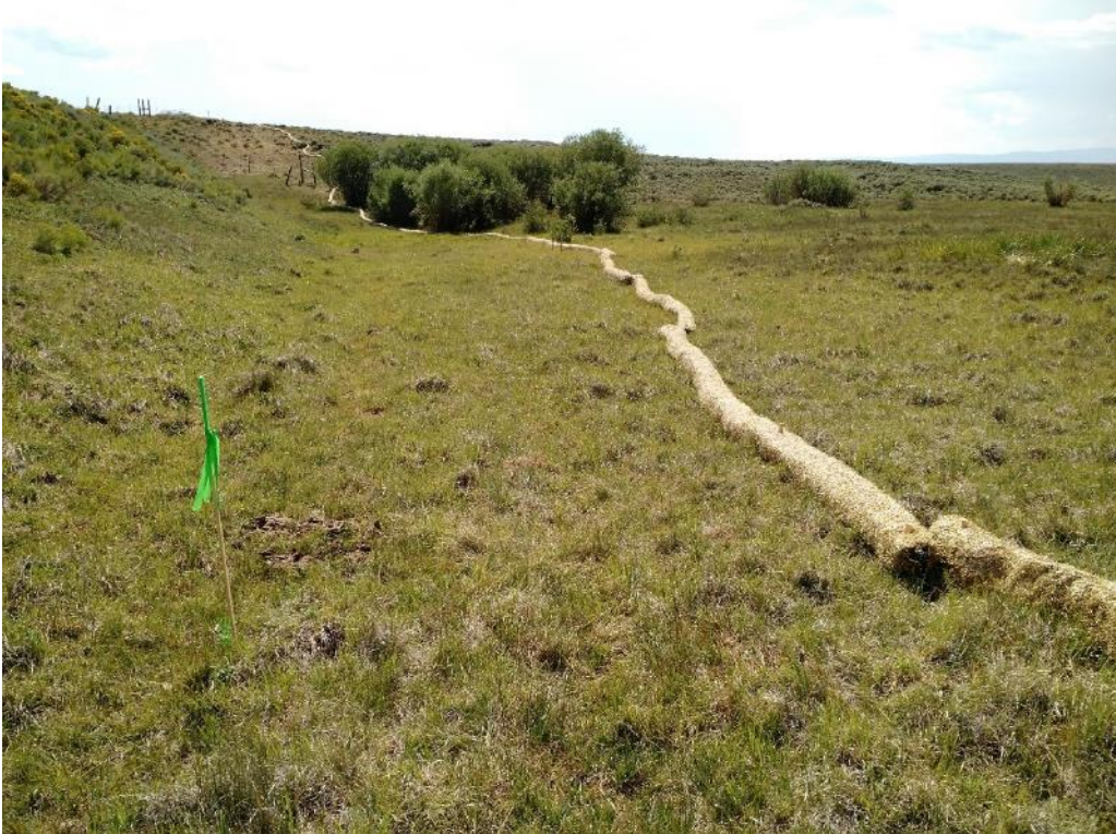
Photo 1. Erosion control wattles staked down at the toe of the North Embankment. View looking left along the toe of the North Embankment. August 1, 2017.
