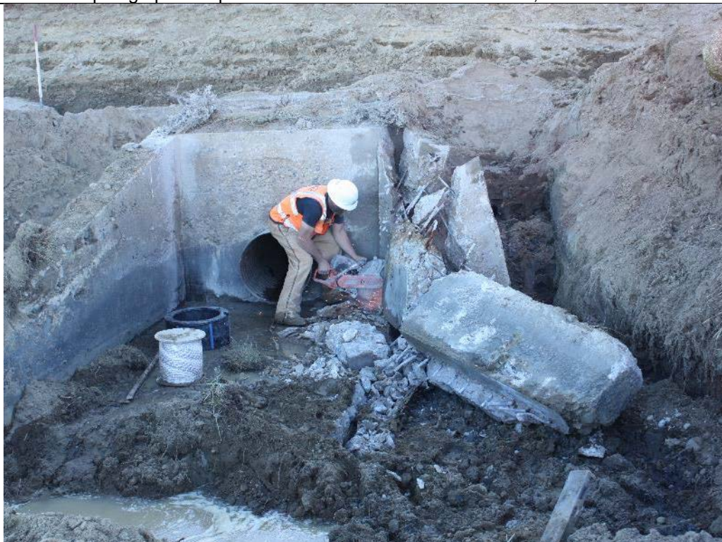
Photo 77. View looking upstream from the temporarily filled in outlet plunge pool at the demolition of the existing outlet structure wing walls. Oct. 17, 2017.
