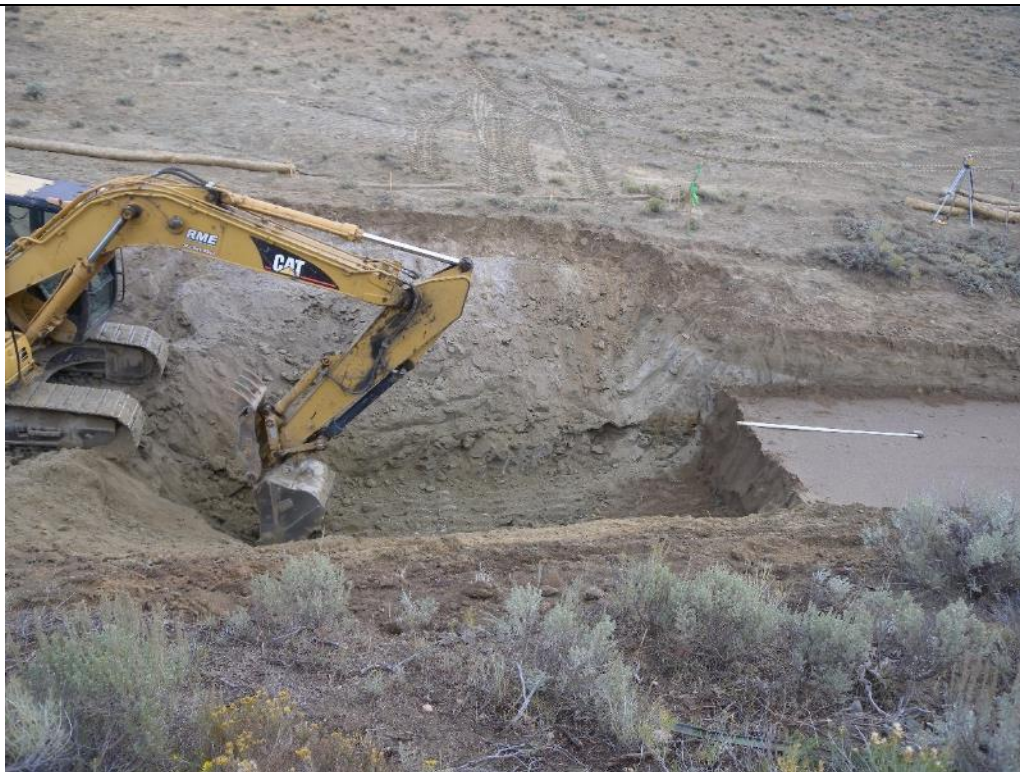
Photo 41. View looking downstream at the excavation from MTD Sta. 0+35 to 0+50. The excavator shown above was trying to cut into a rapidly rising layer of sandstone/claystone bedrock that appeared near MTD Sta. 0+35. It was decided after discussions with the SEO, Kumar and Wheeler to end the toe drain at MTD Sta. 0+50 instead of 0+00 and place the toe drain cleanout at MTD Sta. 0+45. Sep. 13, 2017.
