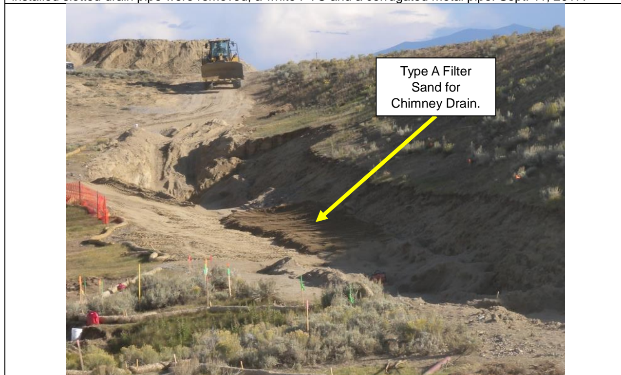
Photo 40. View looking right at the first lift of Type A Filter Sand that represents the start of the chimney drain from MTD Sta. 3+00 to 4+50. Sept. 12, 2017.
