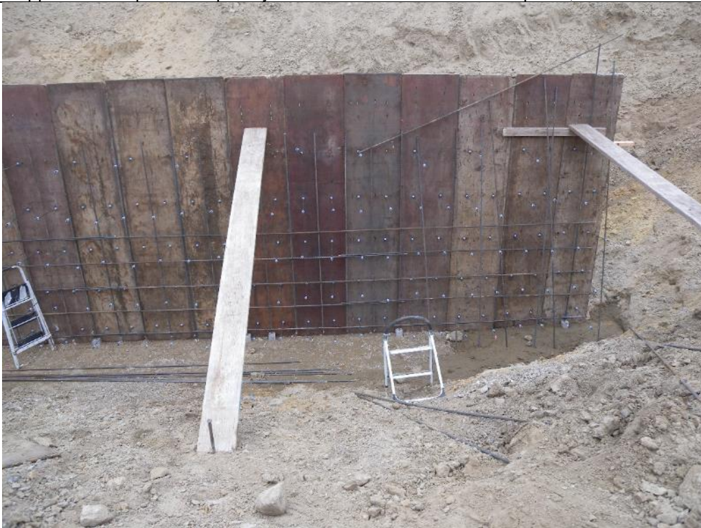
Photo 58. View of the formwork and rebar installation for the downstream spillway cutoff wall located at ES Station 5+20. Sept. 22, 2017.
