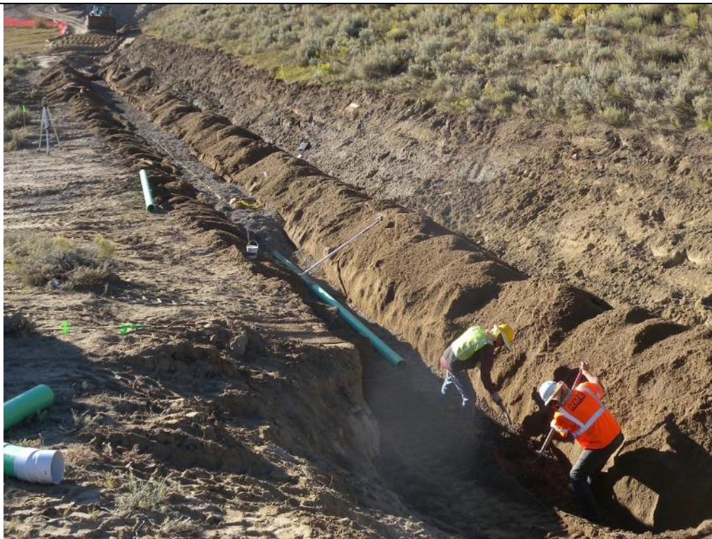
Photo 43. View looking right from approximate MTD Sta. 0+50 at a representative view of the Main Dam, right Chimney Drain installation and placement of the Embankment Fill Lift from MTD Sta. 3+00 to 4+00. Sept. 14, 2017.
