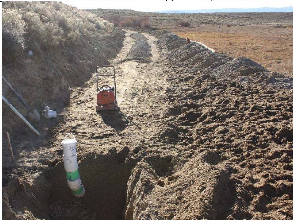
Photo 75. View looking left from NTD Sta. 5+15 at work on the North Dam Seepage Collection System including installing the slotted drain pipe, Type B Gravel drain in the Type A Filter Sand, and the Toe Drain cleanout. From approximate NTD Sta. 3+34 to 4+50, the Type A Filter Sand layer stopped at a lower elevation than elsewhere along the seepage collection system, which meant that RME had mound the Type B gravel over the slotted pipe for the required 1-foot of coverage. Oct. 17, 2017.
