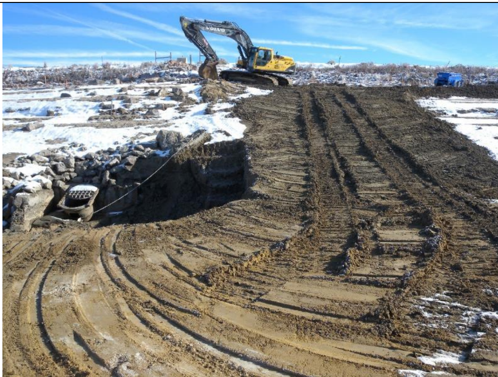
Photo 68. View of the top of the re-constructed coffer dam. The original coffer dam was washed out following the rising reservoir levels associated with the snow storm from October 1. Oct. 10, 2017.
