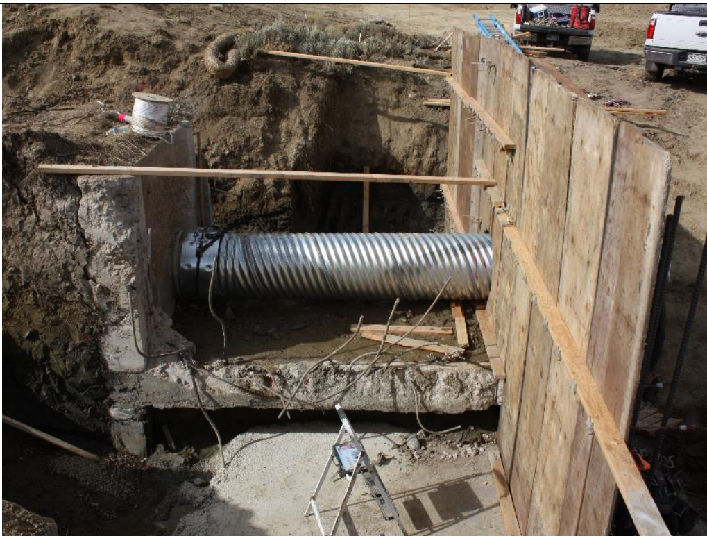
Photo 76. View looking left from approximate MTD Sta. 2+60 at the CMP extension and downstream side of the headwall form.
