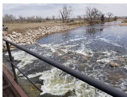
Figures 4 & 5 - Bank stabilization upstream and downstream of diversion structure.
