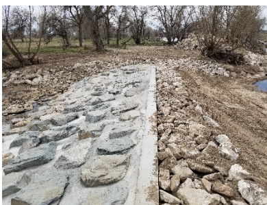
Figure 2 - Diversion repair on South side of diversion structure.
