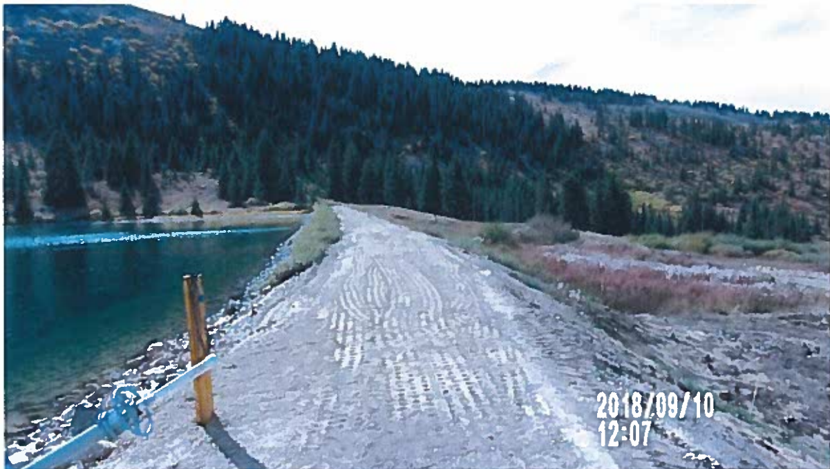
Dam crest with new fill, View to South
