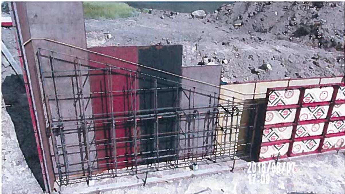
Rebar for Control Wall being installed, view to East
