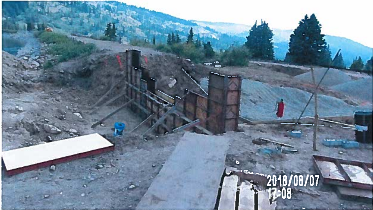
Concrete form work for Control Wall, View to Southwest
