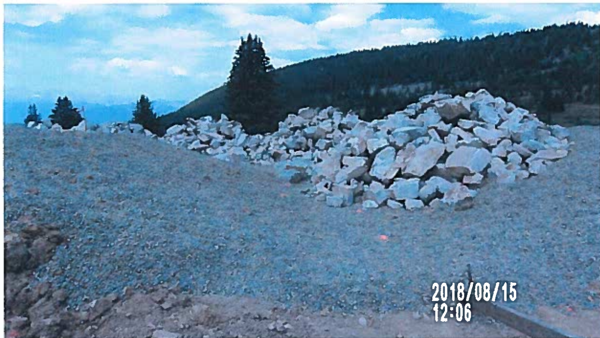
View of spillway channel downstream of Control Wall showing bedding and riprap before placement, View to West
