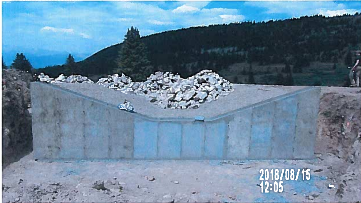
Completed Control Wall before backfilling, View to West
