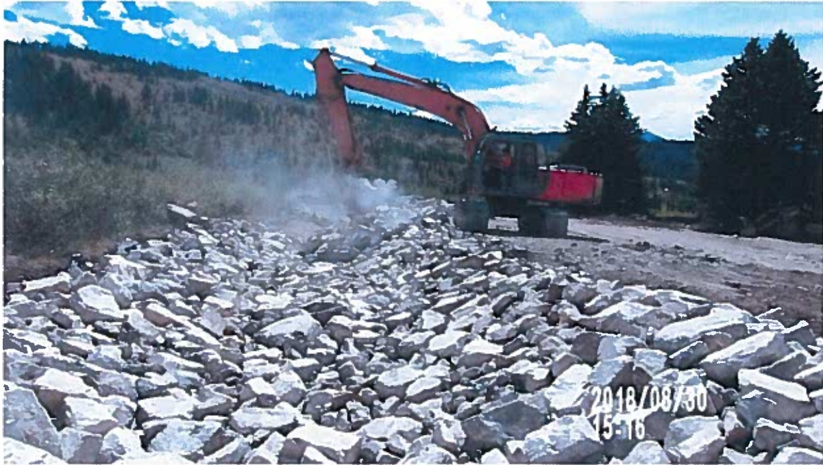
Riprap being placed in spillway channel, View to South
