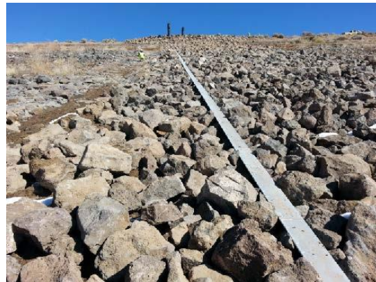
Figure 5 - After construction - new staff gage
