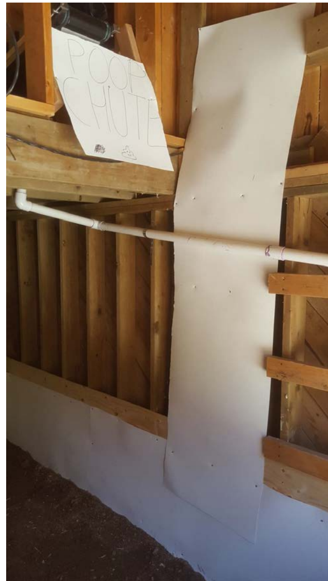
Figure 12. Vinyl sheeting to keep the wood surfaces clean/from rotting.
