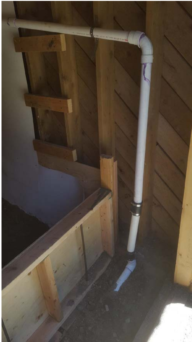
Figure 11. Urine drain line where it ties into the existing leach field.
