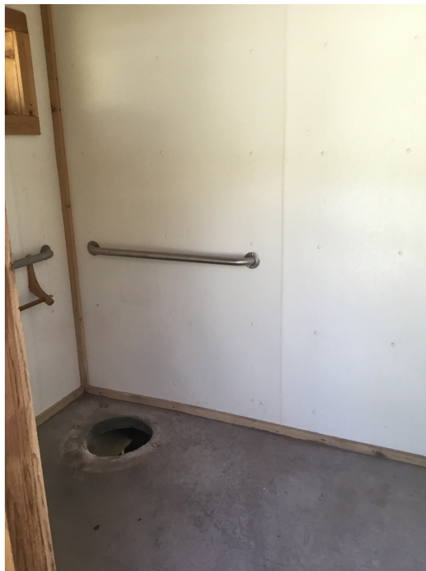
Figure 6. Removal of the old toilet.
