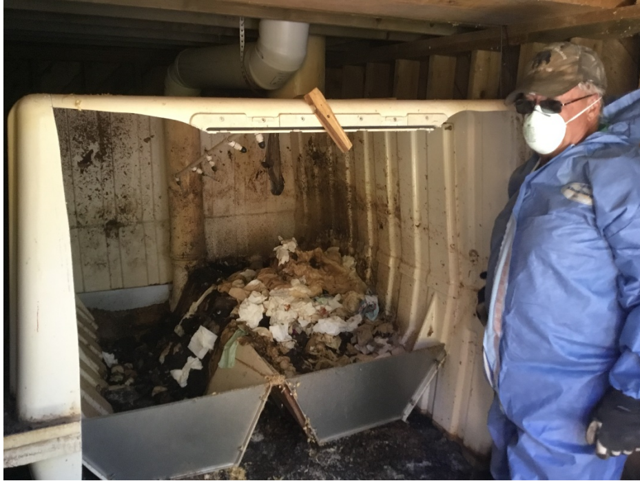
Figure 5. Removal of waste from the vault. The vault was also removed leaving an empty chamber below the toilet.
