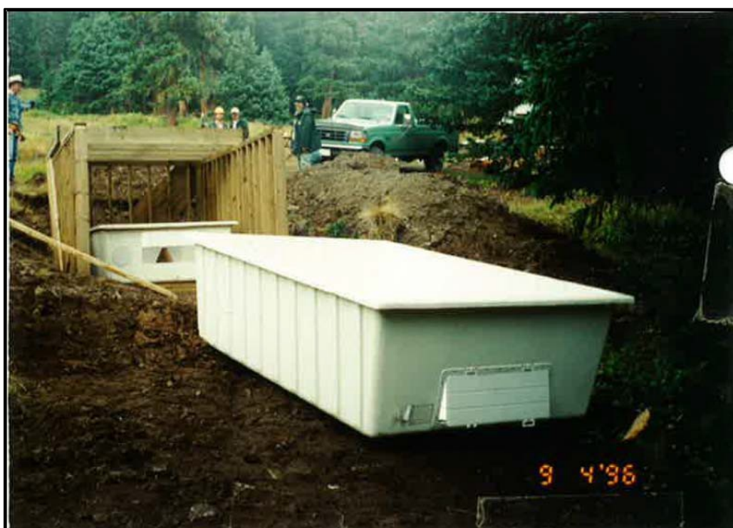
Figure 2. Installation of Nellie Creek toilet in September 1996.
