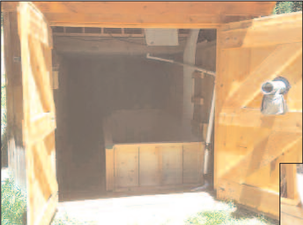
Behind the scenes view at newly revamped Uncompahgre Trailhead toilet, left, shows lowest level of building with vented swinging doors accessing waste crib and piping for urine drain. Bottom photo also illustrates end of conveyor belt, below left, and chute into the containment area.
