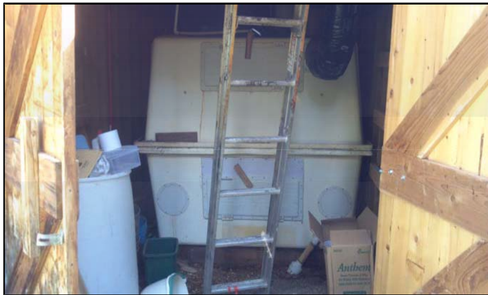
Figure 4. Photo of the full vault. Even the black vent pipe in photo right was full of human waste that did not decompose.
