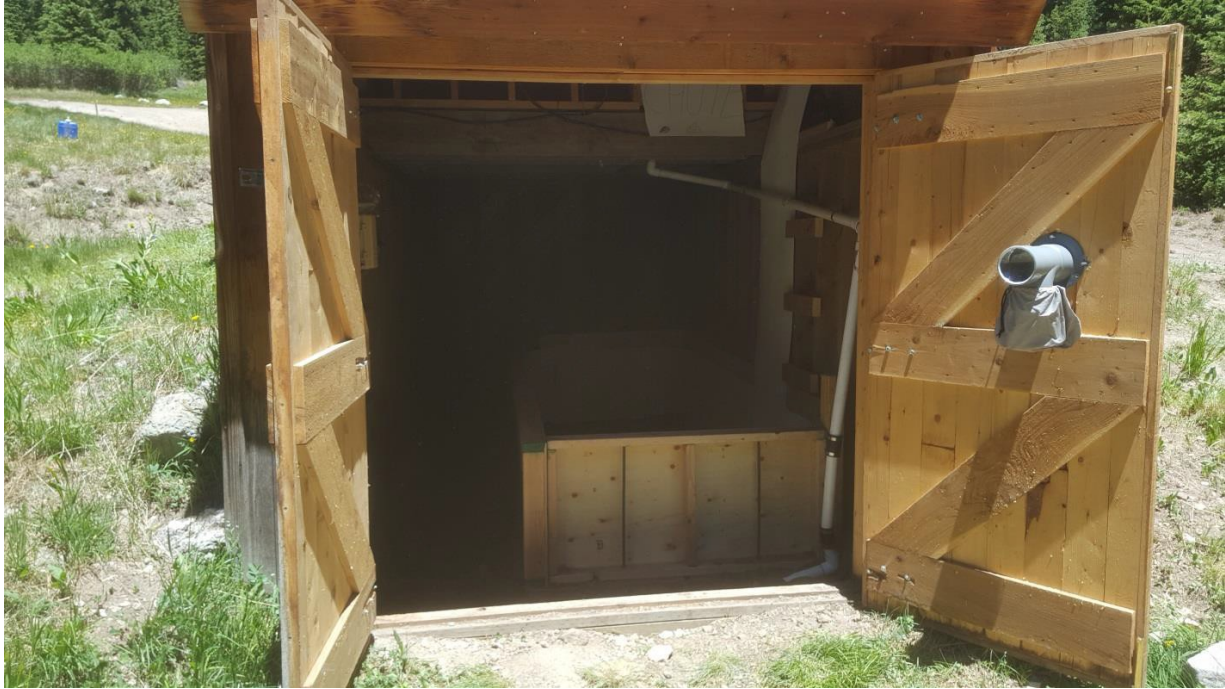
Figure 9. The completed Basement (visible area the waste crib, the urine drain line, and the fly trap.
