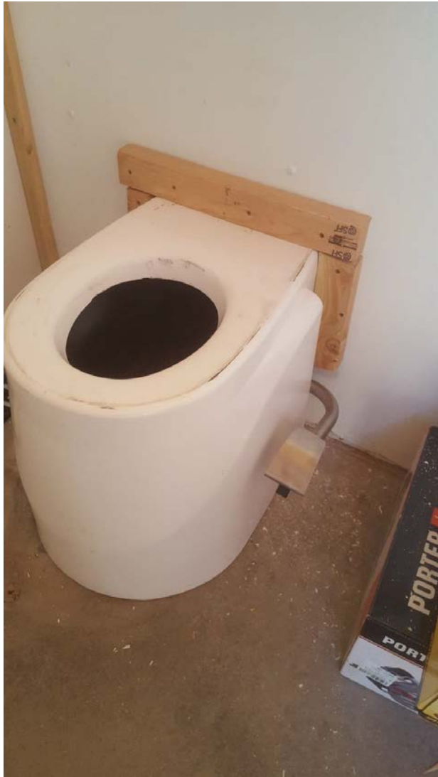
Figure 14. The toilet riser secured in place with wood trim.
