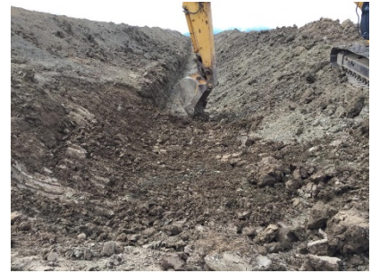
Figure 3 - Construction - Dam core
