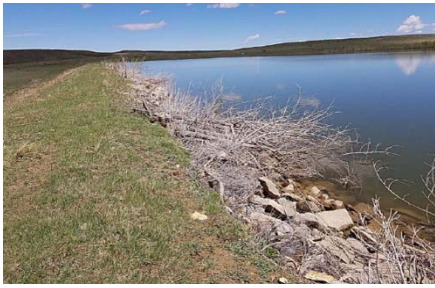
Figure 1 - Reservoir before construction
