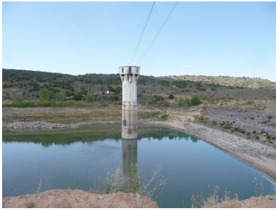
Figure 1 - Before construction - original outlet tower
