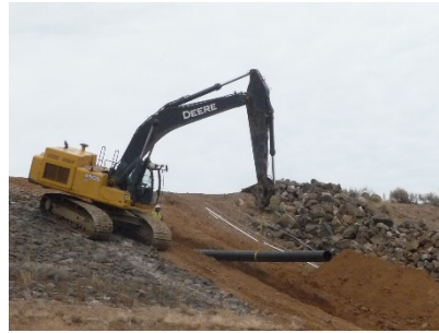
Figure 2 - New staff gage construction
