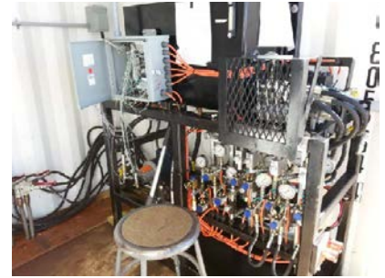
Figure 3 - After construction - new outlet controls
