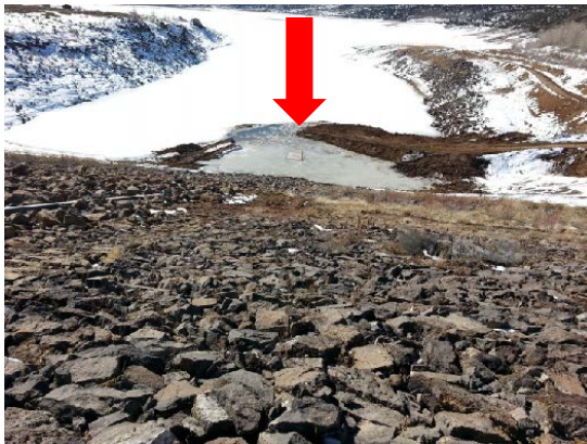
Figure 4 - After construction - new intake
