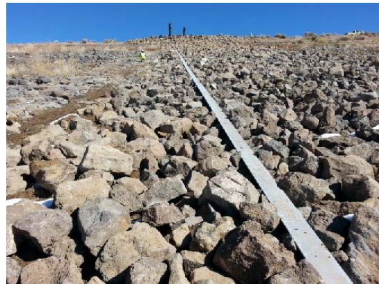
Figure 5 - After construction - new staff gage
