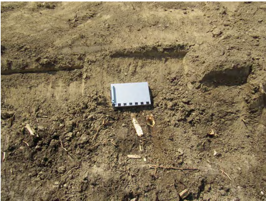
Photo 02 (08-22-2017) Roots in embankment by primary spillway (1)
