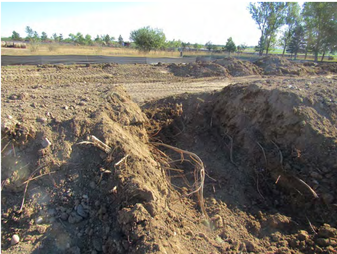
Photo 04 (08-25-2017) Roots in north dam embankment
