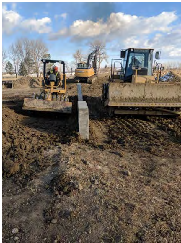
Photo 14 (12-14-2017) Spillway grade control beam backfill
