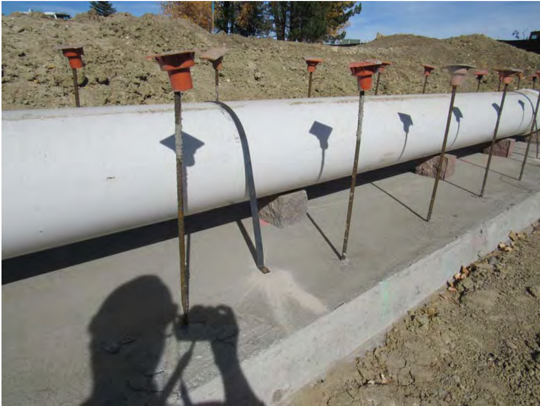
Photo 09 (10-24-2017) Irrigation PIP anchored to base of encasement
