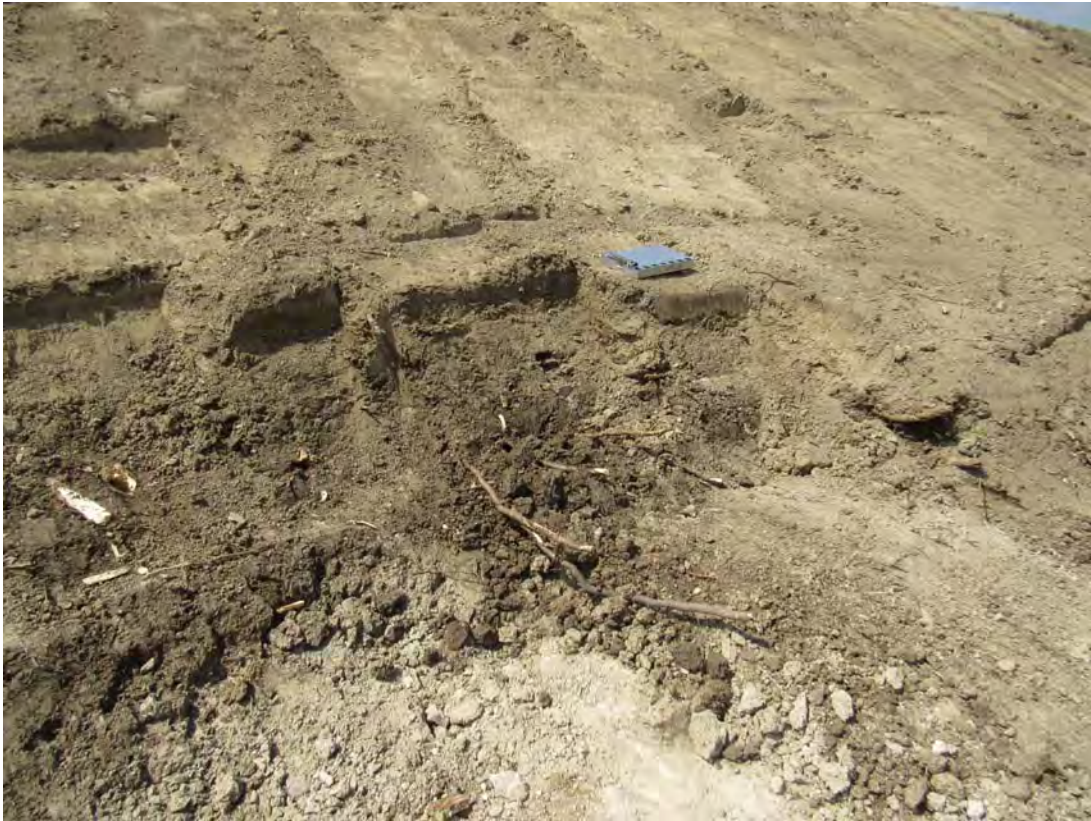
Photo 03 (08-22-2017) Roots in embankment by primary spillway (2)
