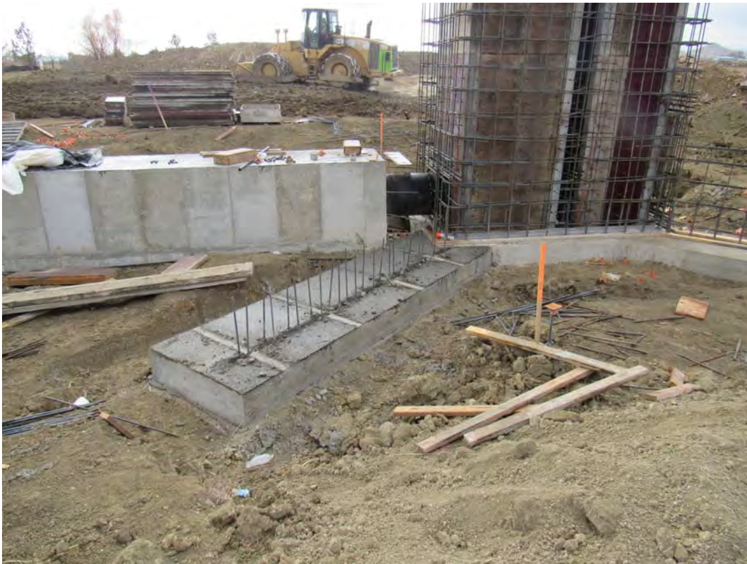
Photo 13 (11-21-2017) Northeast wingwall foundation after form removal
