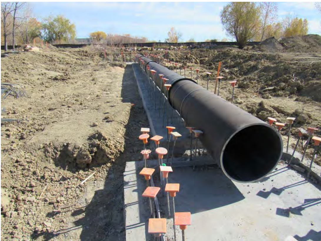
Photo 10 (10-24-2017) Primary outlet DIP anchored to base of encasement
