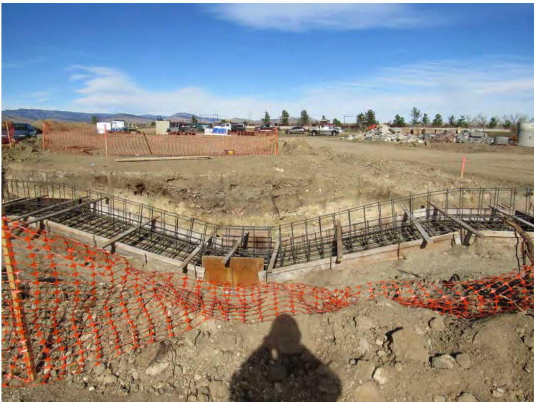
Photo 12 (11-20-2017) Spillway grade beam reinforcement
