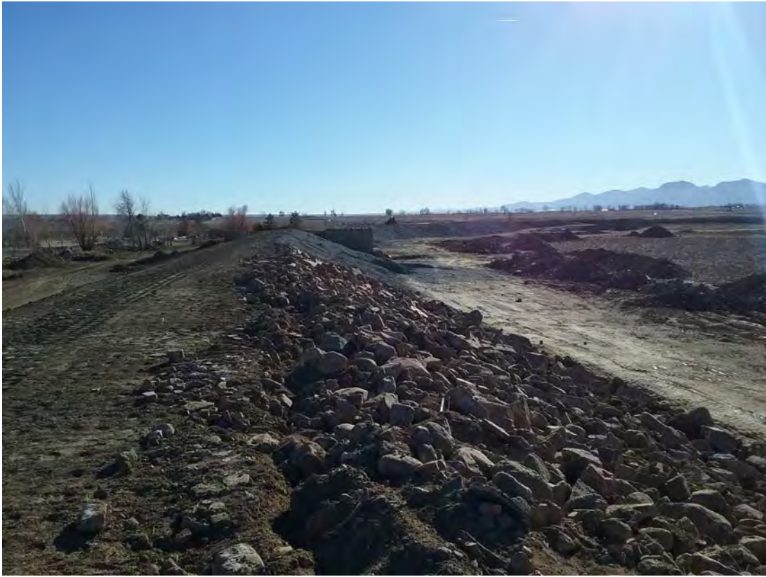
Photo 15 (01-02-2018) Bedding and riprap on upstream face
