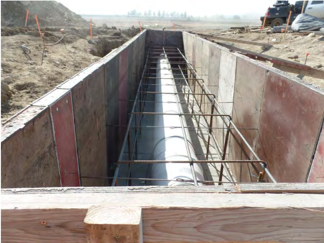
Photo 11 (11-03-2017) Irrigation outlet ecasement rebar and formwork
