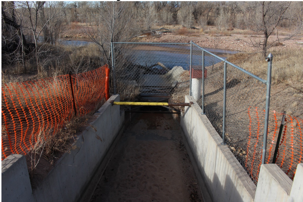
Chilcott Ditch Augmentation Station & Parshall Flume
