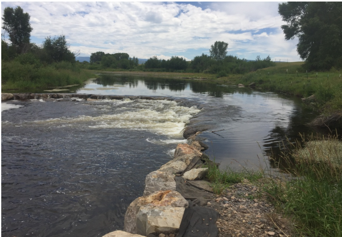
Figure 12. Diversion structure on Chuck Lewis SWA.
