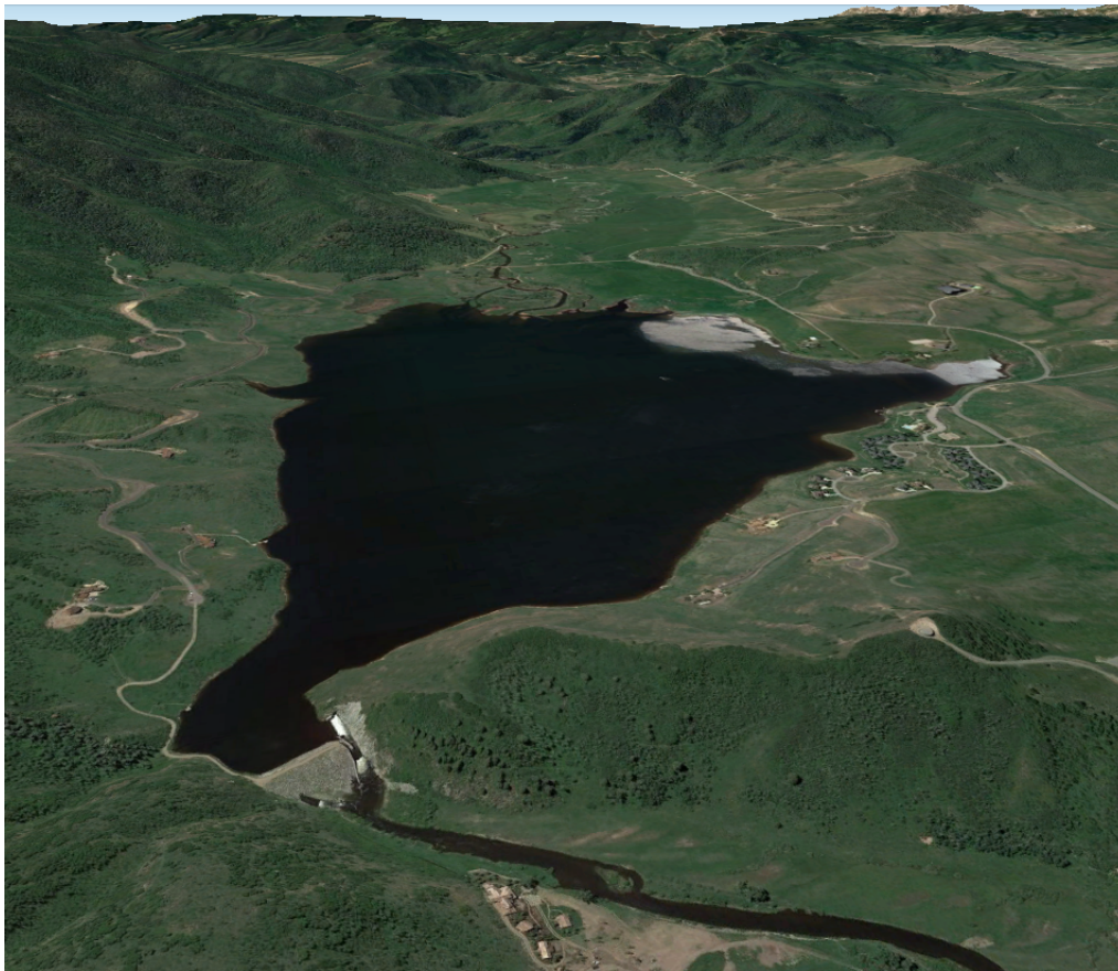
Figure 2: In-line dam and reservoir on the Yampa River at Lake Catamount.
