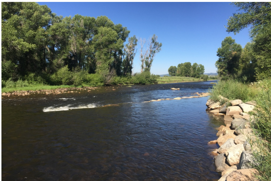
Figure 14. Diversion structure Below Town
