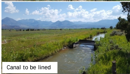
Canal to be piped
