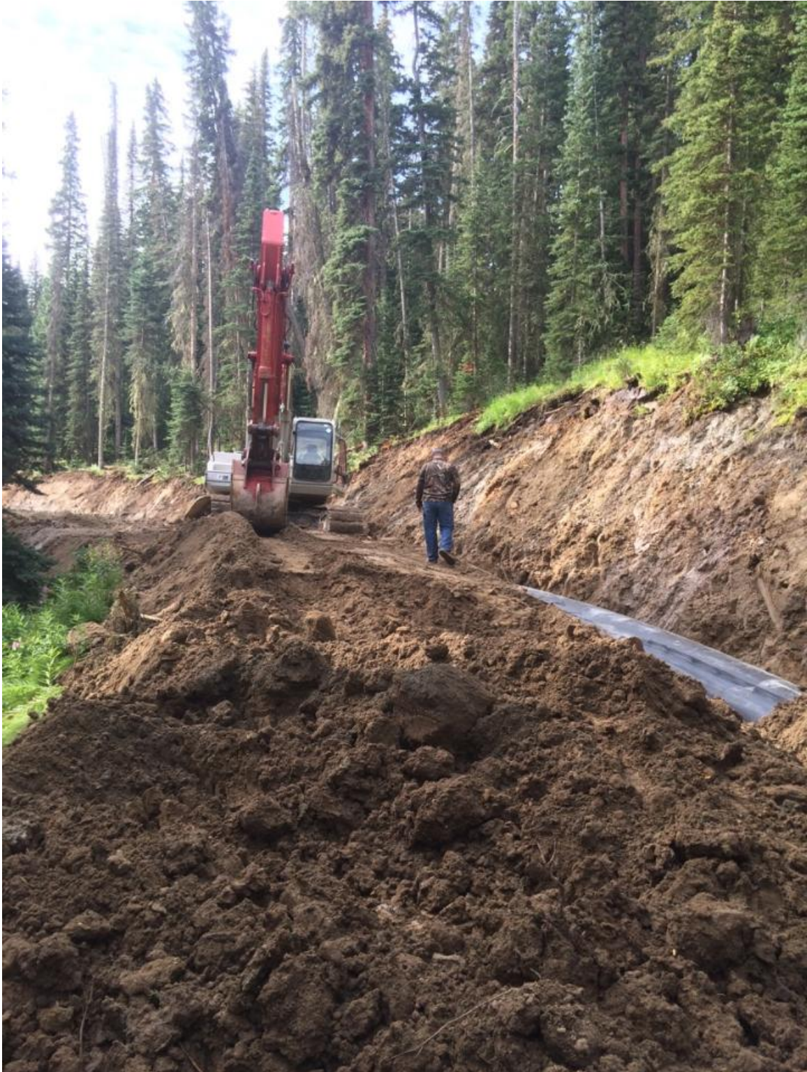
Pipe installed in ditch and backfill process being done
