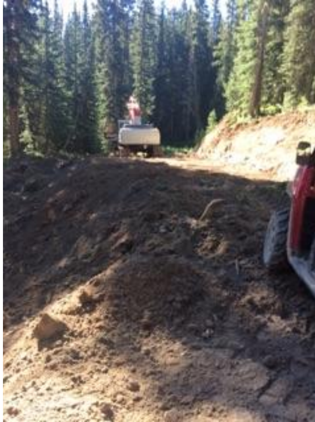
Pipe installed in ditch and covered
