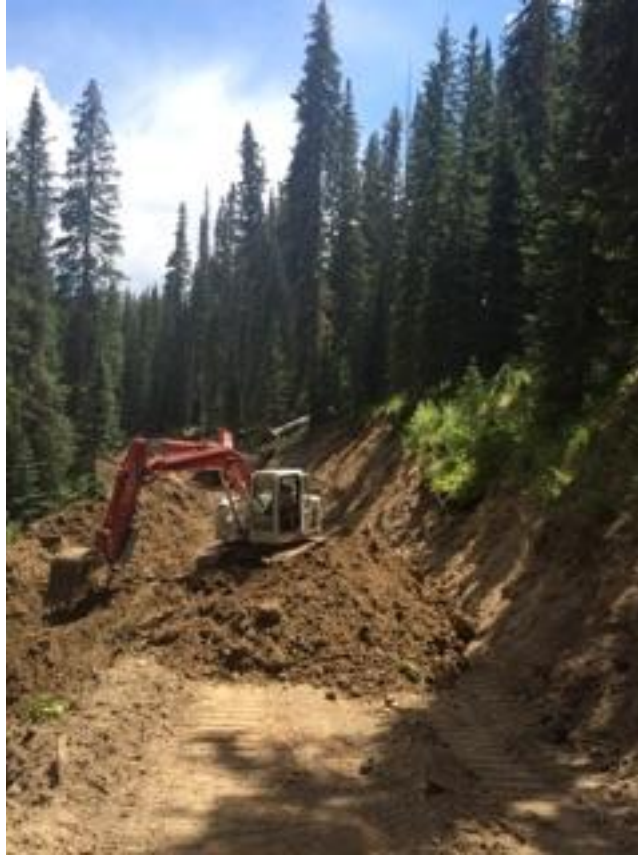
Finishing backfill process
