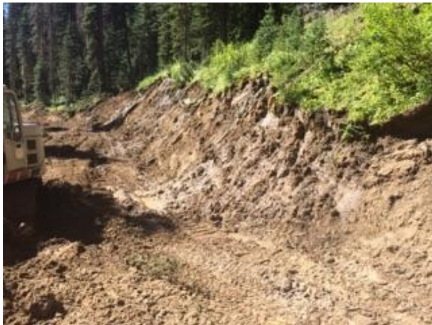
Pipe installed and backfill completed
