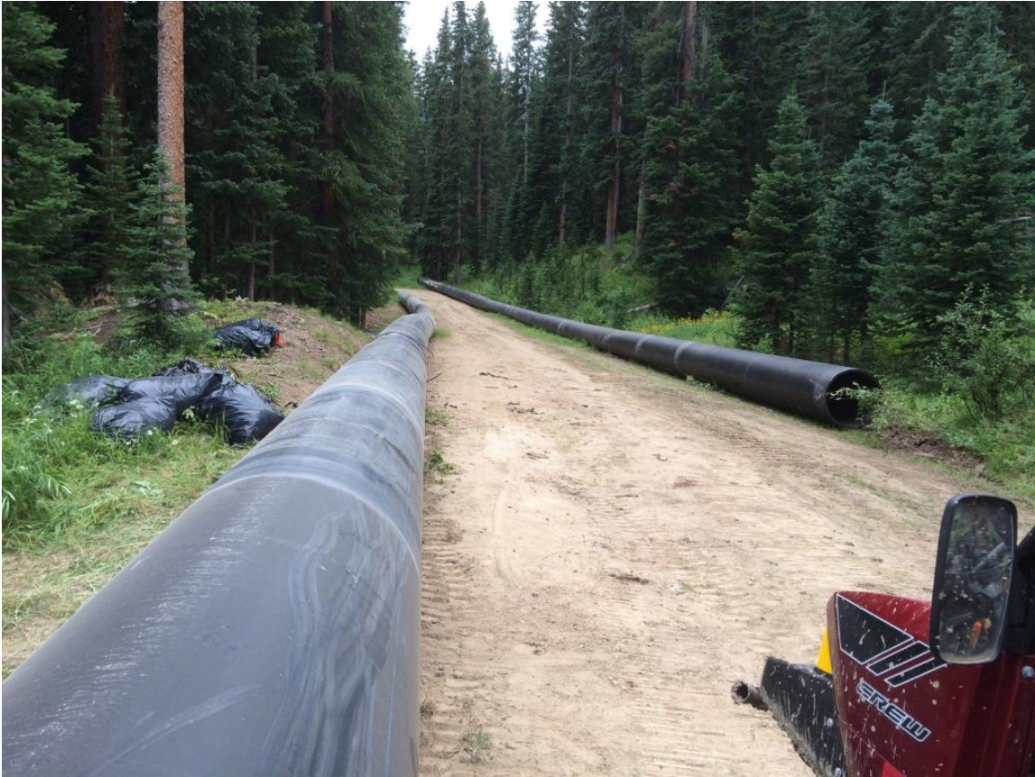
36" pipe on road above slide area welded & waiting to be transported to ditch.
