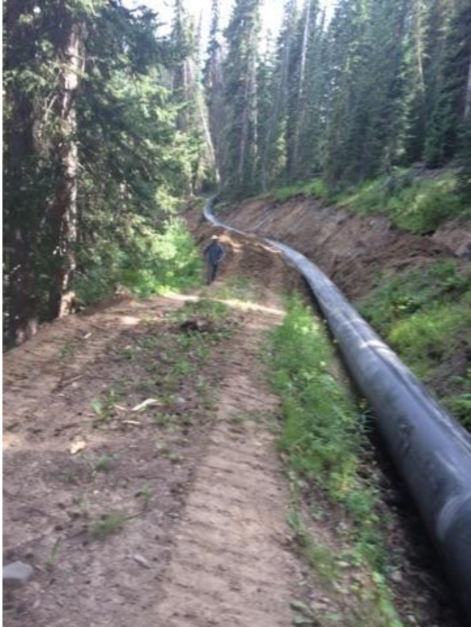
Pipe laid in ditch prepared for backfill
