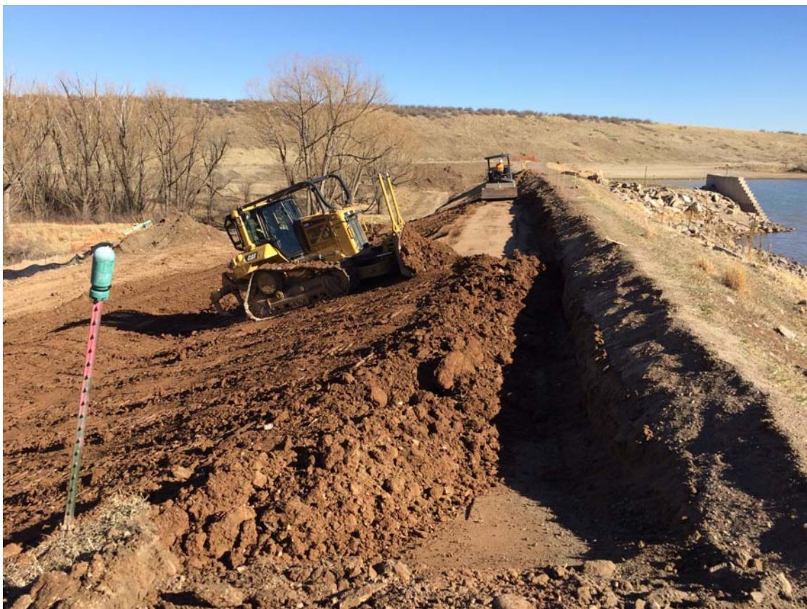
Completing the Chimney Drain Blanket
